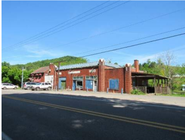
Photograph 8. Heaters District BX-0411
