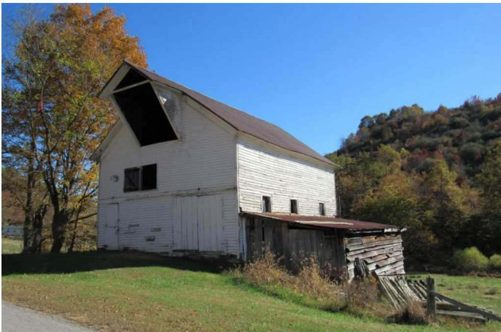
Photograph 5. RT-0744, frame barn with hay hood, facing southeast
