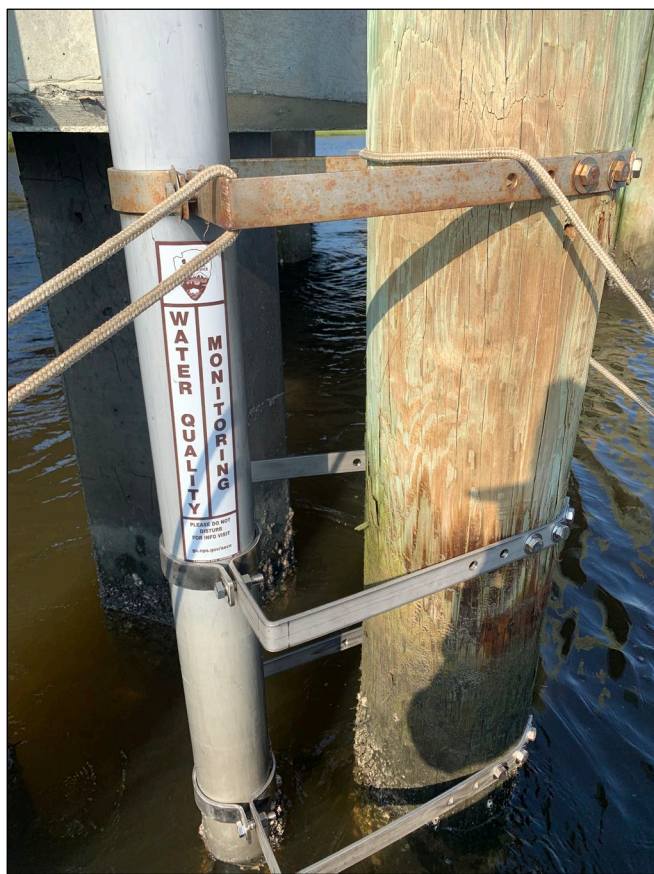
Figure 4. Stainless steel brackets affixing a 4-inch (10.16 cm) schedule 80 PVC sonde housing to a piling at site TIMUking01.
