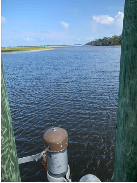
Figure 8. Locking end cap with bolt installed.
