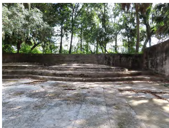
FIGURE 48. Overall view of the gun mounts and parapet wall.
