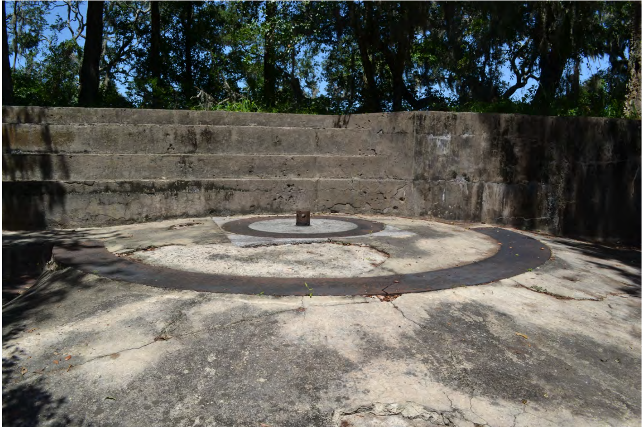
FIGURE 1. One of the gun emplacements associated with the Spanish-American War Battery overlooking the St. Johns River near Jacksonville, Florida, 2019. (Source: all photographs by the authors unless otherwise noted)
