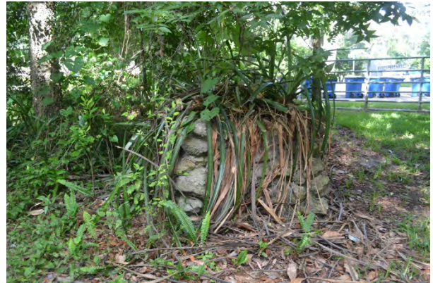
FIGURE 70. One of the two masonry columns located near the property boundary along Fort Caroline Road.
