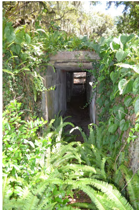
FIGURE 40. View northeast of the tunnel leading to the Spanish-American War Battery from the adjacent residential property.
