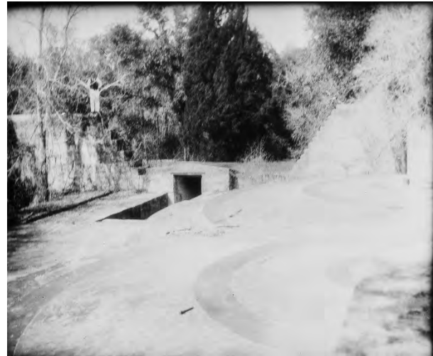
FIGURE 22. Spanish-American War Battery, St. Johns Bluff in 1934. (Source: HABS FL-15-2)
