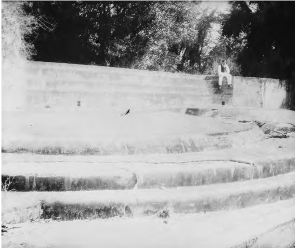
FIGURE 79. View northwest toward the battery showing the wooded nature of the top of the bluff beyond, 1934. (Source: HABS)
