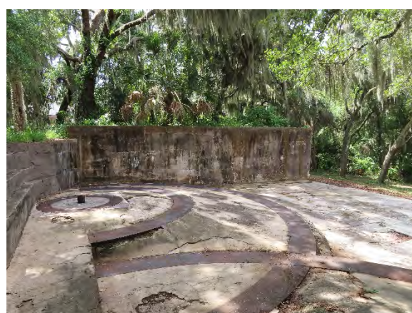
FIGURE 51. A view to the southeast of the traverse wall and a gun platform.
