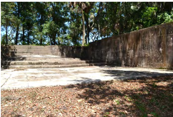
FIGURE 43. The concrete gun emplacement platform of the Spanish-American War Battery is set below a concrete retaining wall set into the slope near the top of the bluff.
