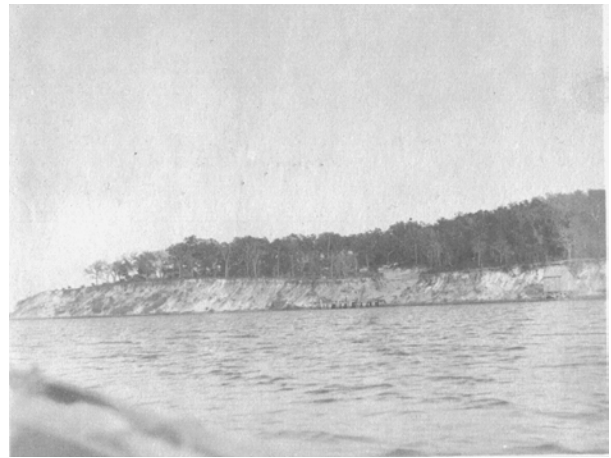
FIGURE 77. Circa 1900 photograph of St. Johns Bluff from the St. Johns River. The photograph shows a dock and a cut in the bank of the river near the center of the image where a rail line was established to convey construction materials to the top of the bluff for construction of the Spanish-American War Battery. To the right is a possible mine field terminal to the right. (Source: State Library & Archives of Florida) 337
