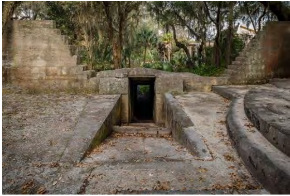
FIGURE 45. The Spanish-American War Battery contains a concrete gun emplacement platform and a concrete magazine. A concrete tunnel links the two features and continues to a western arched opening.
