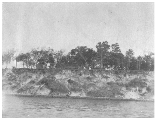
FIGURE 78. Circa 1900 photograph of St. Johns Bluff and the military reservation associated with the Spanish-American War Battery from the river. Buildings erected to support the project are visible, along with riprap placed along the river shoreline to protect against erosion. (Source: State Library & Archives of Florida) 338
