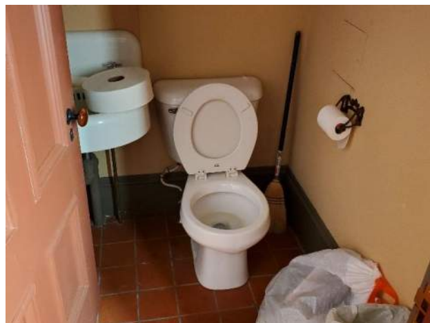
Figure 3.68: First floor toilet room.
