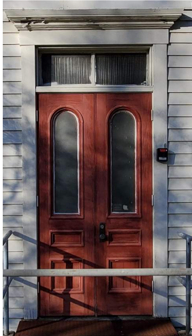
Figure 3.29: South, Back Door - Elevation.
