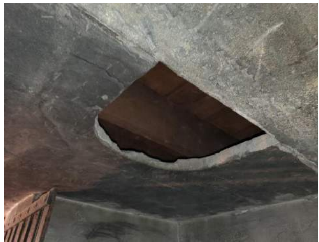
Figure 3.81: Broken bluestone.
