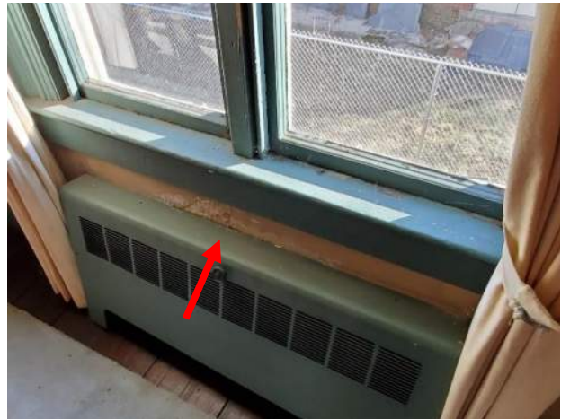
Figure 3.57: Moisture damage.
