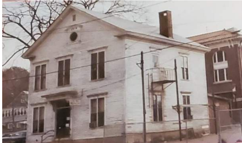
Figure 2.5: Mid-century photo shows Town Hall in need of some repair, but by now front steps were already replaced and a fire access provided from the second floor. Courtesy of the Town of North Providence.
