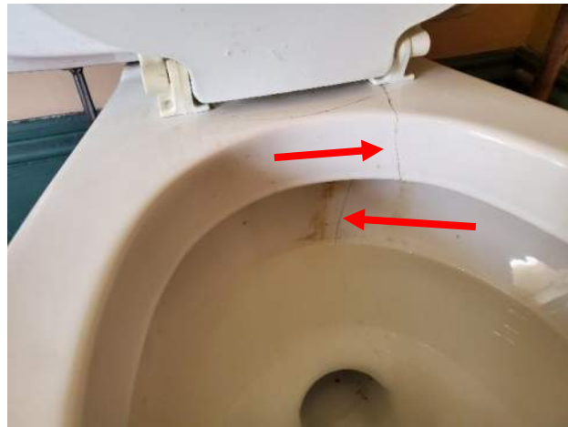
Figure 3.60: Cracked toilet.
