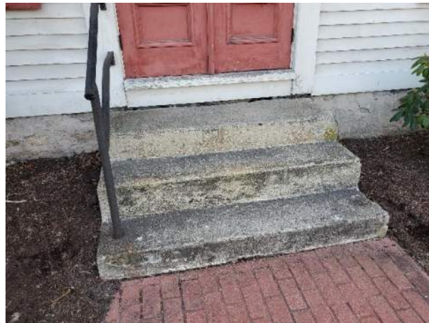
Figure 3.4: Concrete steps to north entrance.
