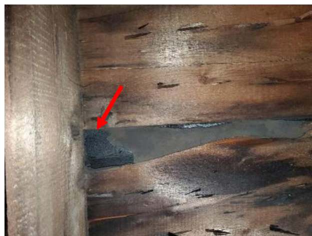
Figure 3.51: Visible backside of shingles.
