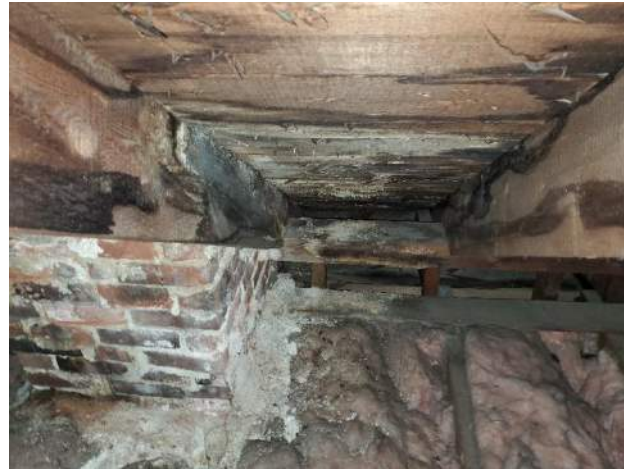
Figure 3.52: Roof deck at chimney.
