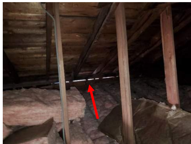
Figure 3.54: East roof edge.
