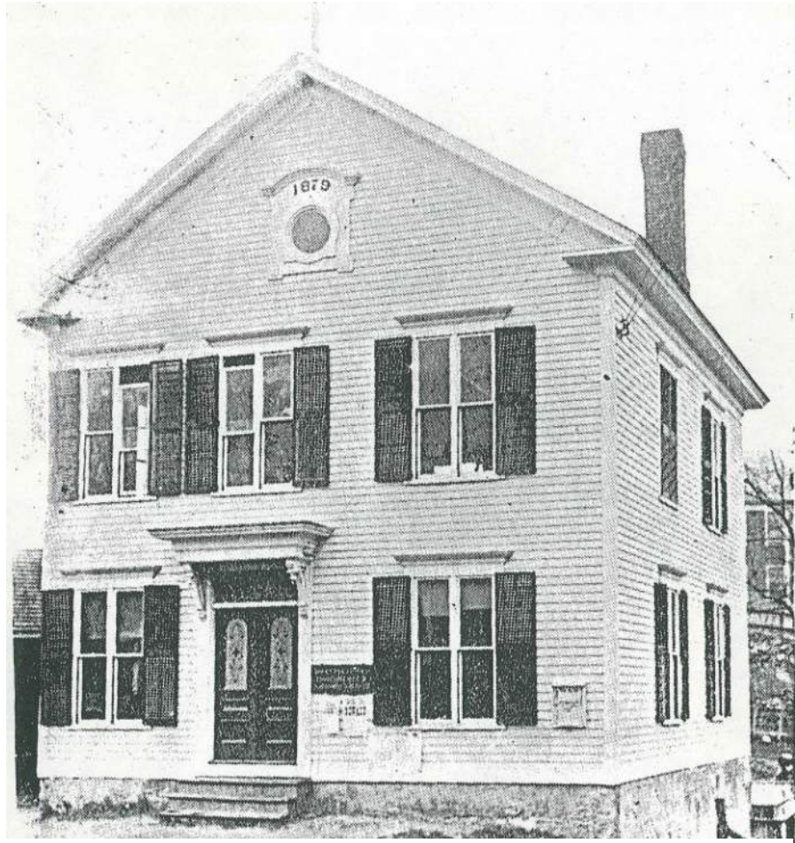
Figure 2.2: Significant details are noted in this older photo of Town Hall: An older version of the chimney, the original second-floor window at the northwest corner, the coal chute, the front wooden steps, window shutters, and a structure standing seemingly close to the east wall. Courtesy of the Town of North Providence. Undated.
