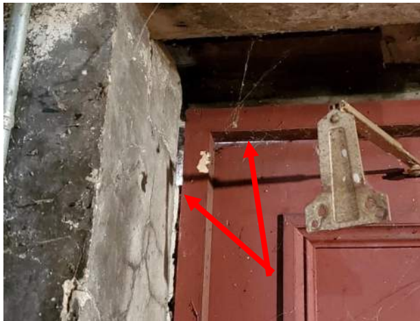
Figure 3.38: Basement Door - Daylight.
