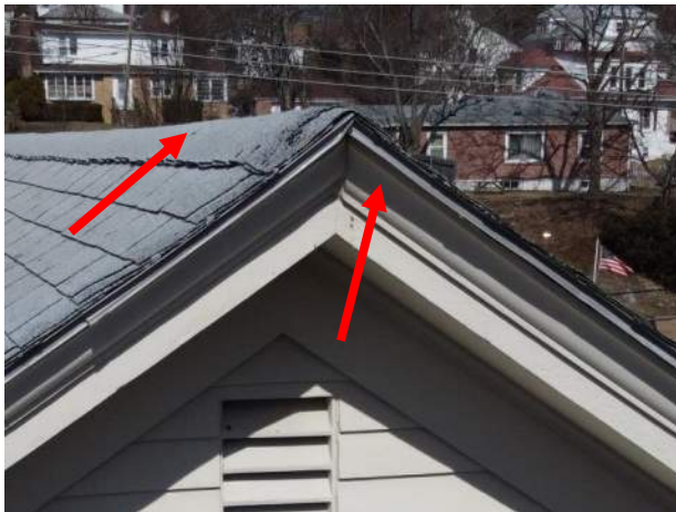
Figure 3.14: Ridge is straight, Metal edge at rake.
