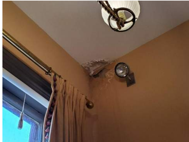
Figure 3.59: Roof Leak.
