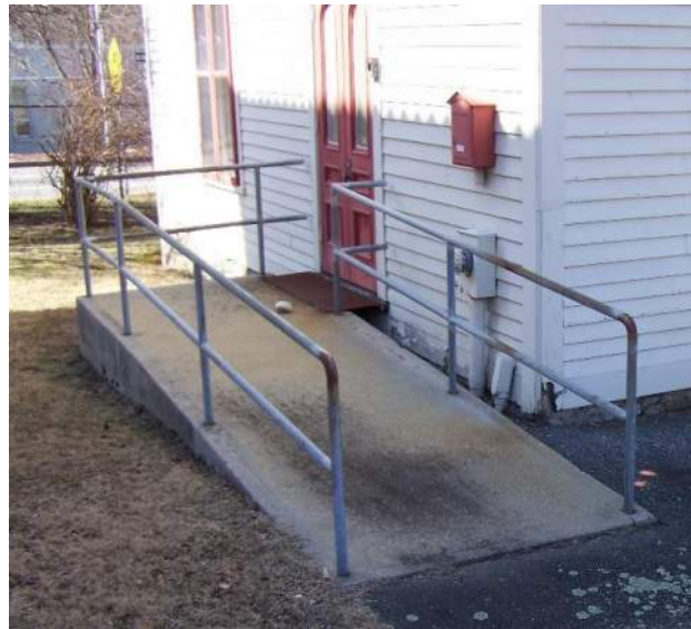
Figure 3.3: Concrete ramp to south entrance.
