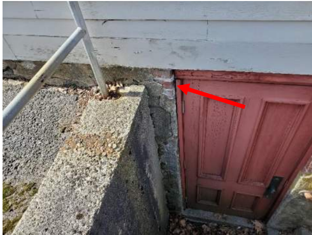
Figure 3.36: Basement Door – exposed brick.
