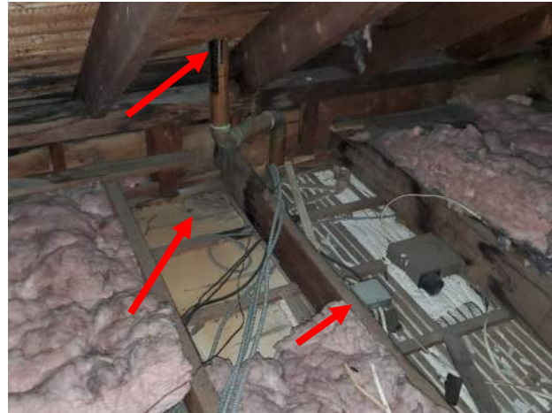
Figure 3.53: Plumbing vent.
