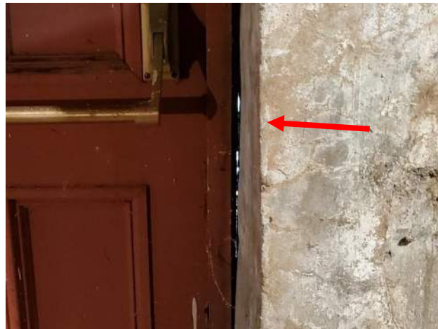
Figure 3.39: Basement Door - Daylight.
