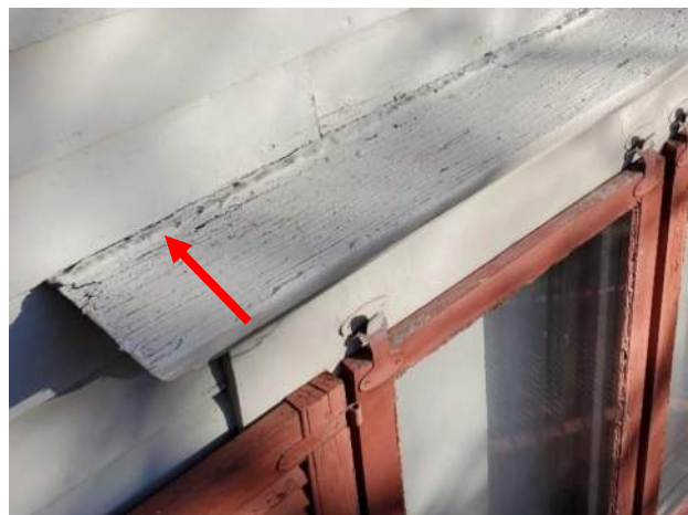
Figure 3.22: Window drip cap.
