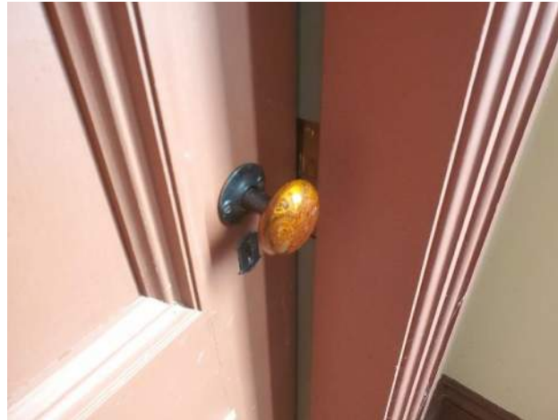
Figure 3.66: Door 1-8 doesn't latch.
