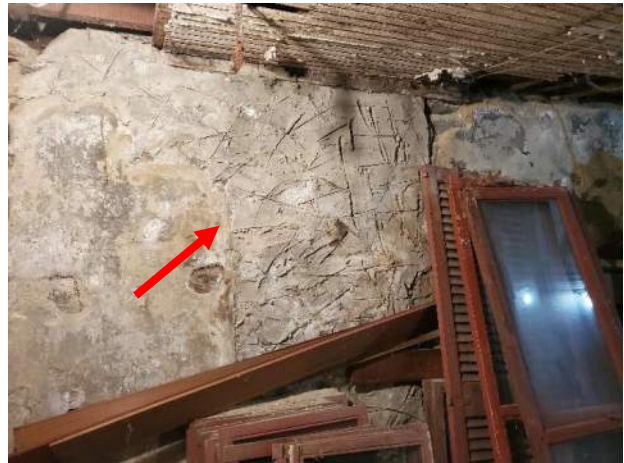
Figure 3.46: Infilled opening.
