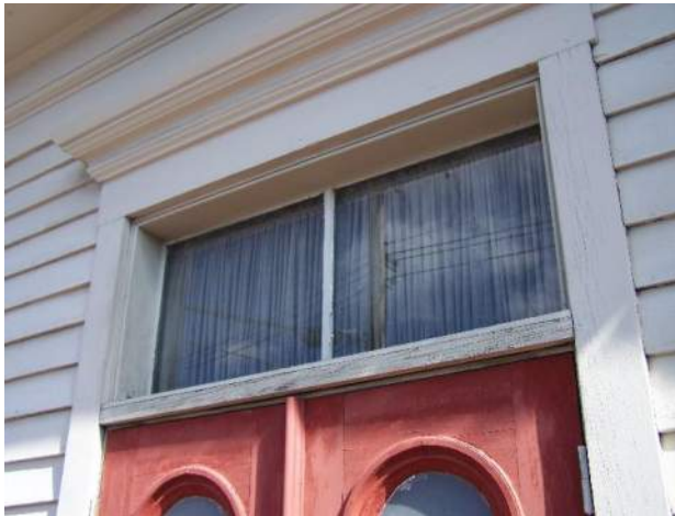
Figure 3.32: Second Floor Egress Door - Transom.
