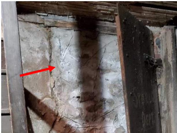
Figure 3.47: Infilled opening.
