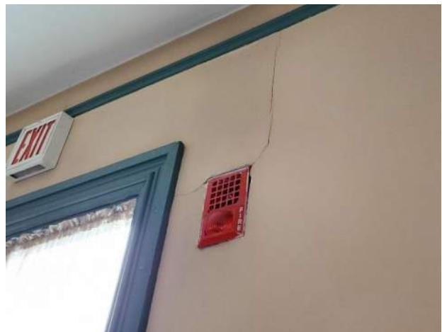
Figure 3.58: Plaster crack.
