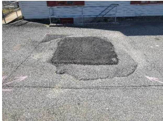
Figure 3.9: Recent work on Parking lot.
