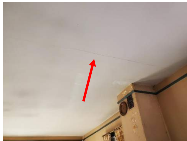
Figure 3.64: Ceiling crack.
