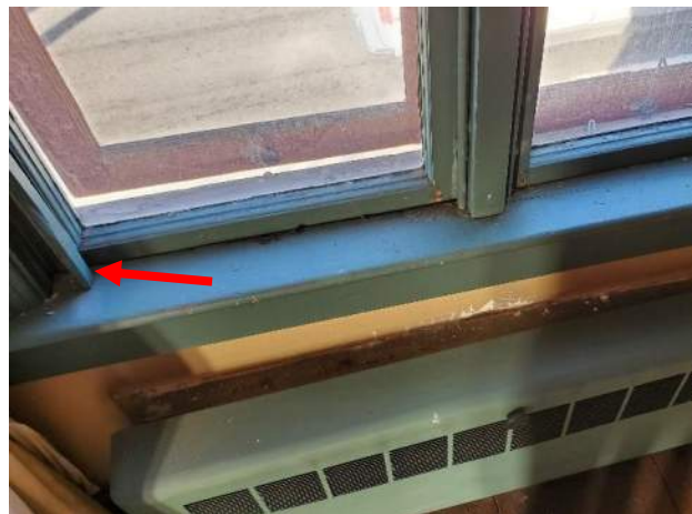
Figure 3.24: Window interior - stool.
