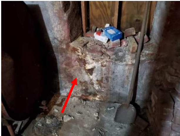
Figure 3.45: Interior Coal Chute.
