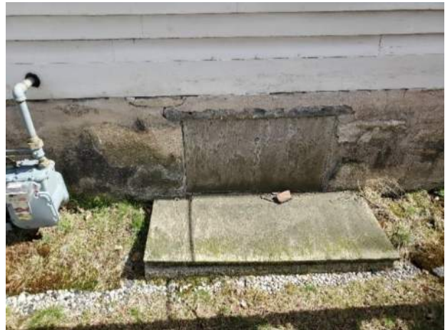
Figure 3.41: Coal Chute.
