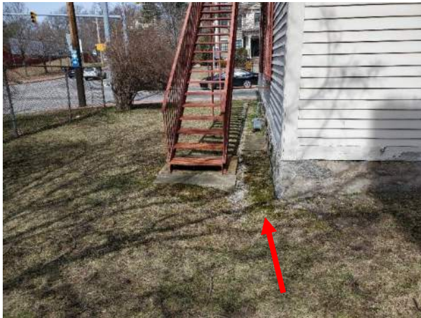
Figure 3.8: Ponding along dripline.
