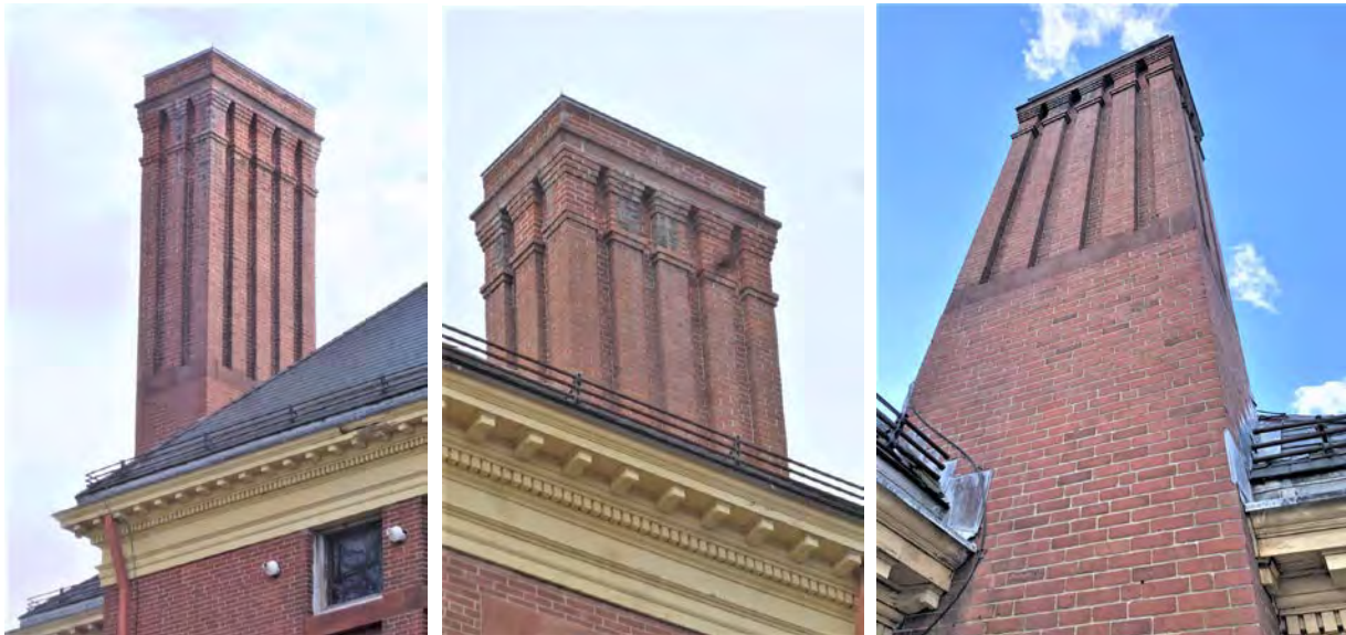
Cumberland Town Hall – Exterior - Masonry Chimney at Northeast Corner – Left: North and East Elevations; Center: South and East Elevations; Right: East Elevation In Good Condition
