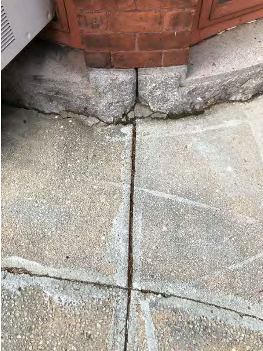
Cumberland Town Hall – Exterior – Landscaping Elements South Elevation – Concrete Pavement adjacent to Building Open Joint in Granite at Base of Building and in Concrete Pavement
