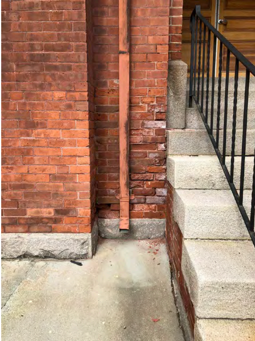
Cumberland Town Hall – Roofing, Flashing, Gutters, Leaders, Metal Trim and Roofing Elements South Elevation
