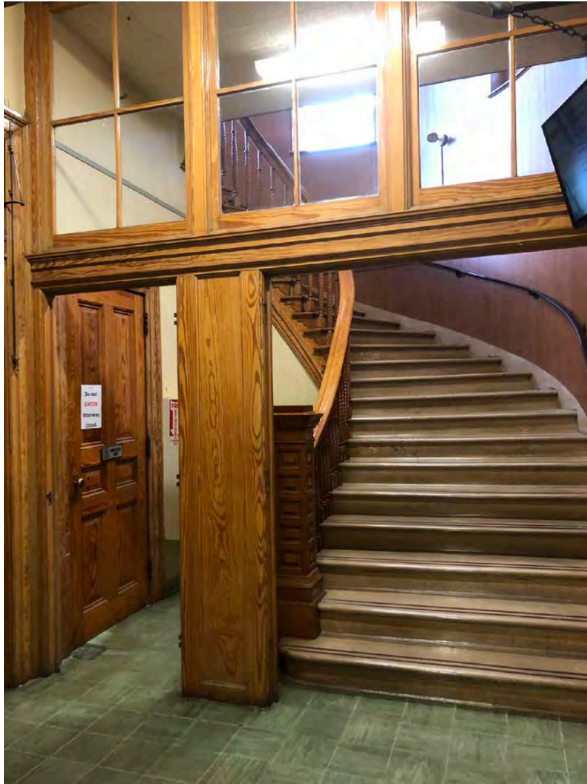
Cumberland Town Hall – Interior – Historic Finishes and Building Elements
