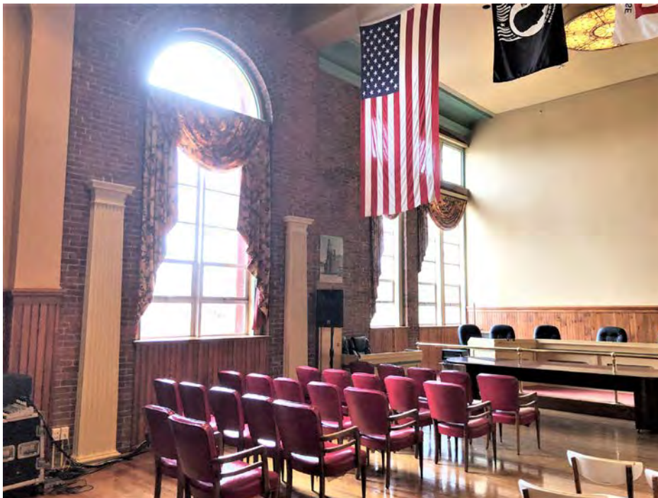
Cumberland Town Hall – Interior – Masonry - Historic Finishes and Building Elements Second Floor – Council Chamber Looking Northeast Overall Condition Good
