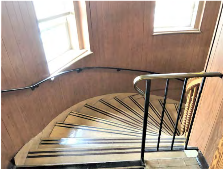
Cumberland Town Hall – Interior – Historic Finishes and Details Second Floor View of Main Stair Vinyl Applied to Treads, Veneer Paneling on Walls
