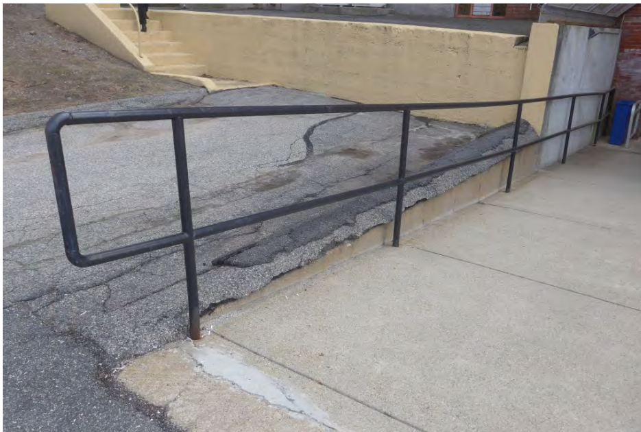
Cumberland Town Hall – Exterior – Retaining Walls, Steps, Landscaping, Asphalt Parking Area and Miscellaneous Landscaping Elements North Elevation
