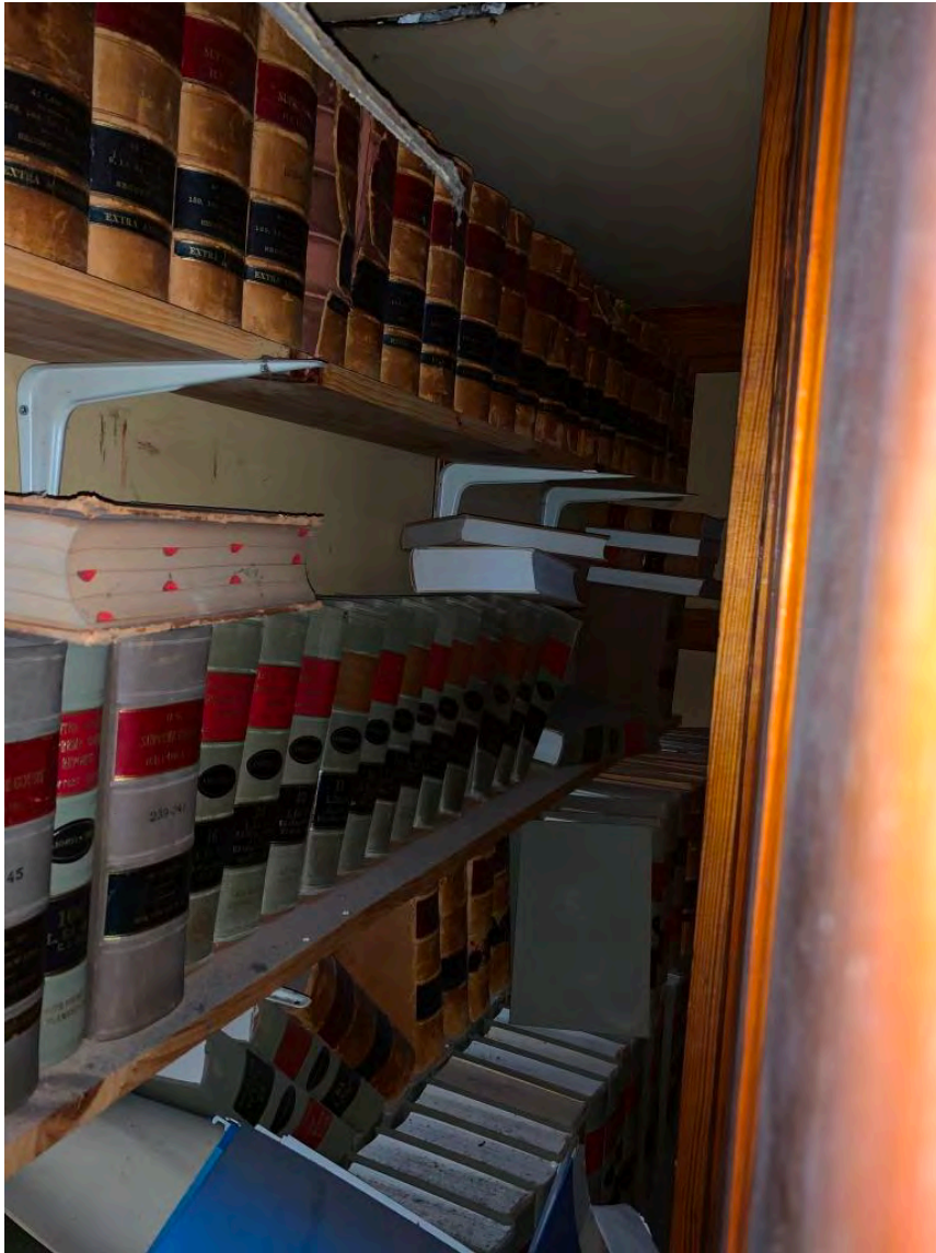
Cumberland Town Hall – Interior – Storage Third Floor – Stair Hall, Northwest Room Neglected Storage Area Behind Wall
