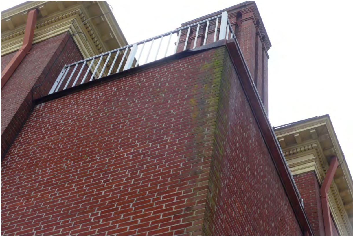
Cumberland Town Hall – Exterior - Masonry East Elevation at Northeast Corner Lifting Fascia at roof level
