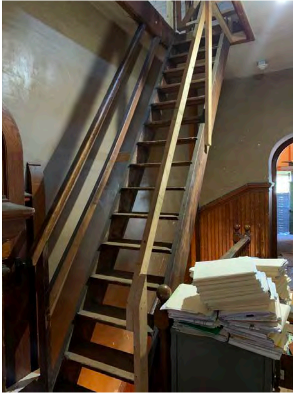
Cumberland Town Hall – Interior – Code Compliance Tower – Stairs Up to Tower Left: Steep Stairs; Right: No Handrail and Limited Access
