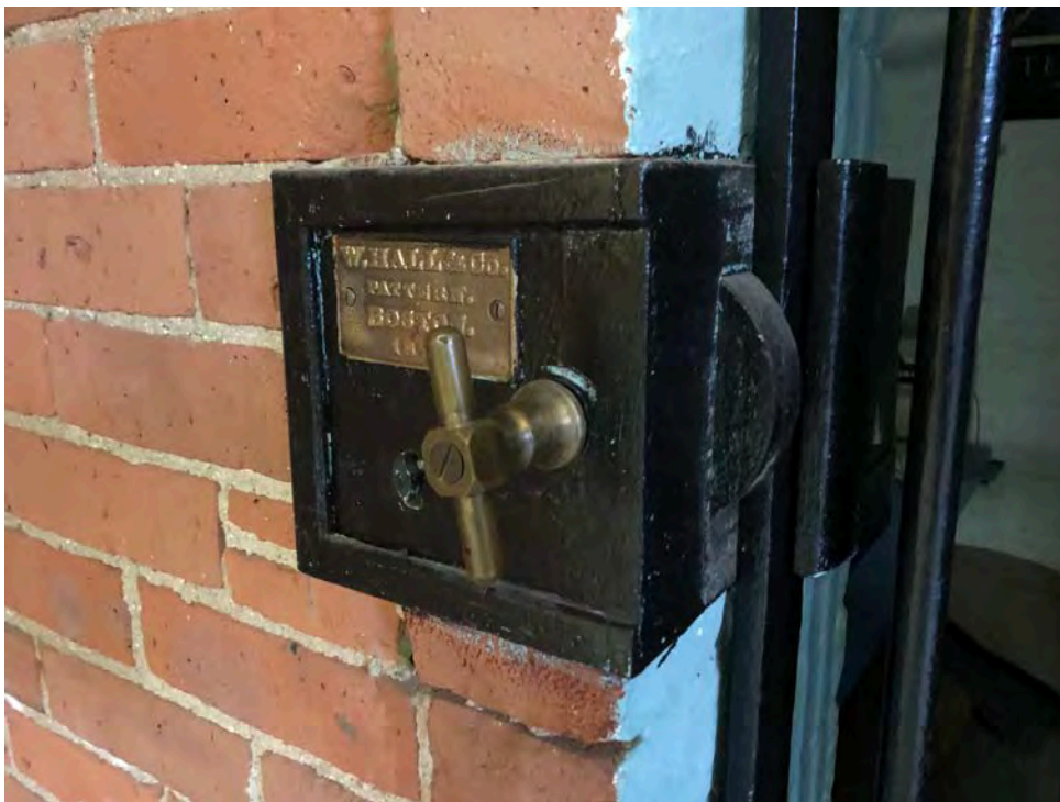
Cumberland Town Hall – Interior – Historic Finishes and Building Elements Basement – At Jail Cells – Original Hardware for Cell Doors Typical Conditions - Good
