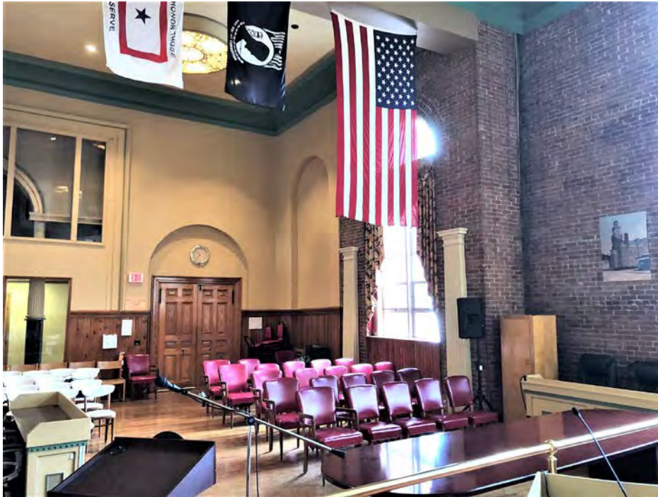
Cumberland Town Hall – Interior – Masonry – Historic Finishes and Building Elements Second Floor – Council Chamber Looking Northwest Overall Condition Good; Exposed Brick not Historically Appropriate
