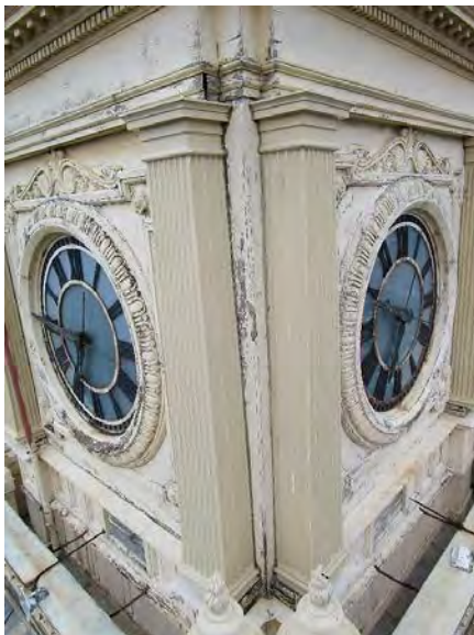
Cumberland Town Hall – Exterior – Wood Elements Tower – Clock Level (Sixth Floor) Flaking and Deteriorated Paint – Some Deteriorated Wood Source: Town of Cumberland
