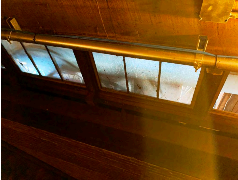
Cumberland Town Hall – Interior – Historic Finishes and Elements Tower – Windows Between Tower and Attic Over Assembly Hall
