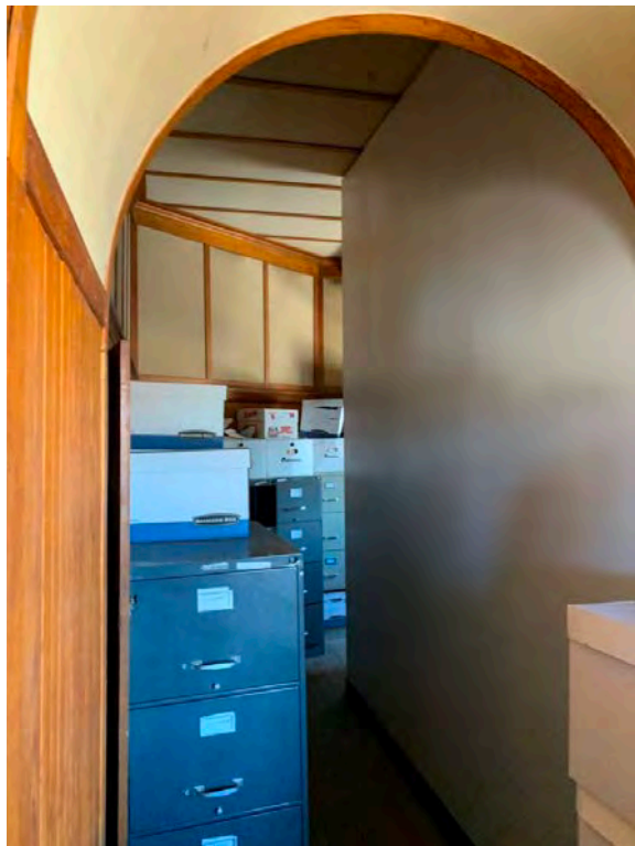
Cumberland Town Hall – Interior – Historic Finishes and Elements - Storage Third Floor – Stair Hall, Northwest Room and Curved Room over Main Stair 1930s-era Paneled Walls and Ceiling in Good Condition; Tech Closet Inserted in Northwest Room Excessive Storage Creating Substantial Load
