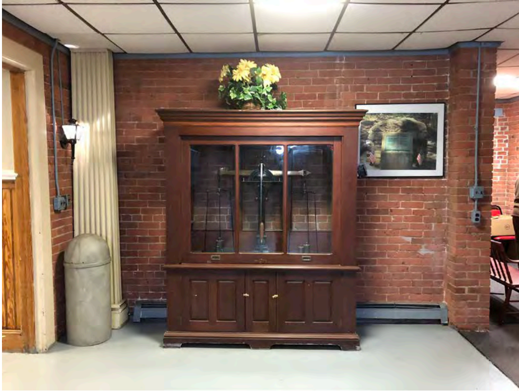
Cumberland Town Hall – Interior – Historic Finishes and Building Elements Basement – Basement Entrance Weights and Measures Cabinet
