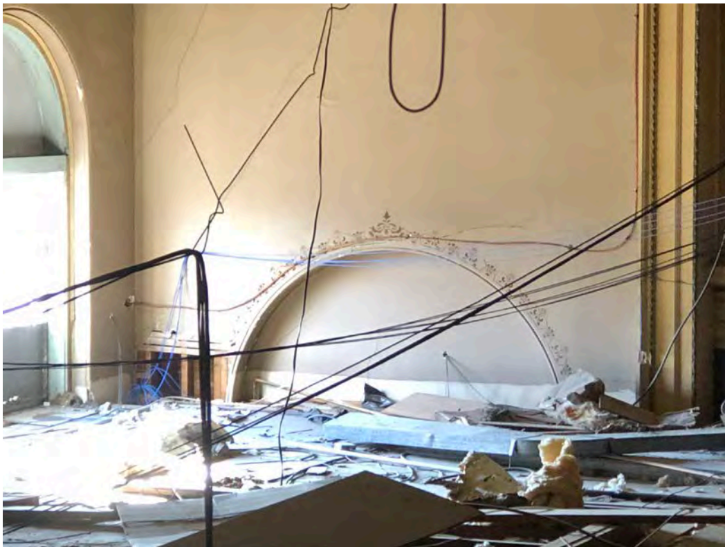
Cumberland Town Hall – Interior - Historic Finishes and Details – Plaster Walls and Ceilings Third Floor – Original Upper Assembly Hall Note: Original Stenciled Detail at Side Arch
