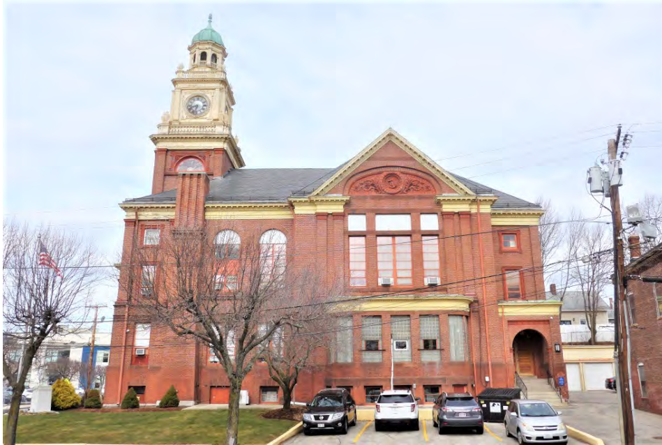
Cumberland Town Hall – Exterior Overalls South Elevation – Overall
