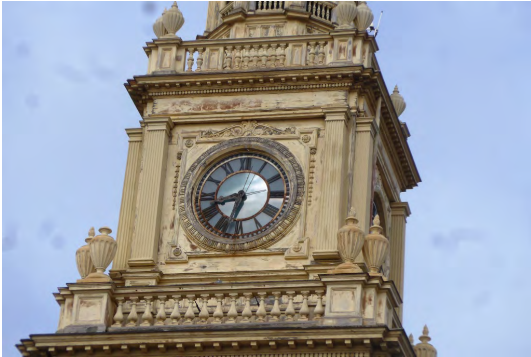
Cumberland Town Hall – Exterior – Wood Elements Tower – Clock Level (Sixth Floor) Overall View - Flaking and Deteriorated Paint – Some Deteriorated Wood
