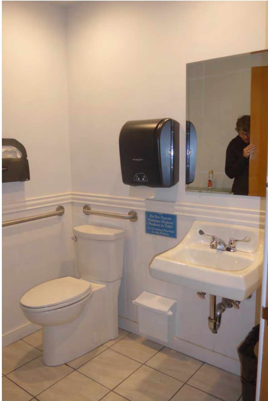
Cumberland Town Hall – Interior - Accessibility Conditions Unisex ADA Compliant Toilet Room
