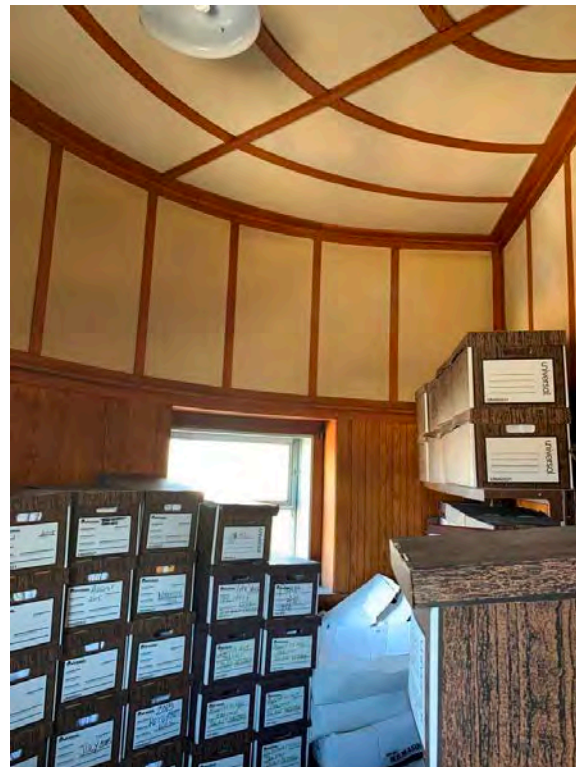
Cumberland Town Hall – Interior – Historic Finishes and Elements - Storage Third Floor – Stair Hall, Northwest Room and Curved Room over Main Stair 1930s-era Paneled Walls and Ceiling in Good Condition; Tech Closet Inserted in Northwest Room Excessive Storage Creating Substantial Load
