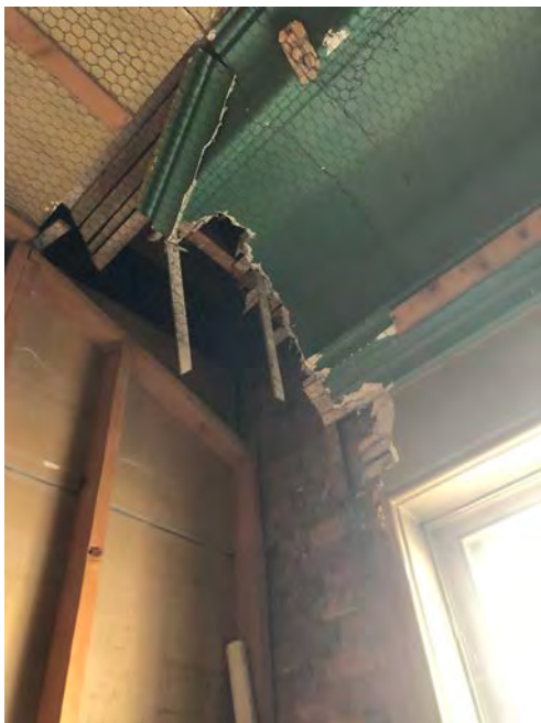
Cumberland Town Hall – Interior - Historic Finishes and Details – Plaster Walls and Ceilings Third Floor – Original Upper Assembly Hall Severe Unrepaired Damage to Plaster Walls, Ceiling, and Trim from Previous Leaks
