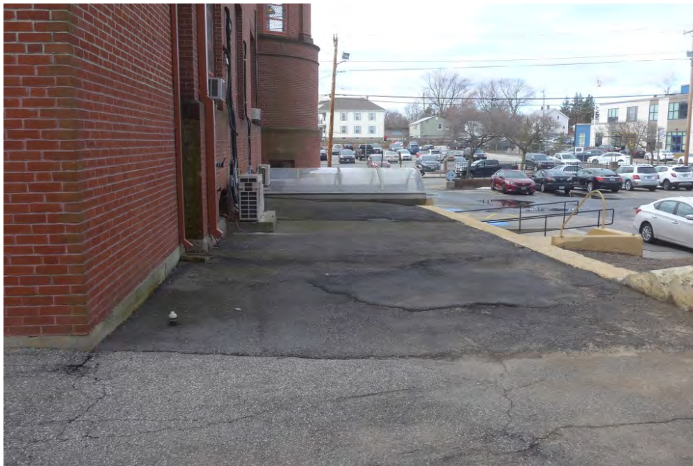
Cumberland Town Hall – Exterior – Retaining Walls, Steps, Landscaping, Asphalt Parking Area and Miscellaneous Landscaping Elements
