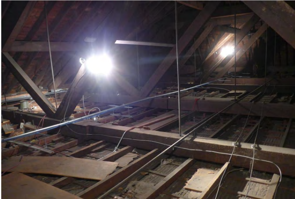
Cumberland Town Hall – Structure Attic – Looking East In Good Condition
