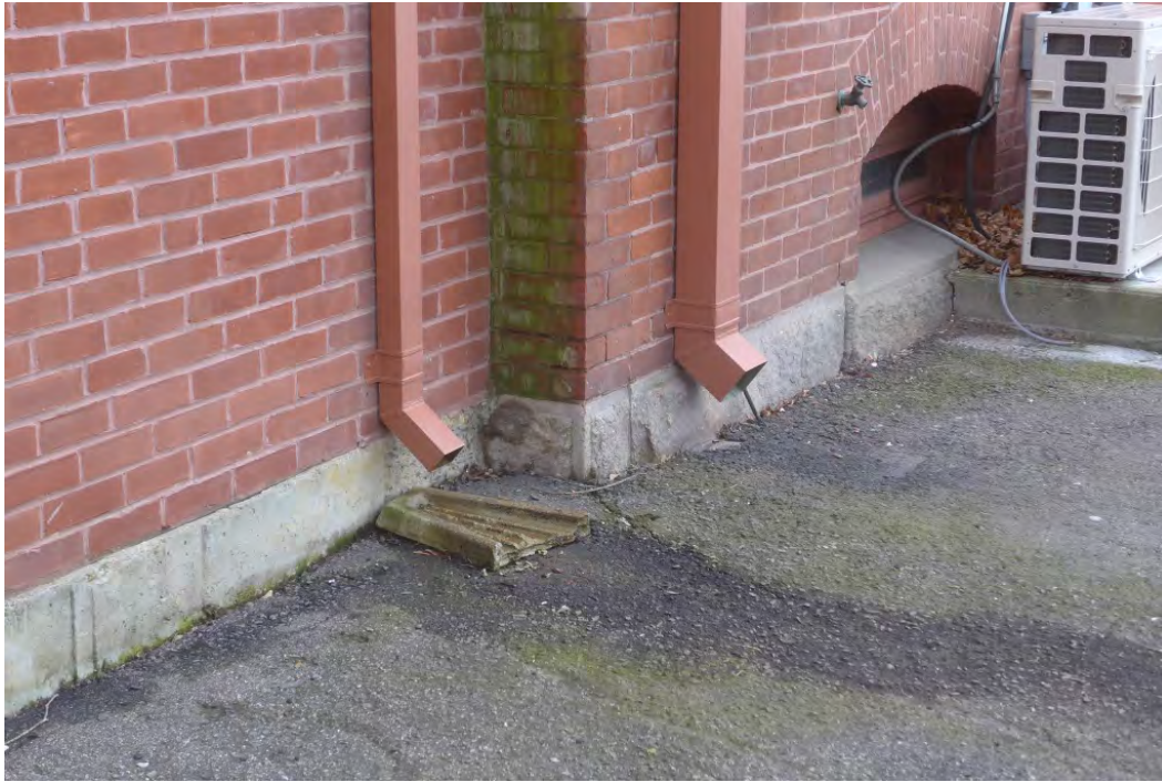
Cumberland Town Hall – Roofing, Flashing, Gutters, Leaders, Metal Trim and Roofing Elements
