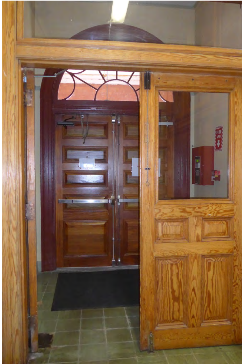
Cumberland Town Hall – Interior –Historic Finishes and Building Elements – Windows, Doors and Hardware
