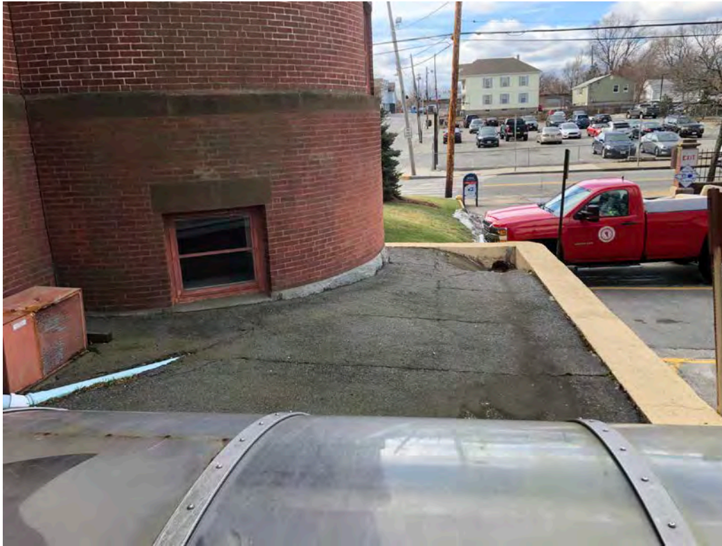
Cumberland Town Hall – Exterior – Retaining Walls, Steps, Landscaping, Asphalt Parking Area and Miscellaneous Landscaping Elements North Elevation
