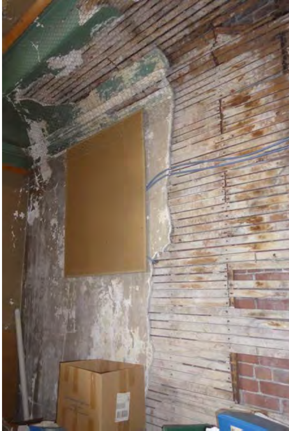
Cumberland Town Hall – Interior - Historic Finishes and Details – Plaster Walls and Ceilings Third Floor – Original Upper Assembly Hall Severe Unrepaired Damage to Plaster Walls, Ceiling, and Trim from Previous Leaks
