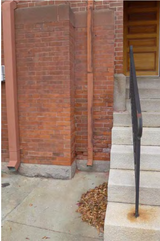
Cumberland Town Hall – Exterior – Masonry South and East Elevations - Southeast Corner – Entrance Open Joints, Deteriorated/Missing Brickwork; Staining
