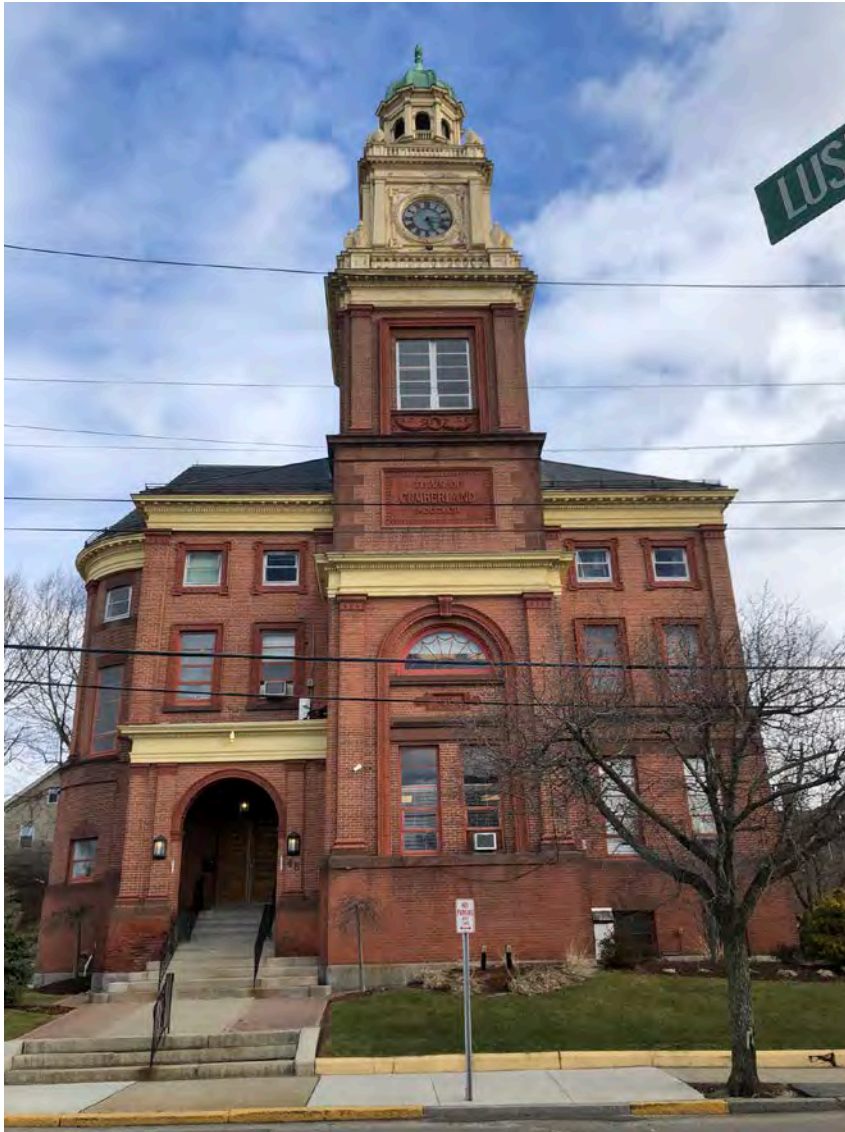
Cumberland Town Hall – Exterior Overalls West Elevation – Overall
