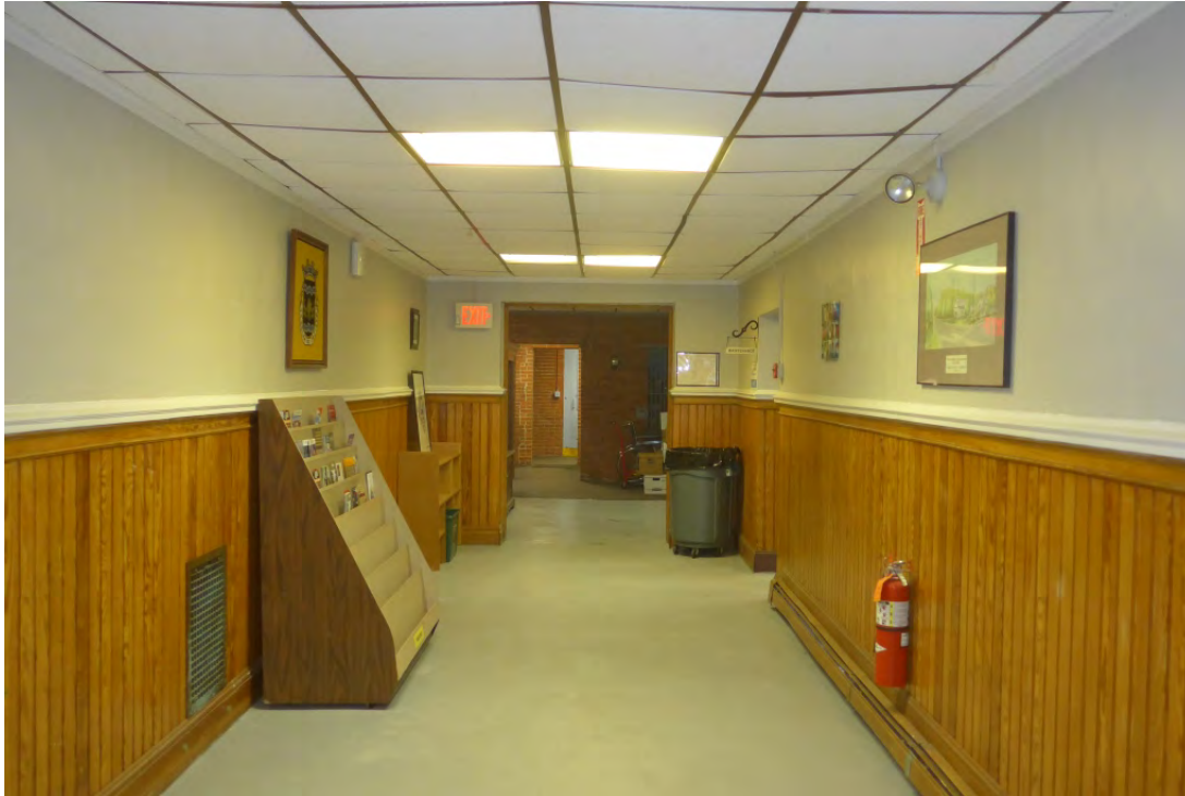
Cumberland Town Hall – Interior – Overall – Historic Finishes and Building Elements - Ceilings
