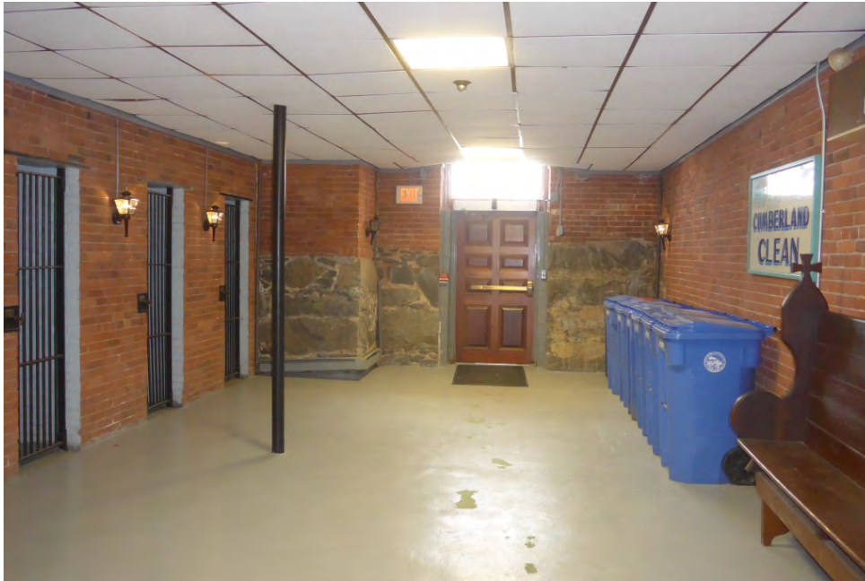
Cumberland Town Hall – Interior - Overall and Masonry Basement – Entrance Looking Toward Handicap Access Typical Conditions – Good
