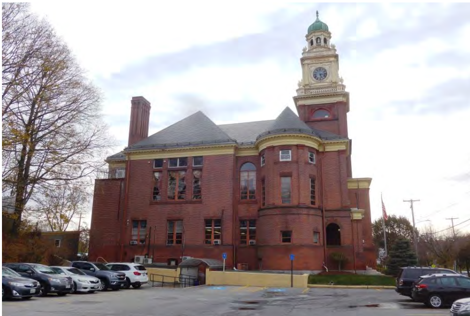
Cumberland Town Hall – Exterior Overalls North Elevation – Overall Note: Ponded water in parking lot
