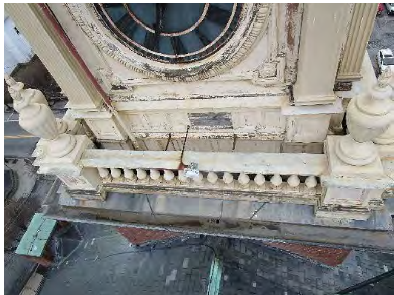
Cumberland Town Hall – Exterior – Wood Elements Tower – Clock Level (Sixth Floor) Overall View - Flaking and Deteriorated Paint – Some Deteriorated Wood
