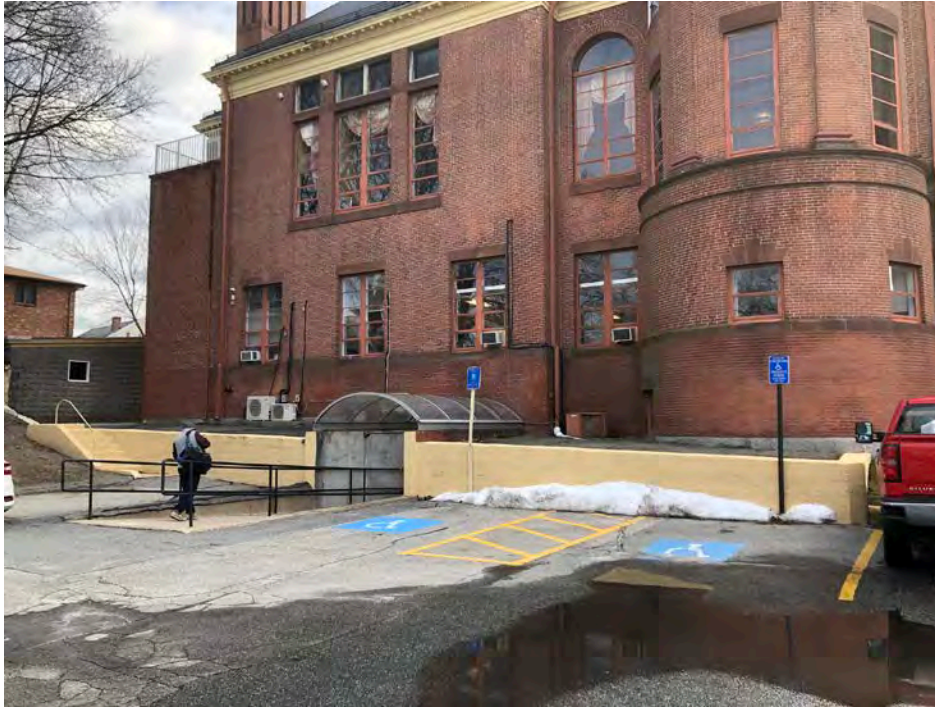
Cumberland Town Hall – Exterior – Retaining Walls, Steps, Landscaping, Asphalt Parking Area and Miscellaneous Landscaping Elements North Elevation – Parking Lot and Raised Platform Adjacent to Building
