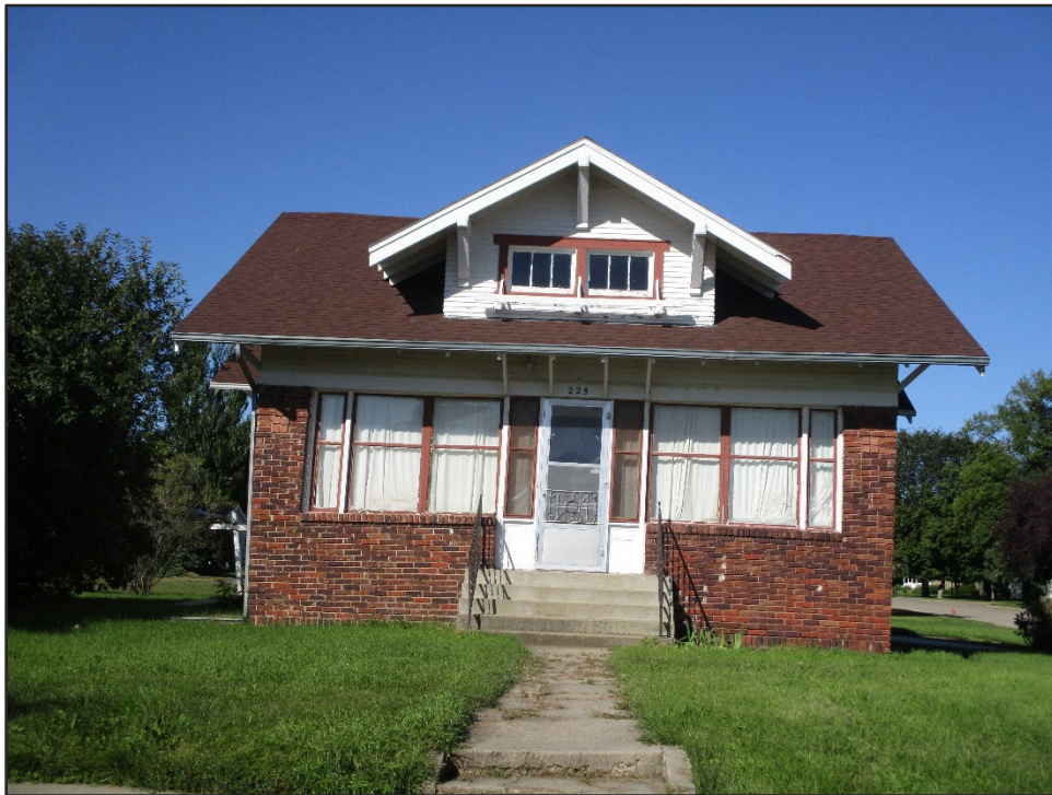
HD-000-00191 – House at 225 W 1st Ave (Miller)
