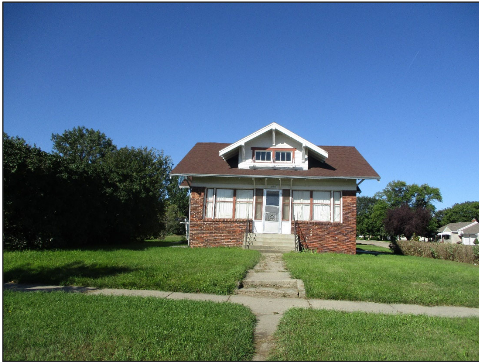
HD-000-00191 – House at 225 W 1st Ave (Miller)
