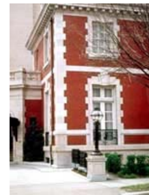
The decorative trim on this brick building is architectural terra-cotta intended to simulate the limestone foundation. Photo: NPS files.
