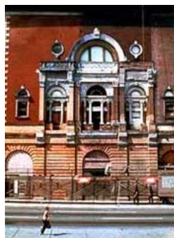
Ninety years of accumulated dirt and pollutants are being removed from this historic theater using an appropriate chemical cleaner, applied in
