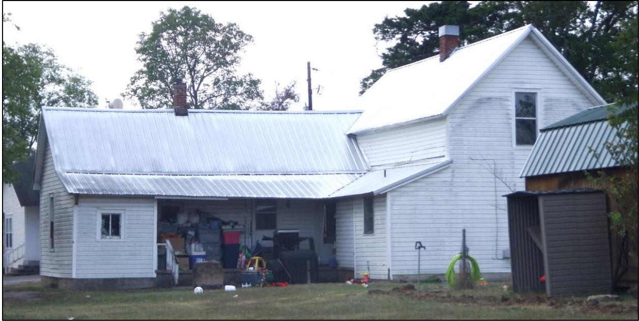
Figure 12. GNAHRGIS Resource 267679 (Gabled Wing Cottage).
