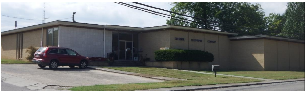
Figure 18. GNAHRGIS Resource 271944 (Trenton Telephone Company).
