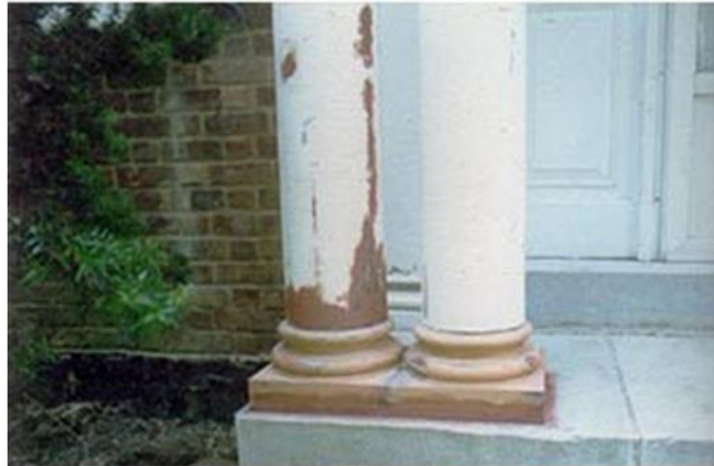
Figure 23 Before and after images of deteriorated wood column bases which have been repaired following the removal of the deteriorated sections, reusing as much historic material as possible.
