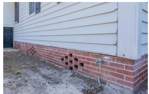
Figure 13 Typical Ford-era brick foundation on Ford Avenue.
