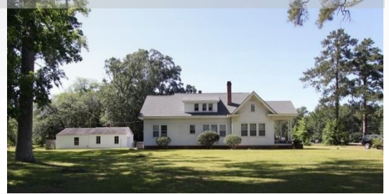
Figure 36 The Mitchum House and garage, which sits at the rear of the property, detached from the main house.
