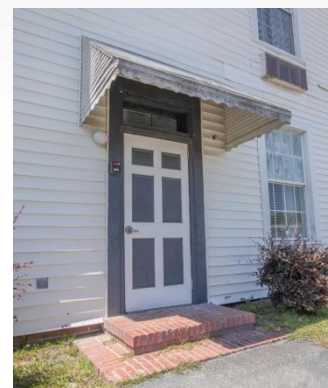
Figure 25 A metal awning that is hiding a historic transom window set above an original entry door.
