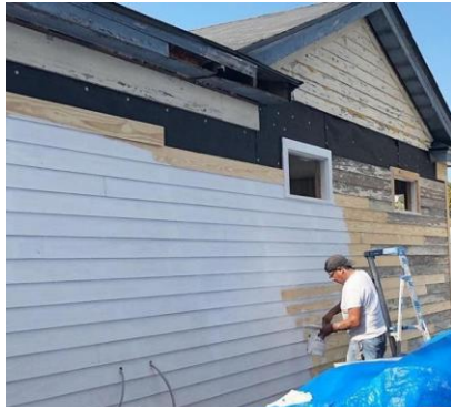
Figure 15 Wood siding repair and replacement and subsequent painting at the Ford Bakery.
