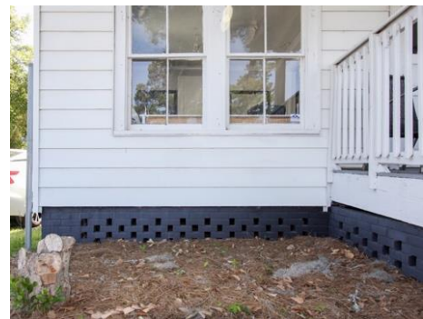
Figure 16 A historic brick foundation that has been painted.
