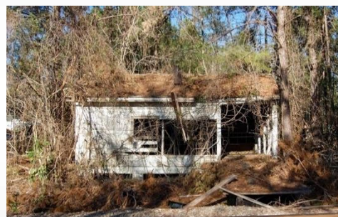
Figure 32 Railroad Postal Delivery Building.
