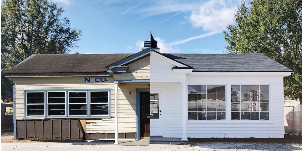
Figure 11 The Ford Bakery before and after rehabilitation.
