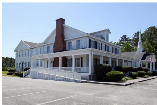
Figure 24 A wood entry ramp which has been placed on the side elevation of the Community House.
