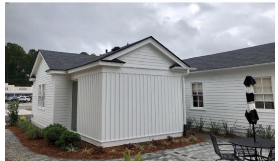
Figure 29 A distinct but compatible addition in board and batten, which has been added to the Ford Bakery. The addition is inset from the corner of the historic building, hidden from view when approaching from Ford Avenue.
