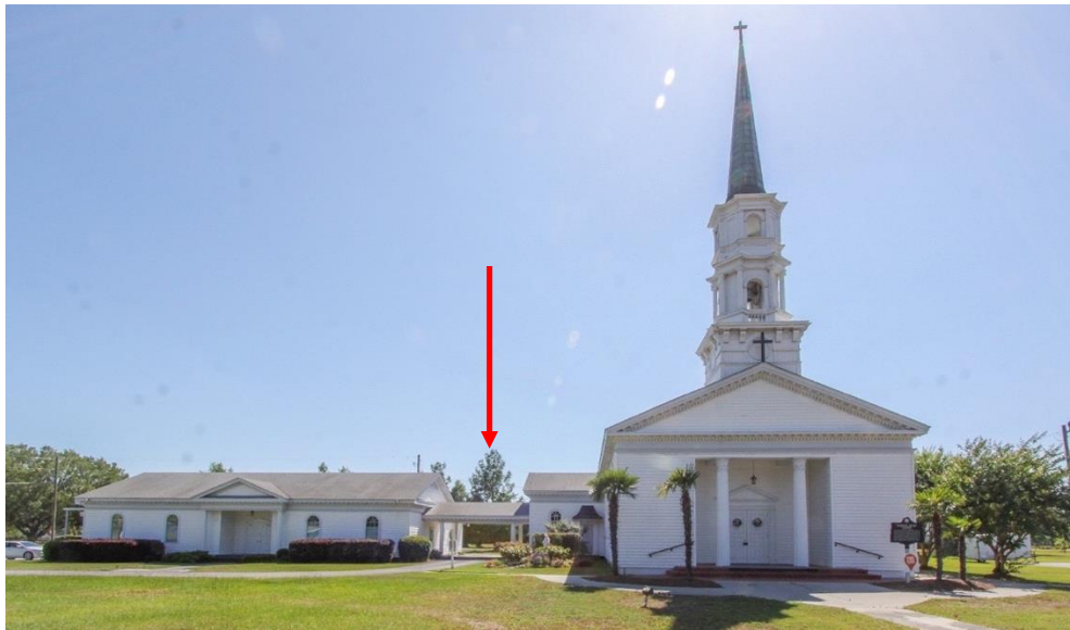
Figure 30 Image illustrating the hyphen used to connect an addition built to accompany the Martha-Mary Chapel.
