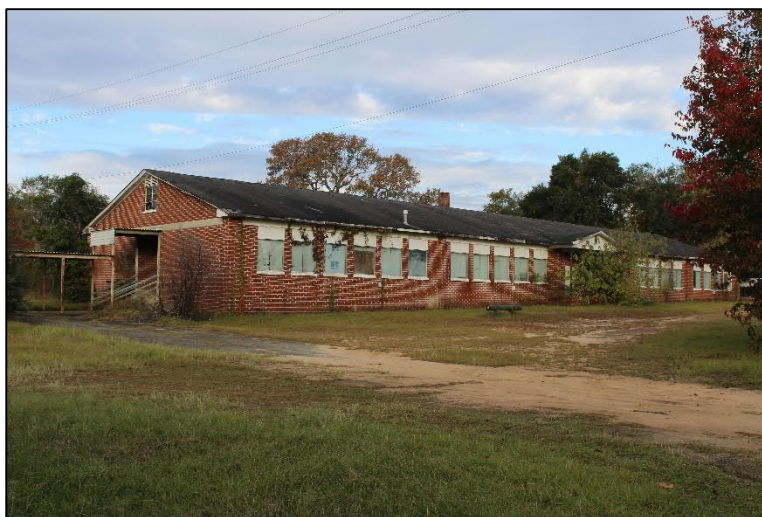
Figure 23: GNAHRGIS ID No. 271562, School Building/Equalization, located at 163 Lumpkin Street.
