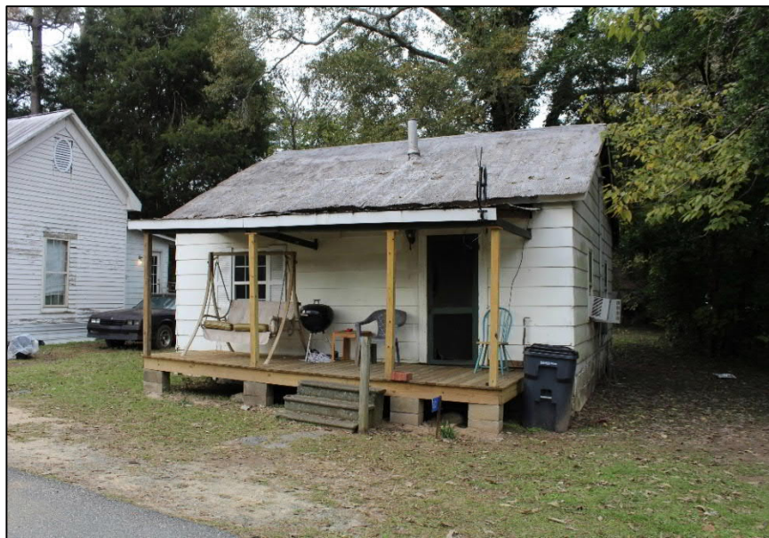
Figure 15: GNAHRGIS ID No. 272062, Side Gabled Cottage Type, located at 23 Railroad Street.
