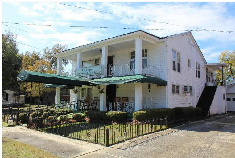
Figure 30: GNAHRGIS ID No. 273617, Neoclassical Revival Style, located at 223 North Dooley Street.
