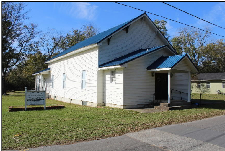
Figure 20: GNAHRGIS ID No. 269371, Front Gable church Type, located at 43 Henry Way.
