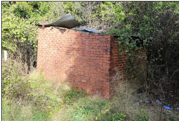
Figure 25: GNAHRGIS ID No. 269406, Storage Shed Type, located on Anderson Lane.
