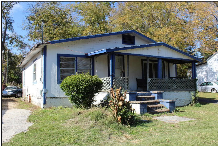
Figure 13: GNAHRGIS ID No. 273615, Bungalow Type, located at 231 North Dooley Street.
