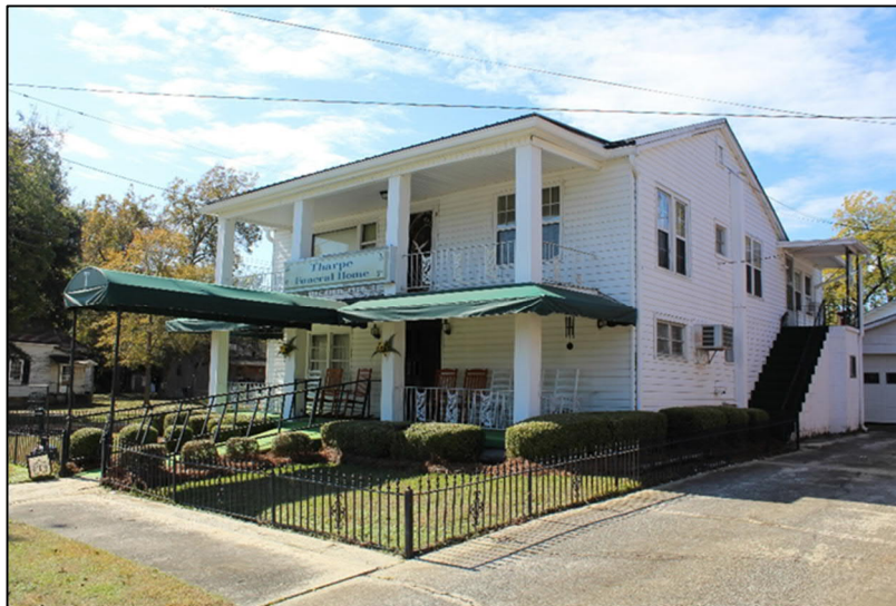
Figure 14: GNAHRGIS ID No. 273617, Georgian House Type, located at 223 North Dooley Street.
