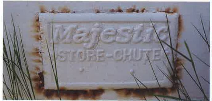
Photograph 5: Majestic Store-Chute on Grey School foundation.
