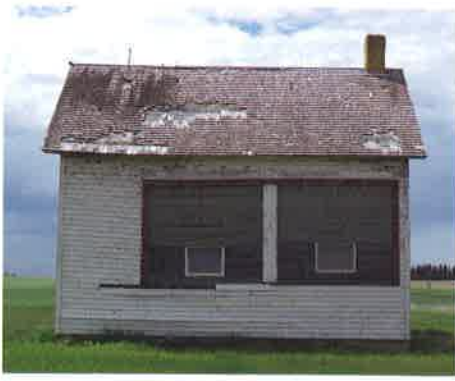
Photograph 3: Glass block window replacements on McGill School.
