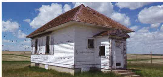
Photograph 11: Grey School, showing coal chute in foundation.
