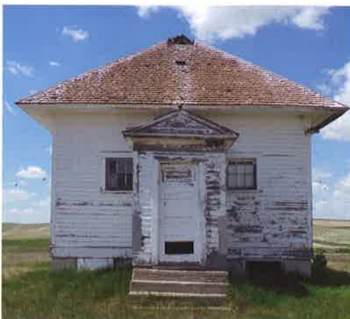
Photograph 4: Prefabricated door, siding, and trim on Grey School.
