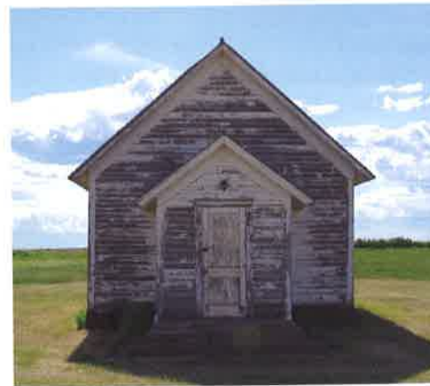
Photograph 2: External entry vestibule on Hartsoch school.
