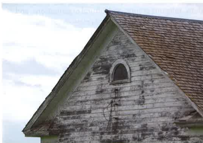
Photograph 7: Decorative eave returns and semi-circular attic window on Thull School.
