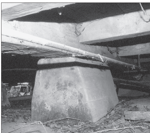
Fig. 19 Cypress trapezoidal sill support block, the Ram Trouille house, St. Landry Parish, LA, 2005. Author photo.
