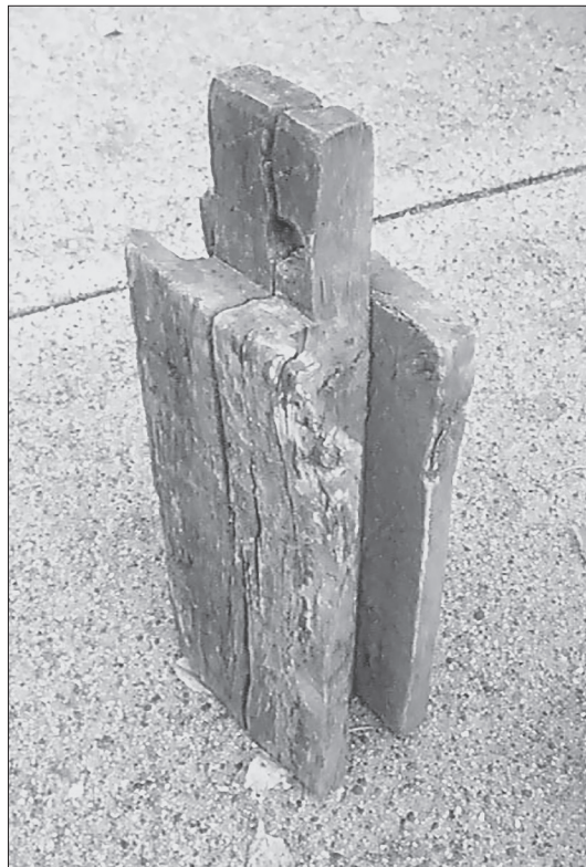
Fig. 15 Top section of tenon en coulisse post, the Lasource-Durand house, Ste. Genevieve, MO, 1998. Author photo.
