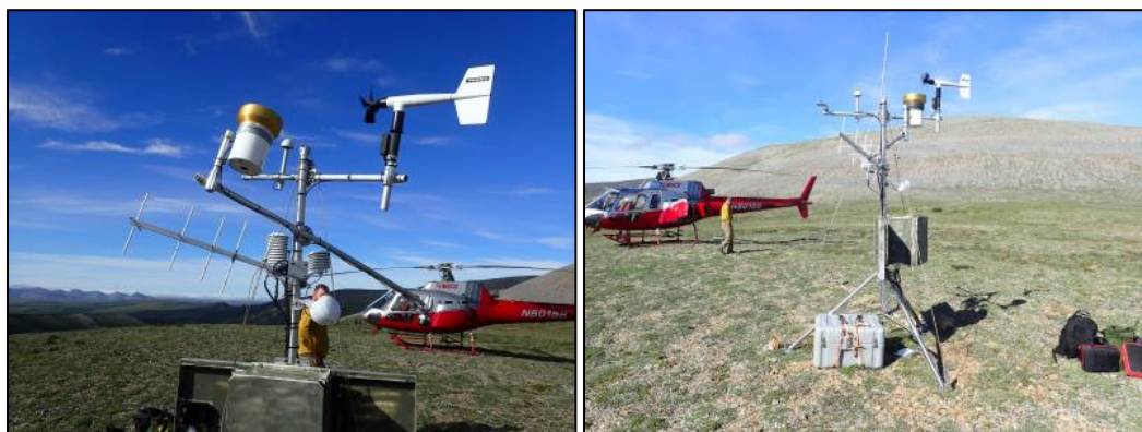
Figure 15. Asik climate station before (left) and after (right) maintenance, July 27, 2017.
