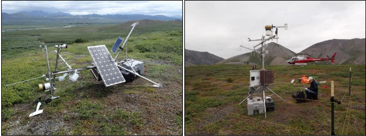
Figure 14. Kugururok climate station had been damaged by a bear (left). The station was repaired on July 21, 2018, only two days after the damage occurred (right).
