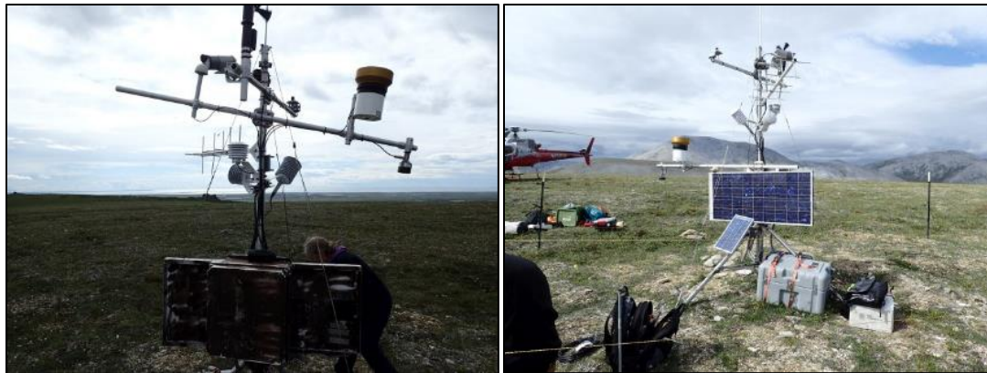
Figure 18. Mt. Noak climate station July 22, 2018 before (left) and after (right) repairs.
