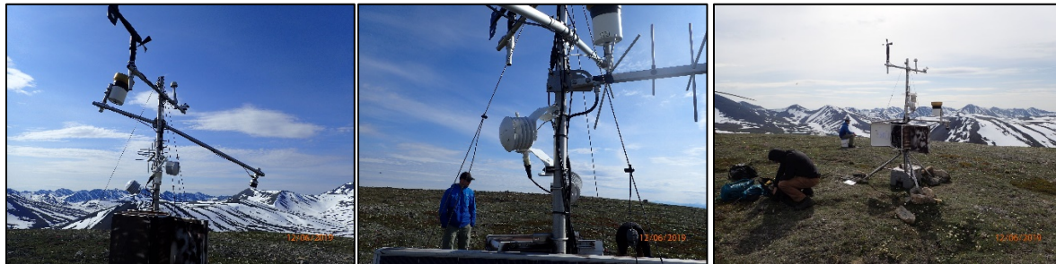
Figure 8. Kaluich climate station June 12, 2019. Before (left, middle) and after (right) repairs.
