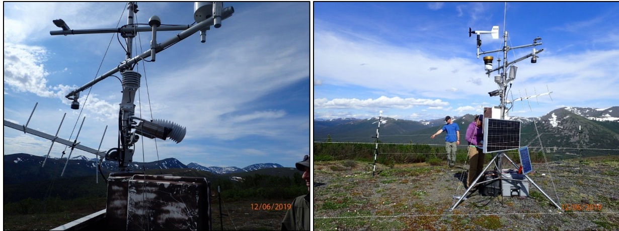
Figure 10. Salmon River climate station June 12, 2019 before (left) and after (right) repairs.
