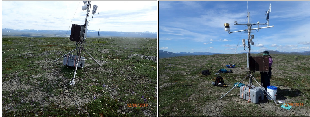
Figure 9. Sisiak climate station June 12, 2019 before (left) and after (right) repairs.
