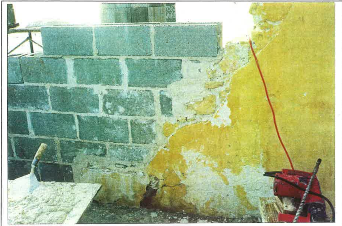
Concrete block was attached to the existing stone work with 3/4 inch galvanized rods anchored horizontally at 16 inch intervals
