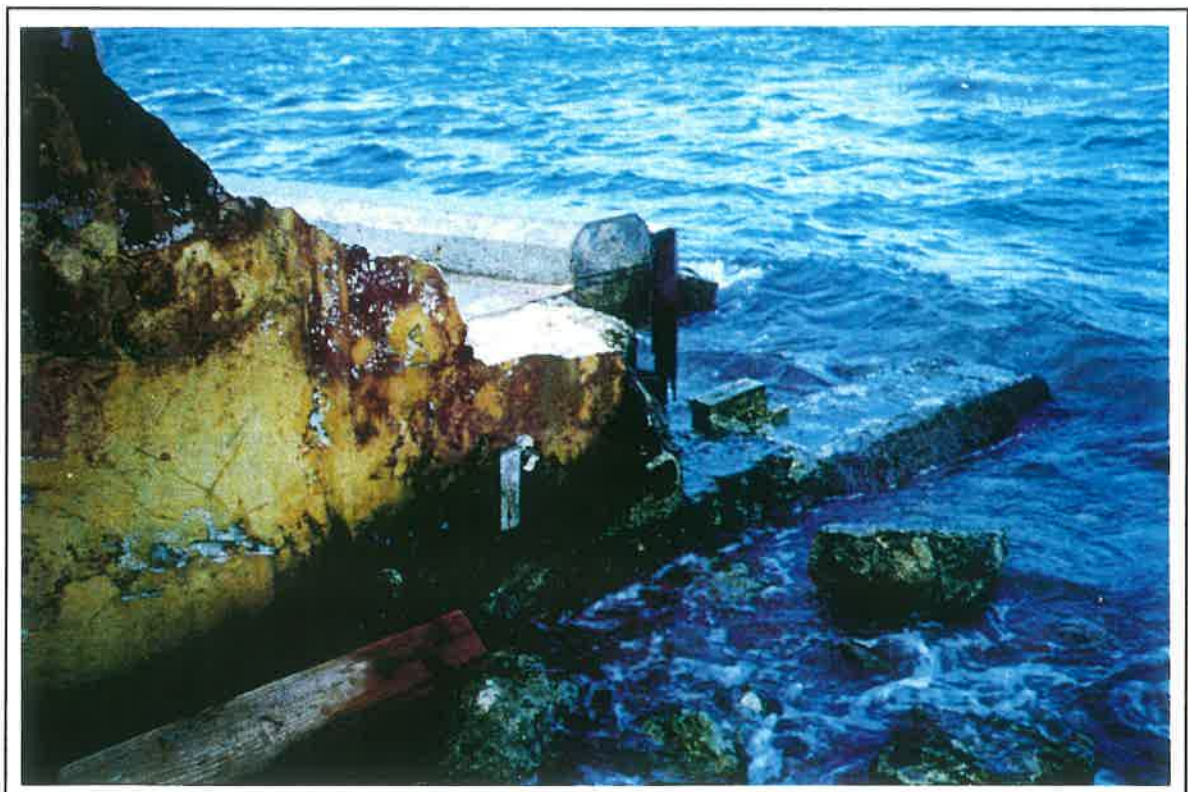
Concrete footing was repaired and reused for wingwall extension
