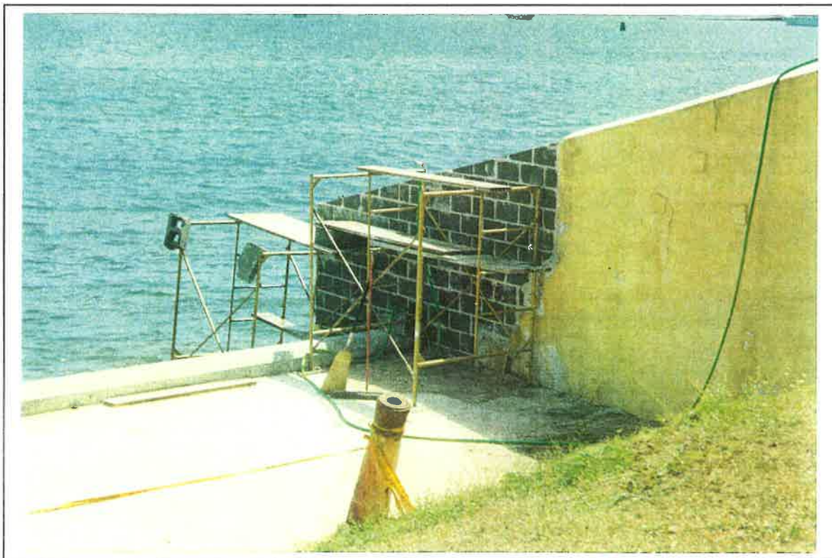
The finished wall prior to stucco application
