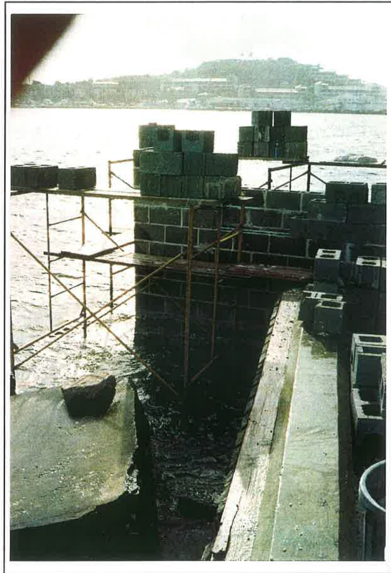
Scaffold was erected in the water in order to rebuild the wall
