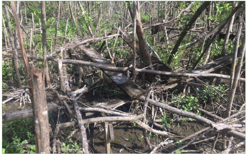
Figure 4. Hurricane damage at the Salt River SARI SET site. Severe wind damage caused debris deposits, mangrove die-off, and missing or damaged platform boards.
