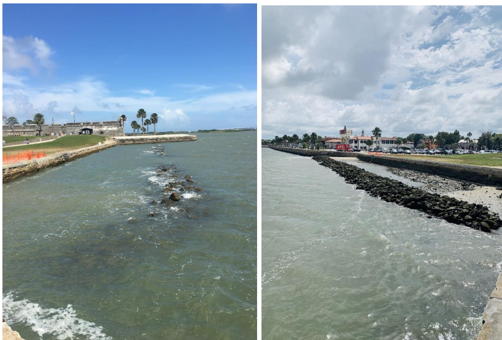
Figure 13: South Wall at High and Low Tide
