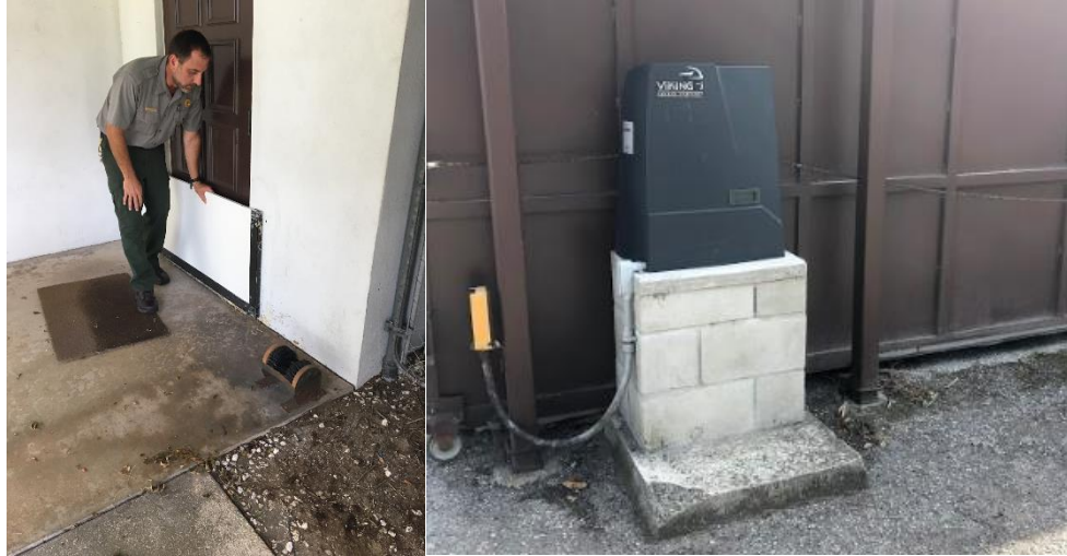
Figure 11: Headquarters Raised Structures and Flood Walls
