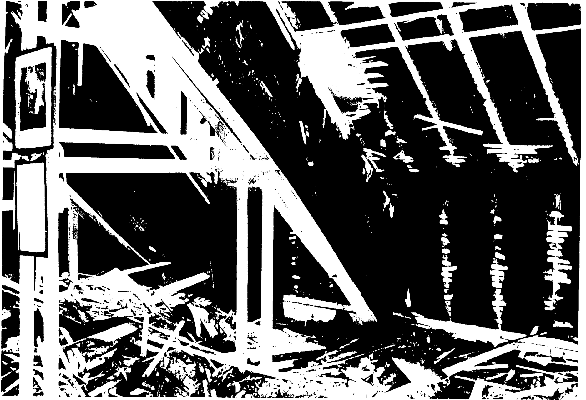
Illustration 72. North Side of Garret, East End, Looking West, Old State House (1921).
