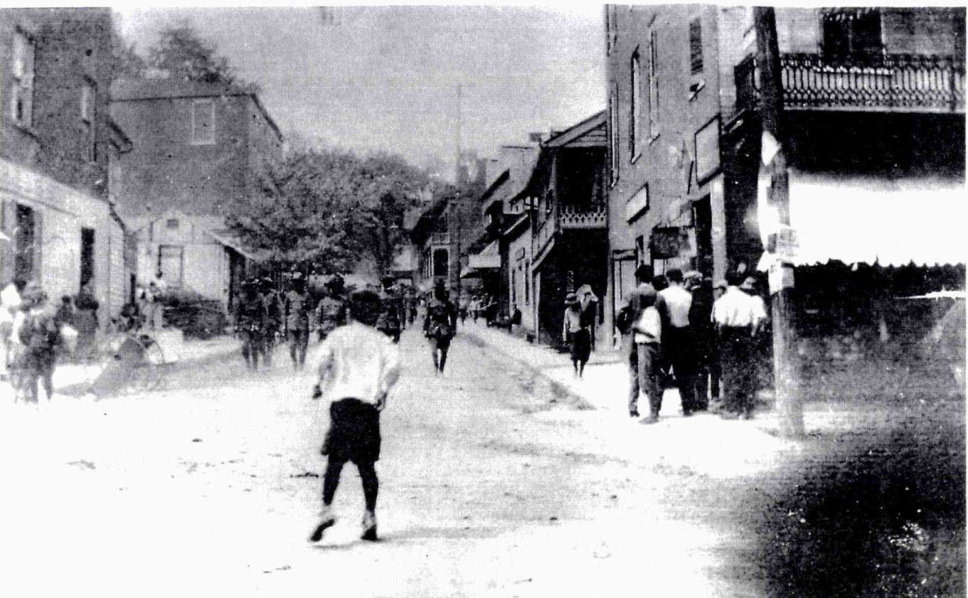
Figure 7. HF-378. Looking up High Street, ca. 1910. Building 3 is on the left beyond the small frame building.
