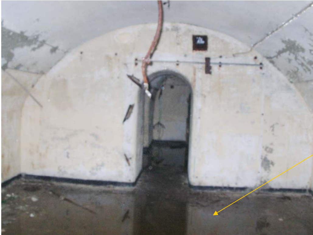
Magazine Tunnel (J)
