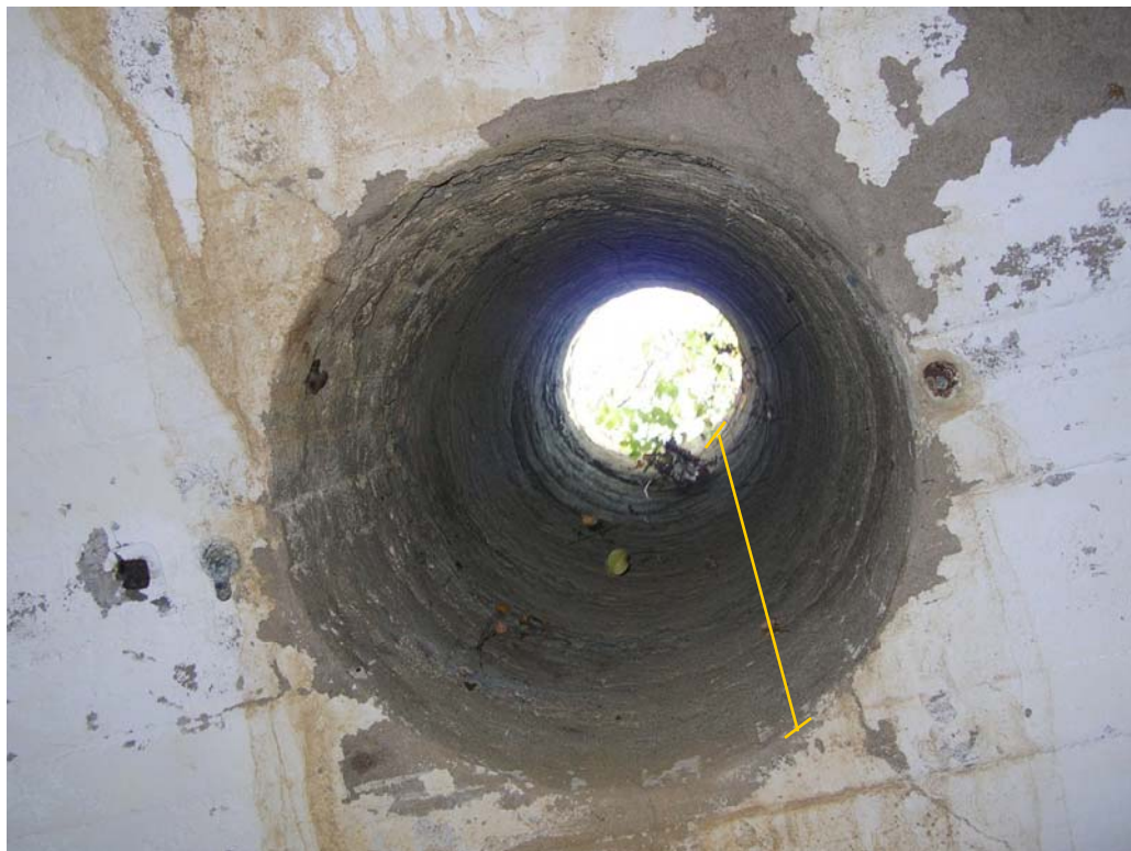
North Transverse Gallery (Y)
