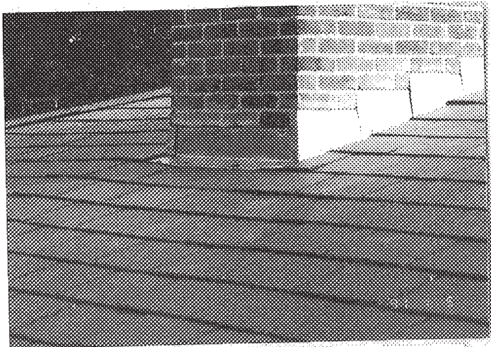
Step flashing.
