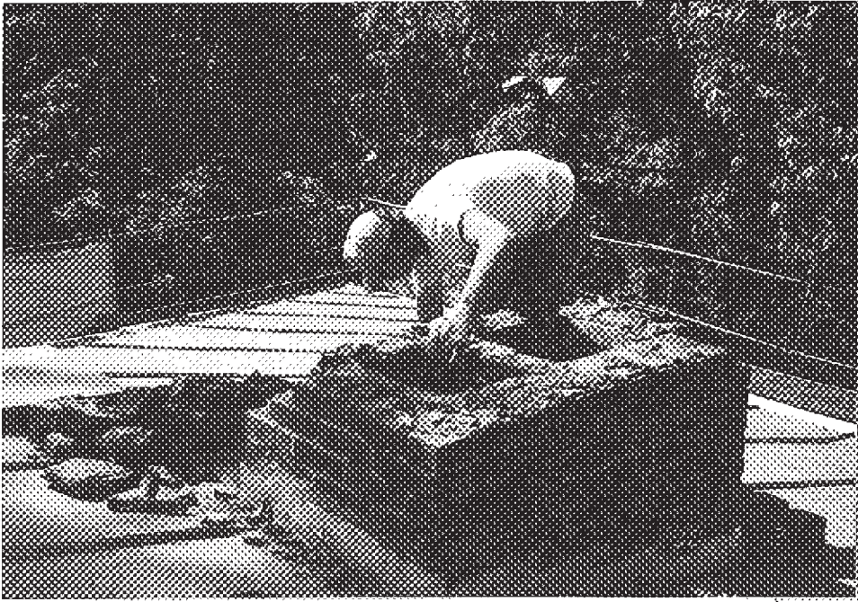
Chimney repair and rebuilt. Bldg 58
