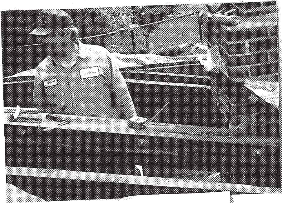
Install 2-cax7.25 each side of the top cord. Bldg 57
