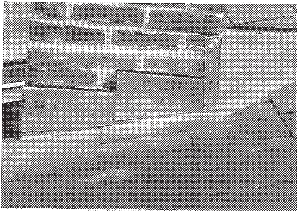
Typical counterflash set into brick joint.
