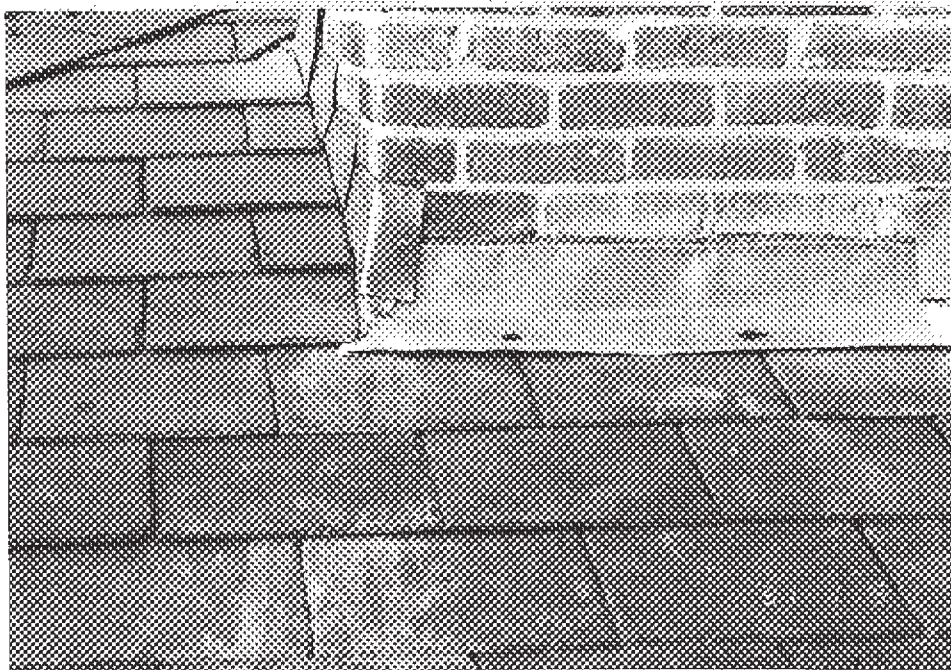
Step flashing.
