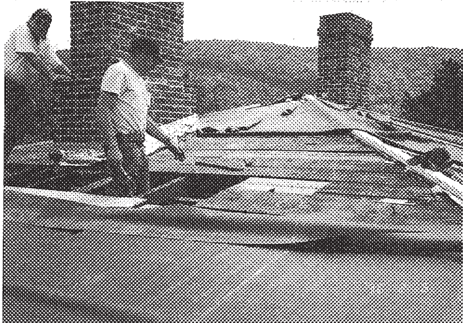
Demolition of existing metal roof. Bldg 57
