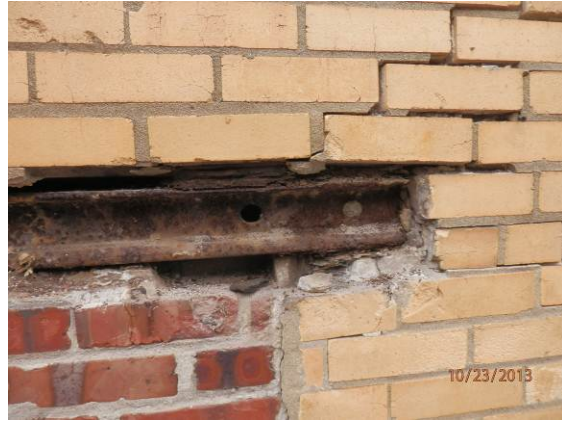
Image 9 – At W-4 probe location, railroad track sections used as a lintel.
