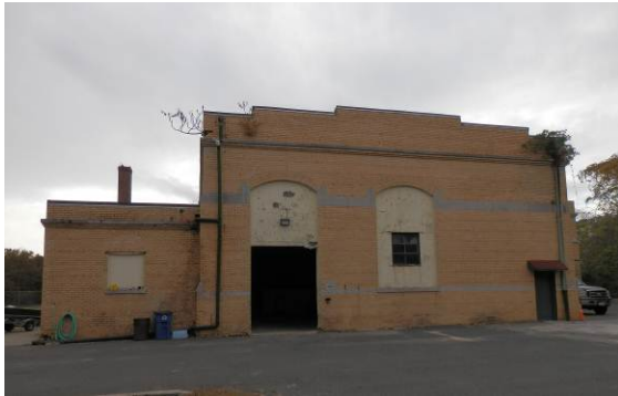
Image 1– North elevation of the Water Plant.
