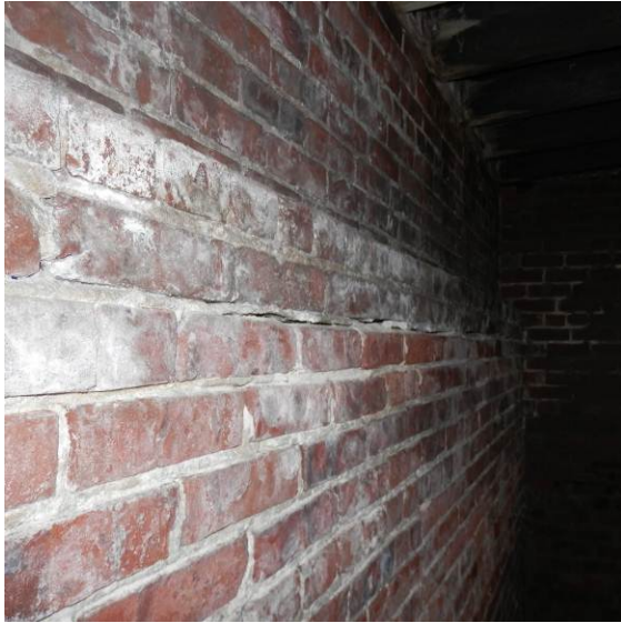
Image 11 – Horizontal crack running two courses below truss as seen at probe location T-3 (see Image 16).
