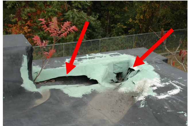
Figure 3: Diagram of the Parapet wall and the southeast corner of Building A showing typical large holes in roof membrane near scupper.
