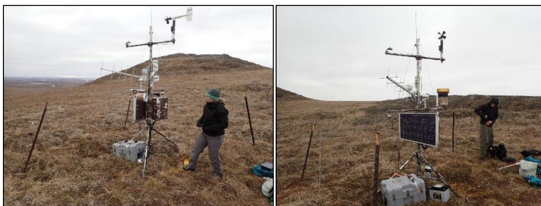
Figure 15. Devil Mountain climate station June 4, 2021, before (left) and after (right) repairs.
