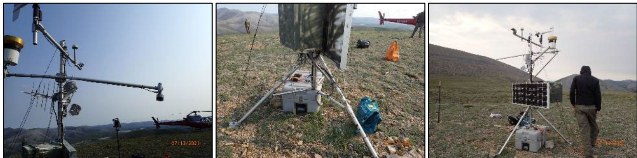
Figure 6. Asik climate station July 13, 2021. The crossarms were out of level (left) and the sensor cables had been pulled out at the enclosure (middle). The station was repaired (right).
