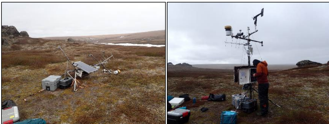
Figure 18. Serpentine climate station June 4, 2021, before (left) and after (right) repairs.
