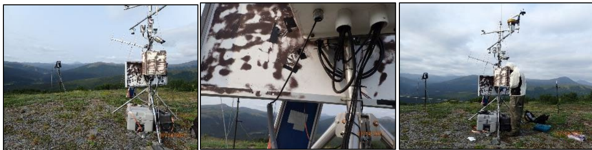
Figure 12. Salmon River climate station July 14, 2021. The camera had been disoriented (left) and some cables had been pulled on at the enclosure (middle). The station was repaired (right).
