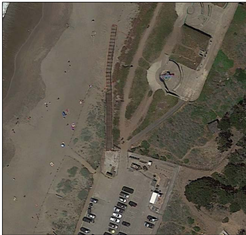
Figure 1 - Google Earth Aerial Imagery from May 2018 Showing In-progress Construction of Accessible Ramp
