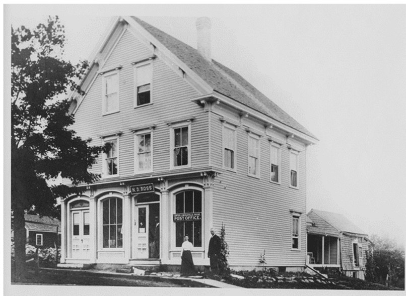
Figure 3. Historic photo of the N.D. Ross store and Post Office (present-day Lincolnville General Store Resource No. 23) (Courtesy of Walsh History Center)
