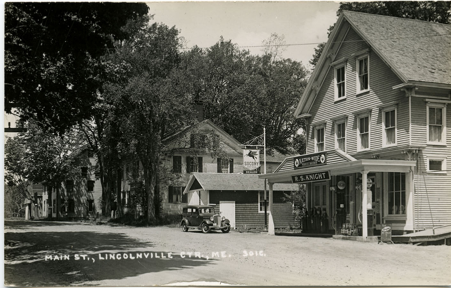
Figure 4. View southeast showing the historic R.S. Knight store (present-day Lincolnville General Store Resource No. 23 and 273 Main Street Resource No. 24) (Courtesy of Walsh History Center)
