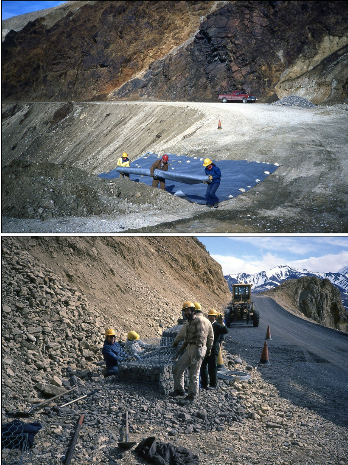
Figure 2. (TOP) Installing geosynthetic layer reinforcement along the road surface which cross cuts the landslide. Photo taken 1987. (BOTTOM) Installing a French drain near the northwestern lateral scarp (i.e. road crack) location. Photo taken 1987.
