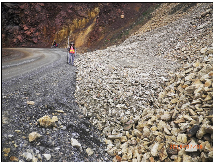
Figure 13. (TOP) Debris flow paths and deposits seen looking northeast. Scarp and deposits highlighted for clarity. Eastern lobe extends beyond photo frame, see B. (BOTTOM) Larger (eastern) debris flow's lobe deposit as diverted by ditch. Photo taken looking northwest.
