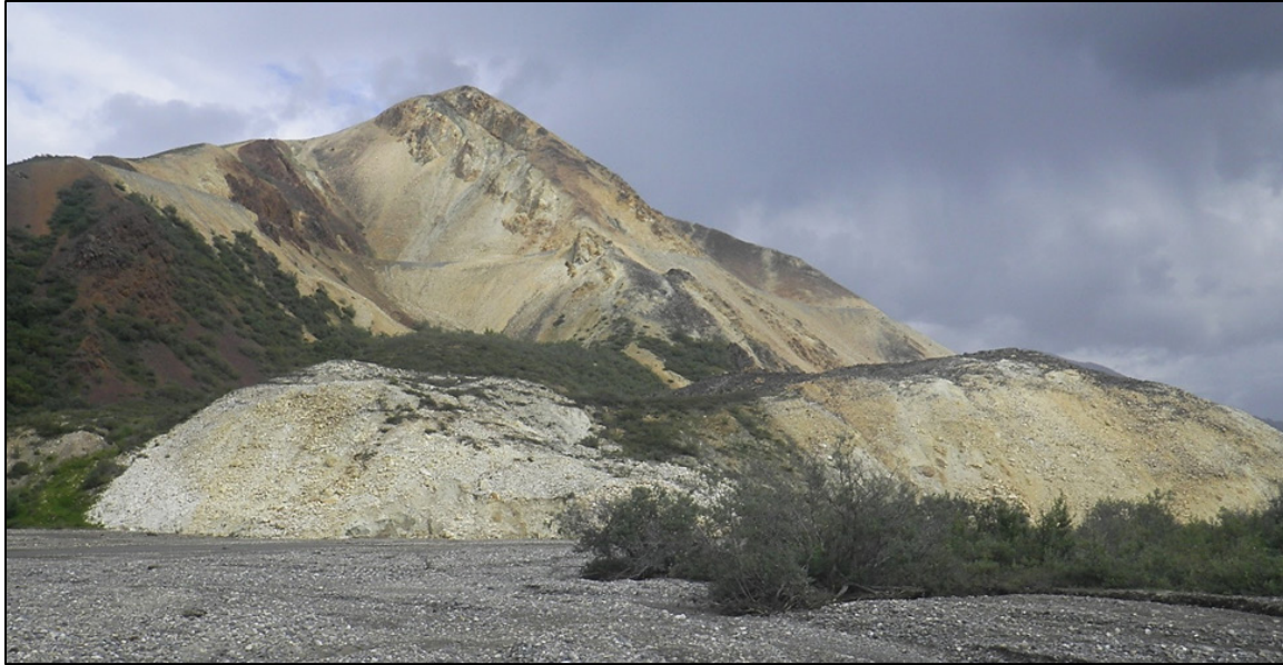
Figure 16. Pretty Rocks Landslide and associated lobe deposits seen from the East Fork Toklat River tributary. Road visible in upper slope for scale. Photo taken looking north.
