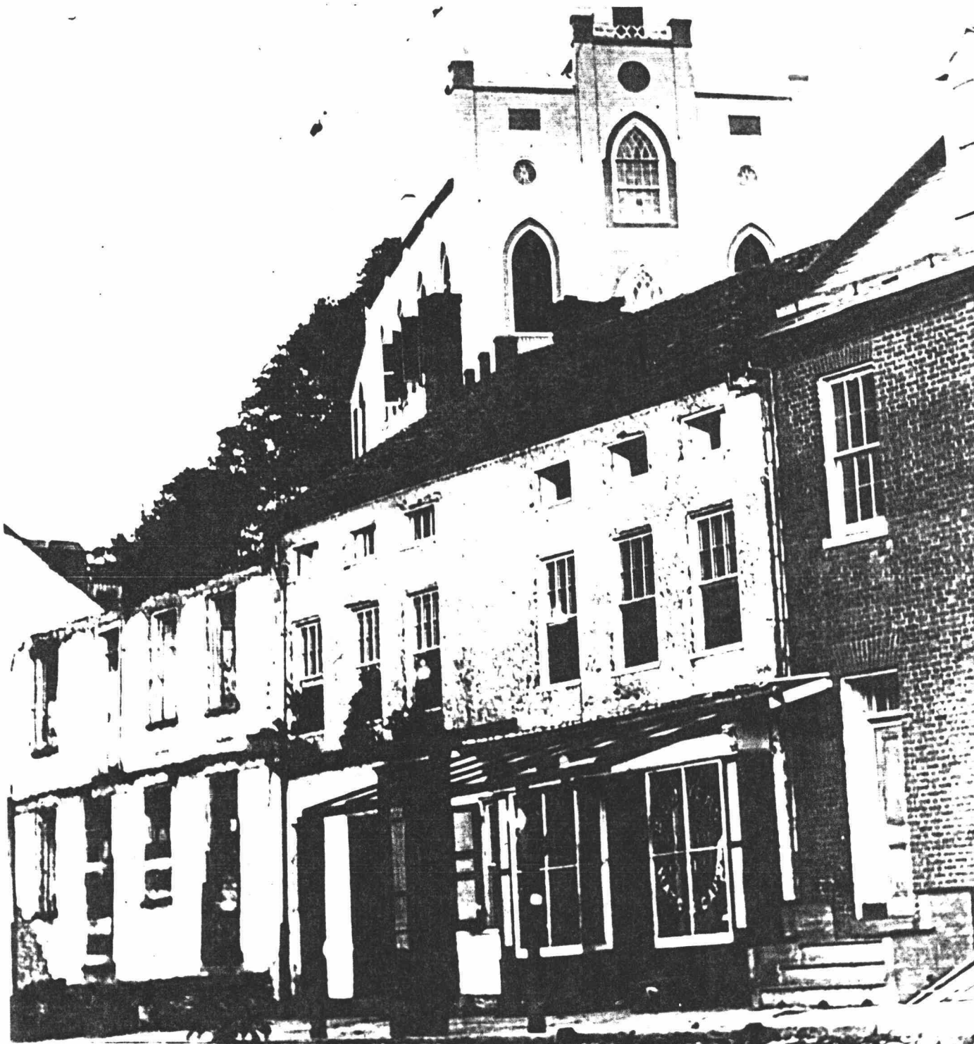
Figure 4 -- View of Shenandoah Street after the Civil War (HF-35). Building 38 is in the center, burned-out Building 40 to its left, then Lot 48, and east wall of Building 43 on far left.
