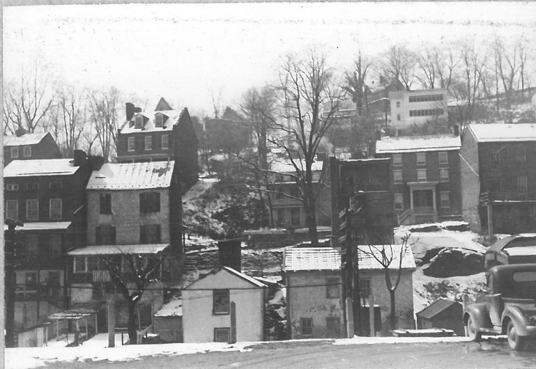
3. View in Harpers Ferry from B&O railroad station.
