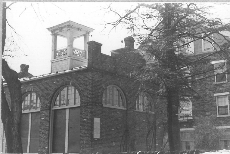
8. Corner view of engine house.
