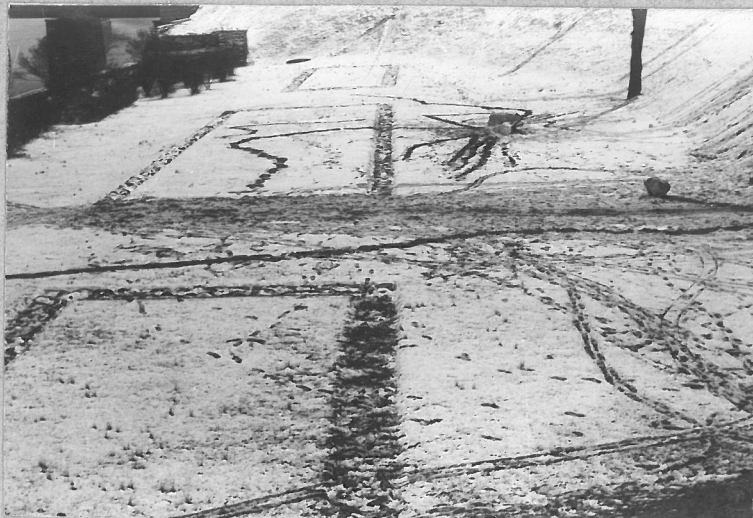
4. Foundation outline of arsenal and engine house where John Brown was captured, Harpers Ferry. This is B&O railroad property. View is from the railroad station.
