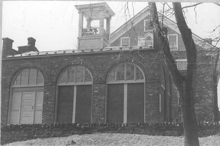
7. Side view of engine house.
