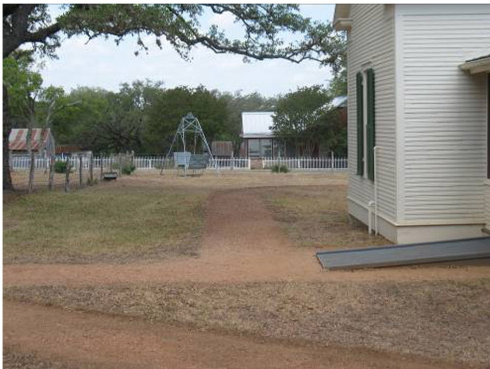
Convergence of dirt footpaths and ADA ramp at the back elevation of the LBJ Boyhood Home (HB-1), facing west (Source: M. Frisbie).
