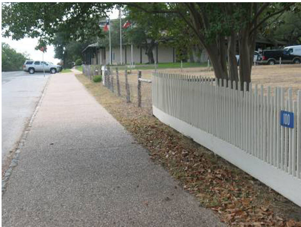
The LBJ Boyhood Home Fences and Gates (HB-1.B), on Elm Street with woven wire and picket fences, facing east (Source: M. Frisbie).
