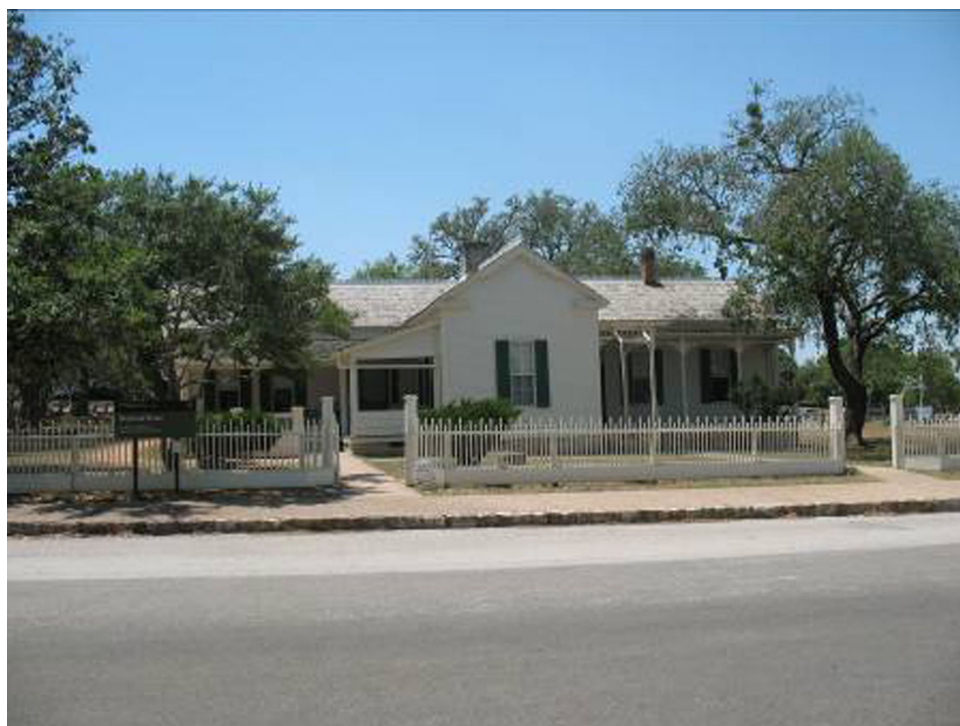
The restored LBJ Boyhood Home (HB-1) north elevation with picket fences (HB-1.B), facing south (Source: M. Frisbie).
