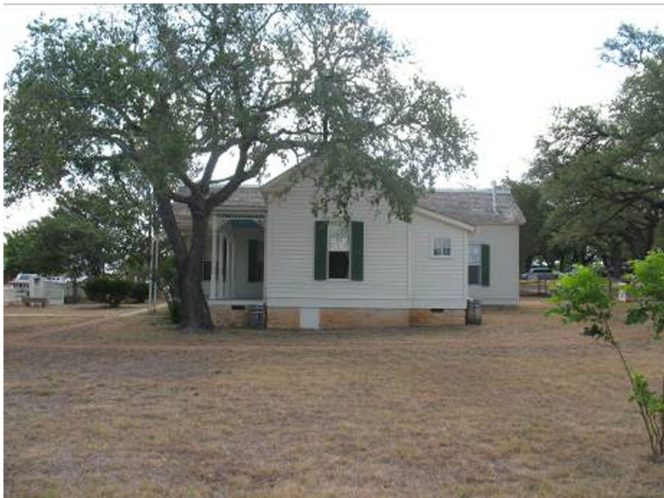
The west elevation of the restored LBJ Boyhood Home (HB-1), facing east (Source: M. Frisbie).
