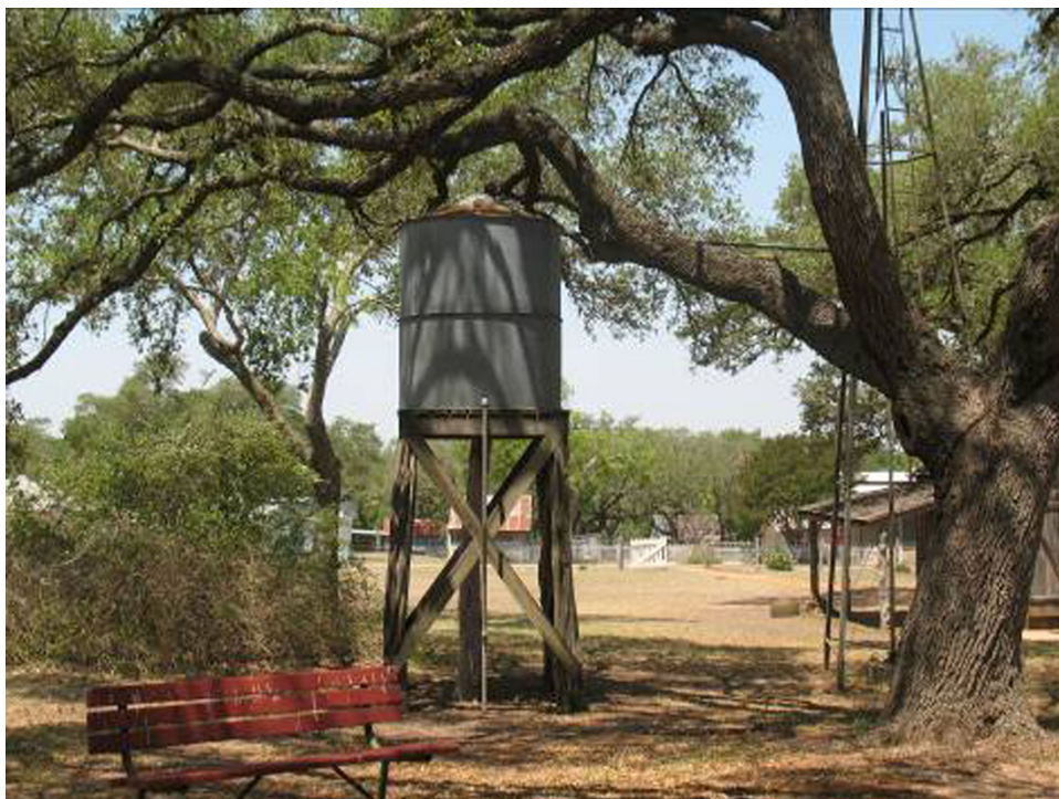
The reconstructed LBJ Boyhood Home Water Tower (HB-6), next to base of LBJ Boyhood Home Windmill (HB-5), facing west (Source: M. Frisbie).
