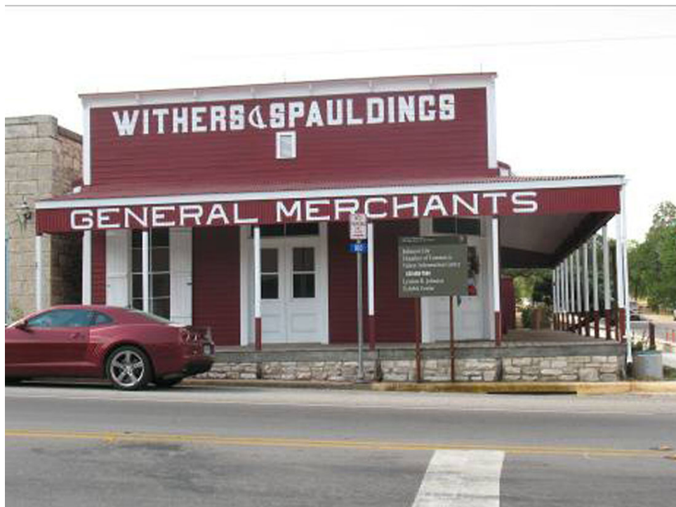
The Withers-SpaULDING Building (HB-43) on Main Street/Highway 290, facing south (Source: M. Frisbie).
