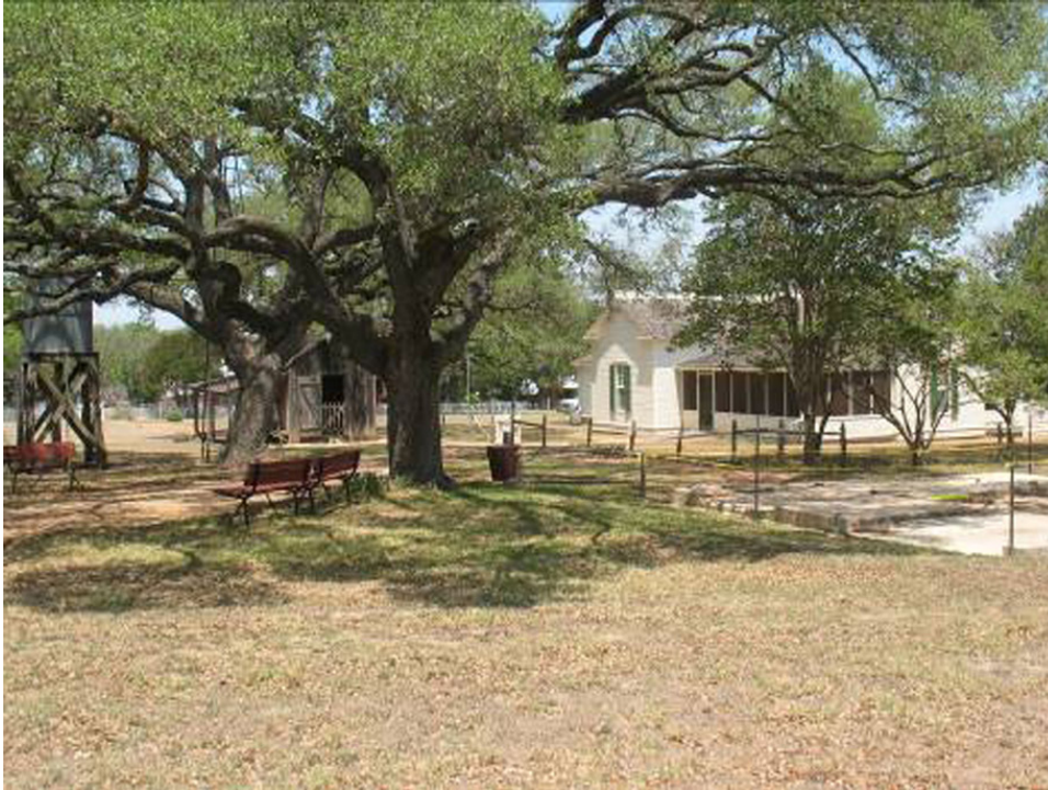
From left to right, the LBJ Boyhood Home Water Tower (HB-6), the LBJ Boyhood Home Windmill (HB-6) (obscured), the LBJ Boyhood Home Smokehouse/Shed (HB-3), and the LBJ Boyhood Home (HB-1), facing northwest (Source: M. Frisbie).
