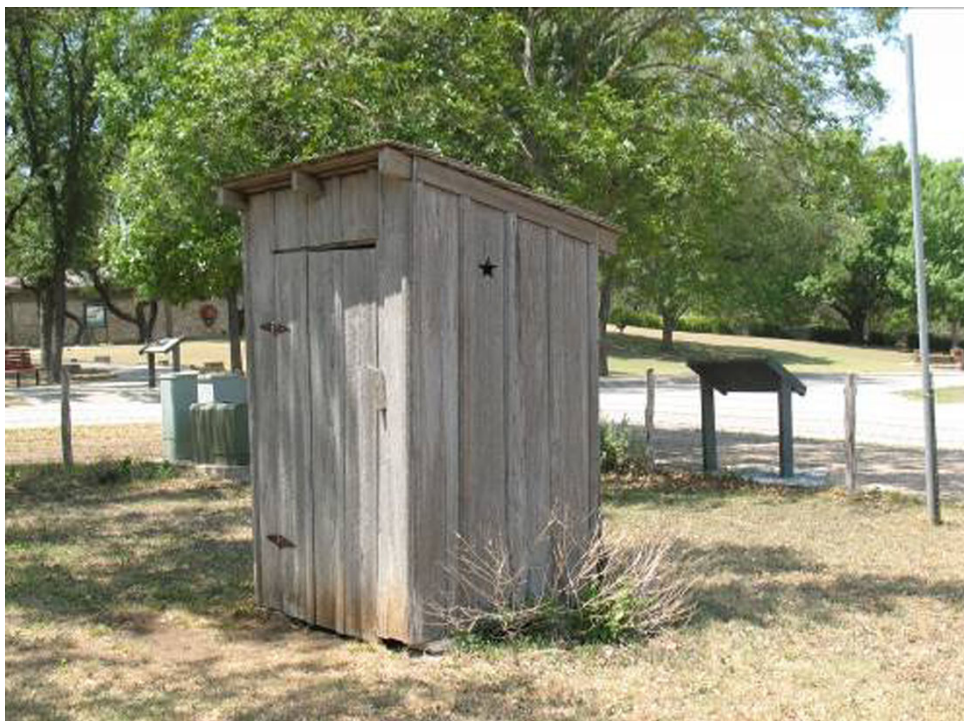
The reconstructed LBJ Boyhood Home Privy (HB-4) in southwestern corner of Block 25 with Visitor Center (HB-100) across the street in background, facing southwest (Source: M. Frisbie).
