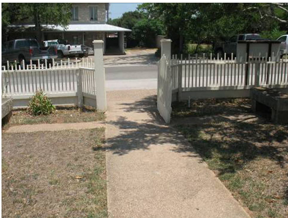
East entrance through picket fence and concrete walkway to LBJ Boyhood Home (HB-1), facing north (Source: M. Frisbie).
