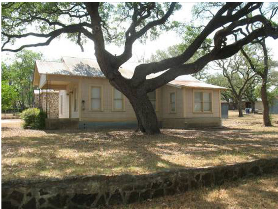
The Moore House (HB-102), with Cantwell House (HB-101) in the background, facing east (Source: M. Frisbie).
