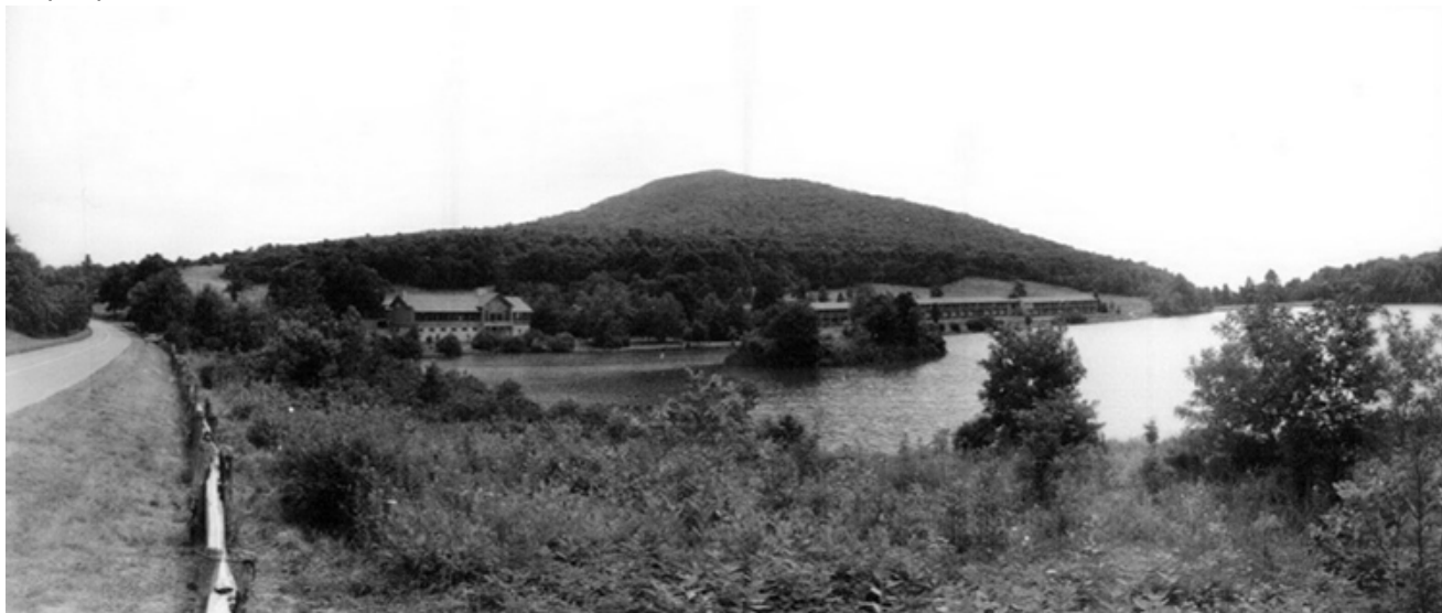
FIGURE 8. The Peaks of Otter Lodge under construction in 1963 (2012 Peaks of Otter Cultural Landscape Report).
