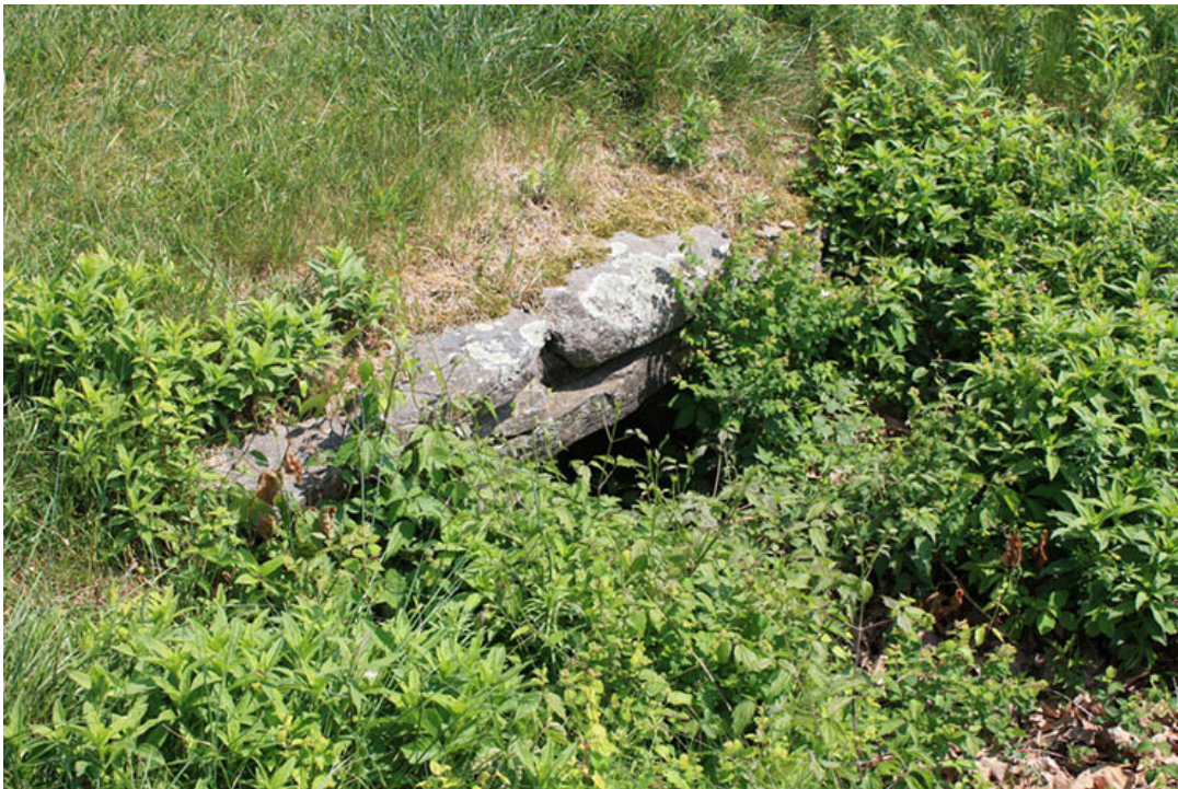
FIGURE 30. A stone-faced headwall associated with a culvert conveying stormwater under the parkway (2012 Humpback Rocks Cultural Landscape Report).
