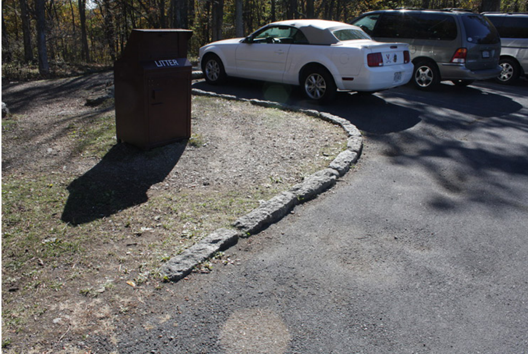
FIGURE 31. Stone curbing edges the parking area and tapers to meet the asphalt; bear proof trash receptacle post-dates the period of significance (2012 Humpback Rocks Cultural Landscape Report).
