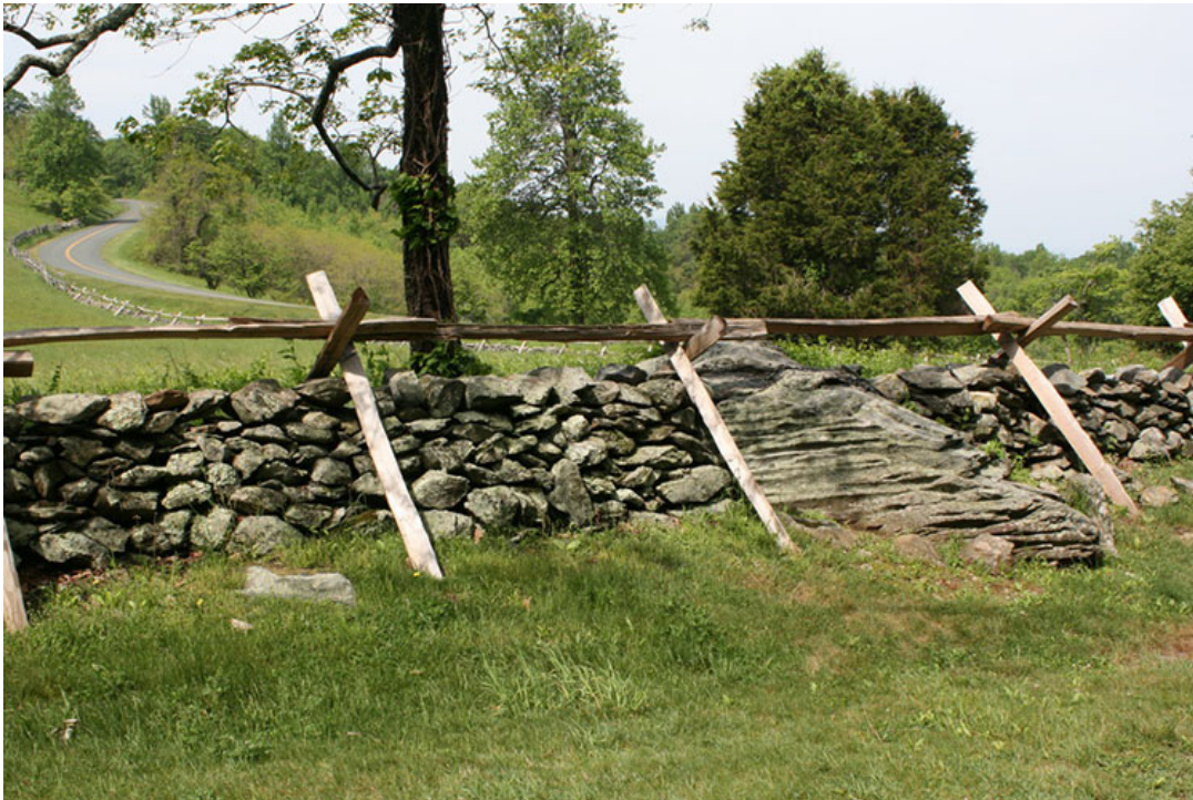
FIGURE 29. A rock outcrop set within the stone and rider fence along the Humpback Gap parking area road (2012 Humpback Rocks Cultural Landscape Report).
