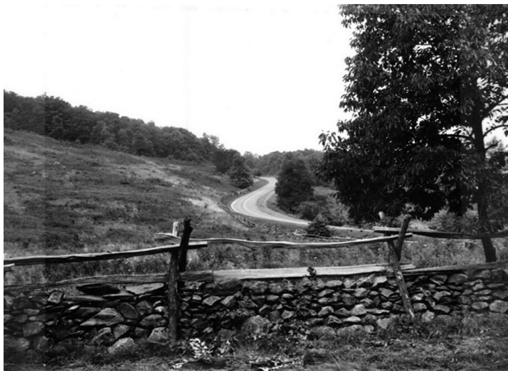
FIGURE 13. The Blue Ridge Parkway from the Humpback Gap parking access road, 1973 (2012 Humpback Rocks Cultural Landscape Report).
