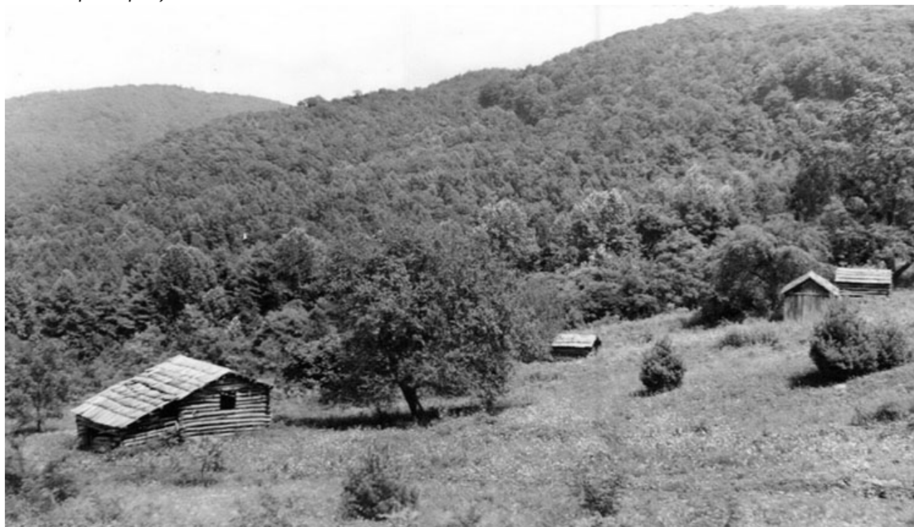
FIGURE 10. Rehabilitation of the root cellar at Humpback Rocks in 1953 (2012 Humpback Rocks Cultural Landscape Report).
