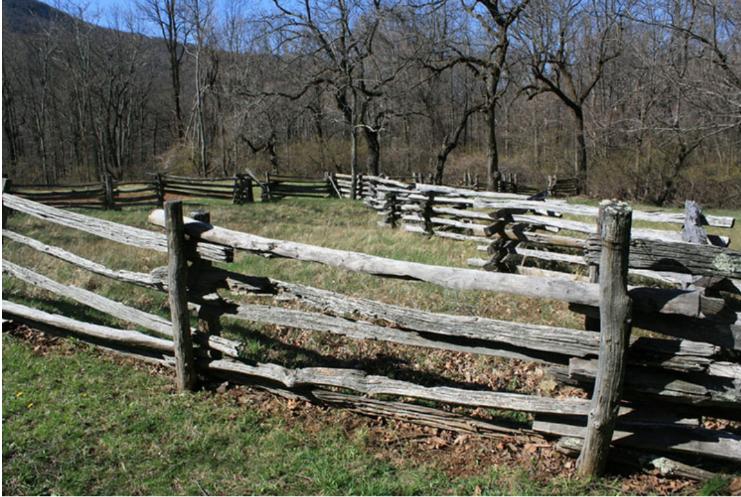
FIGURE 41. Five rail post-and-rail fencing edges a small pasture near the Mountain Farm (2012 Humpback Rocks Cultural Landscape Report).
