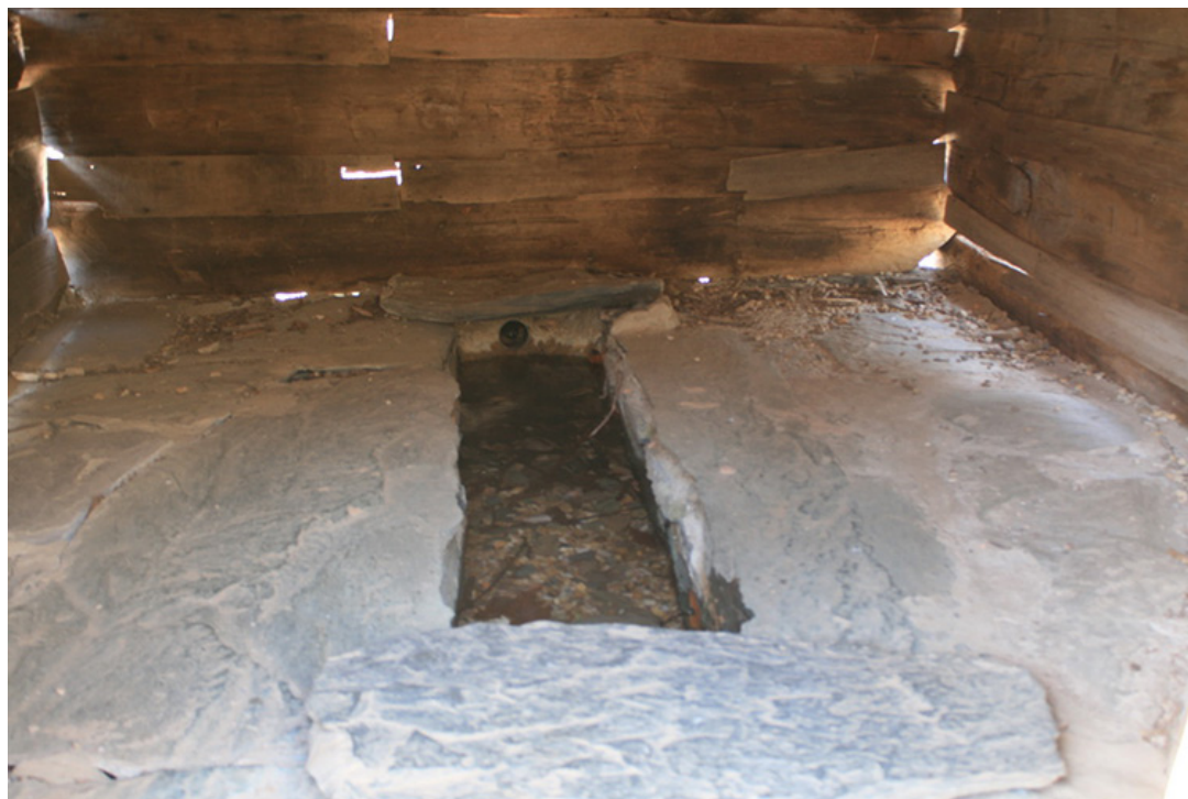
FIGURE 43. A stone-lined pool captures water in the interior of the spring house (2012 Humpback Rocks Cultural Landscape Report).
