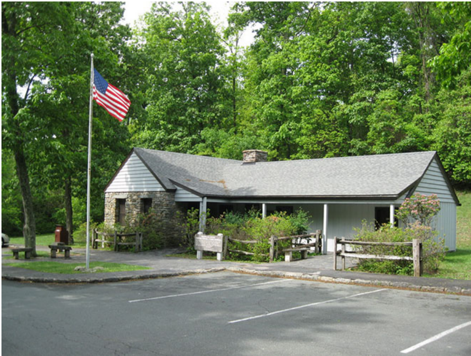
FIGURE 26. The new visitor center, as seen from the adjacent parking lot (2012 Humpback Rocks Cultural Landscape Report).
