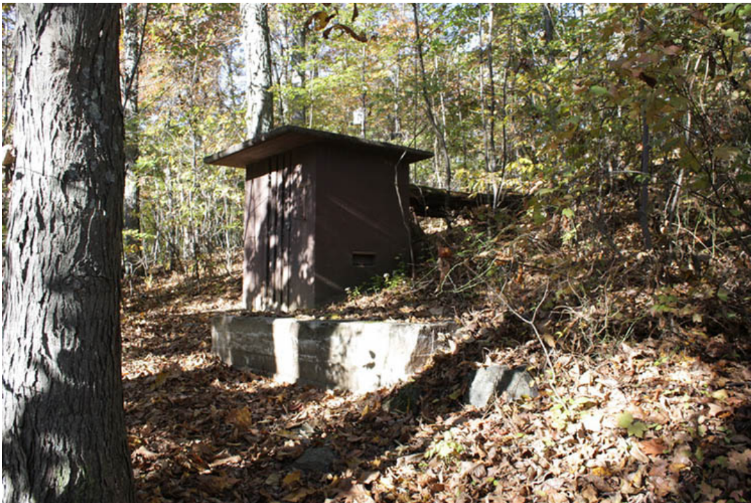
FIGURE 27. The pump house behind the visitor center. (2012 Humpback Rocks Cultural Landscape Report).
