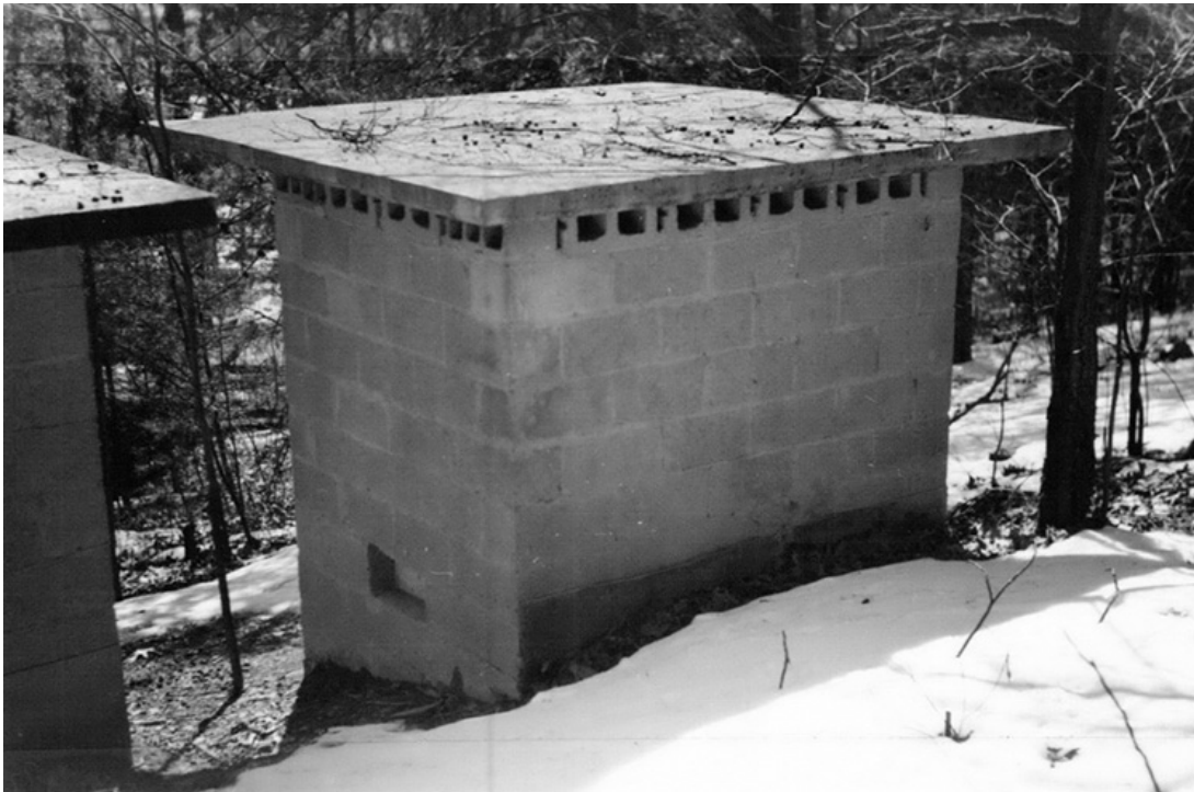
FIGURE 25. March 1958 view of possible former pump house is at left; structure at center no longer exists (2012 Humpback Rocks Cultural Landscape Report).
