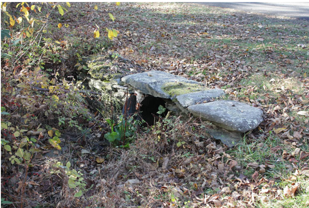
FIGURE 29. A stone headwall and culvert near the visitor center (2012 Humpback Rocks Cultural Landscape Report).
