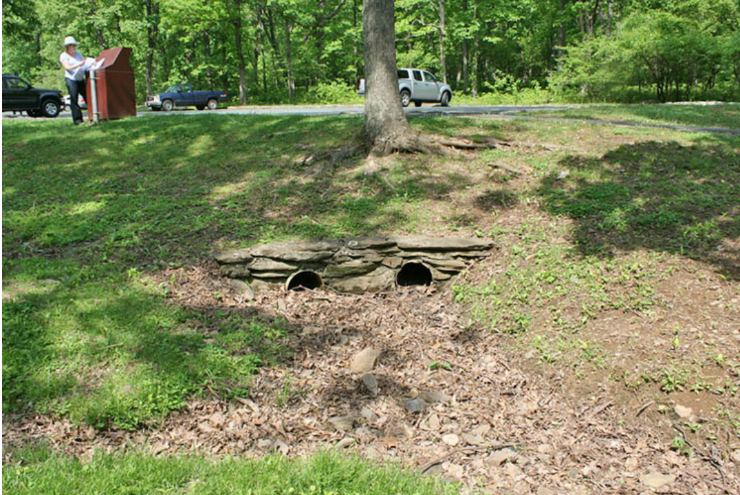
FIGURE 30. A culvert and stacked stone headwall below the parking area (2012 Humpback Rocks Cultural Landscape Report)
