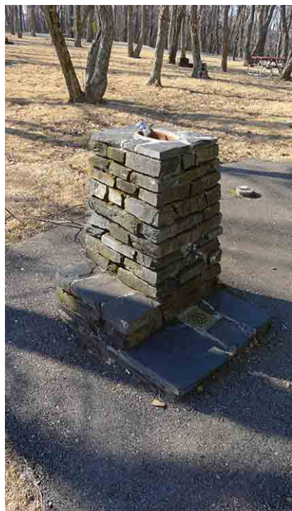
Figure 10. Stone drinking fountain (2014 Rocky Knob Recreation Area CLR, p. 147)
