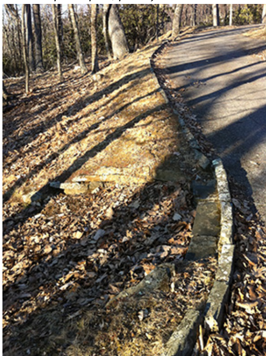
Figure 27. Stone curb in Picnic Area, 2011 (2014 Rocky Knob Recreation Area Cultural Landscape Report, p.150)
