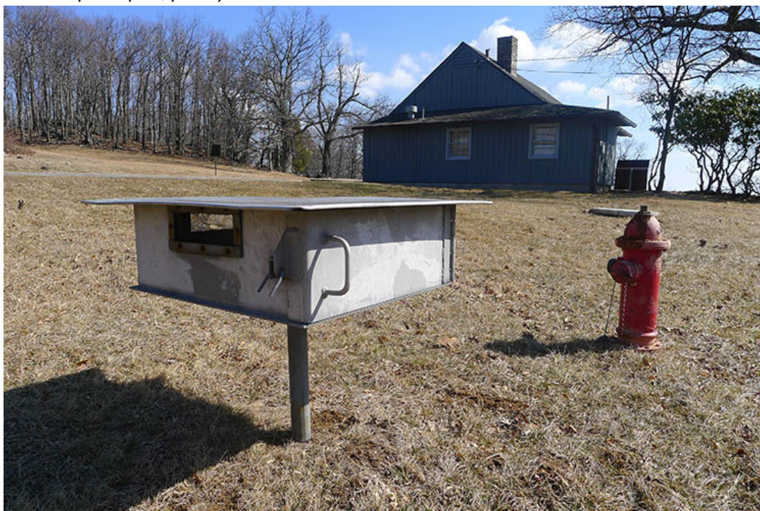
Figure 31. Hose reel and fire hydrant at Gas Station, 2011 (2014 Rocky Knob Recreation Area Cultural Landscape Report, p.157)
