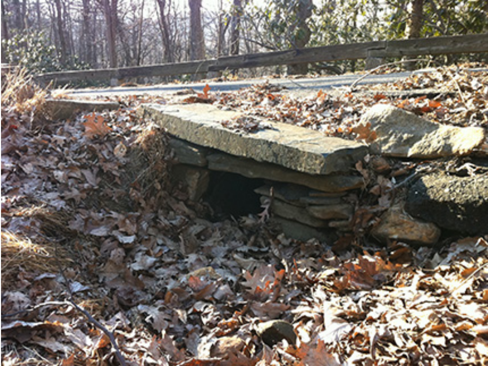
Figure 28. Typical drainage structure in the Picnic Area, 2011 (2014 Rocky Knob Recreation Area Cultural Landscape Report, p.150)
