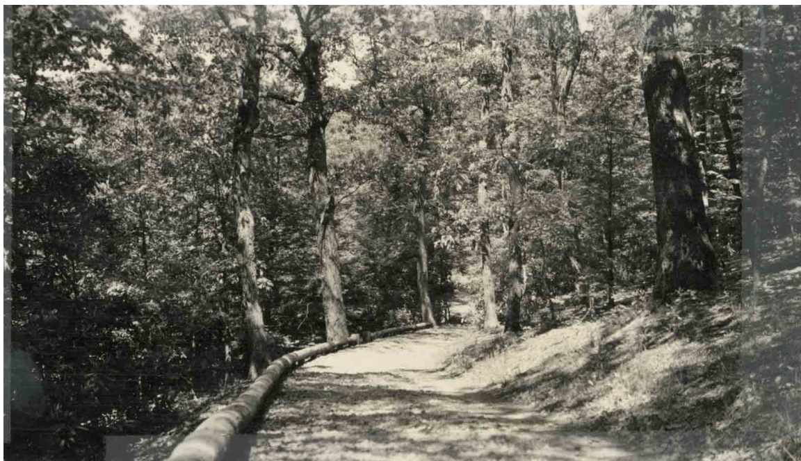
Figure 24. Log guardrail in the Picnic Area, 1938 (2014 Rocky Knob Recreation Area Cultural Landscape Report, p.149)
