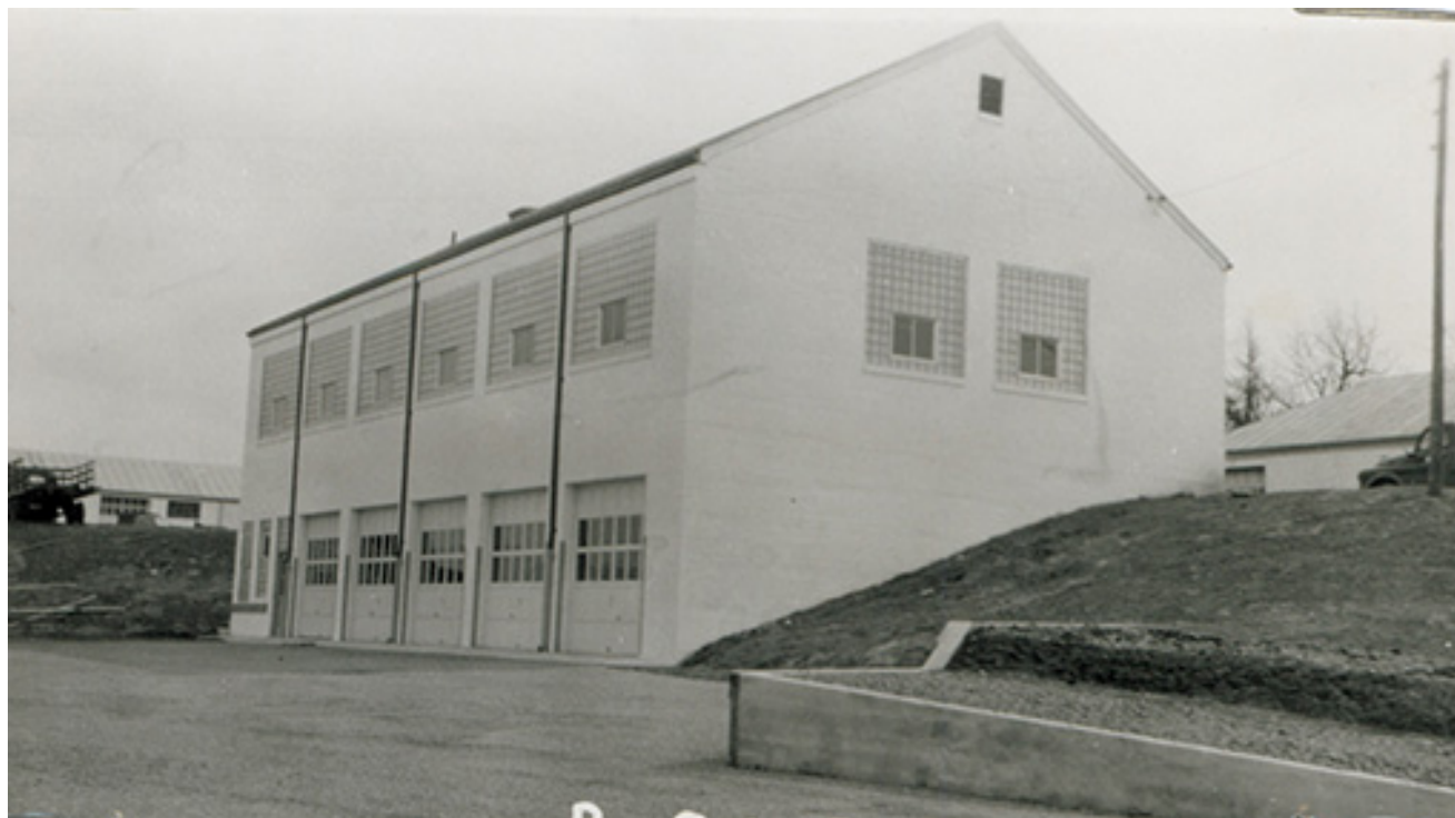
Figure 5a. Upper (top) level of Building #86 after construction. (2014 Rocky Knob Recreation Area CLR, p. 74)
