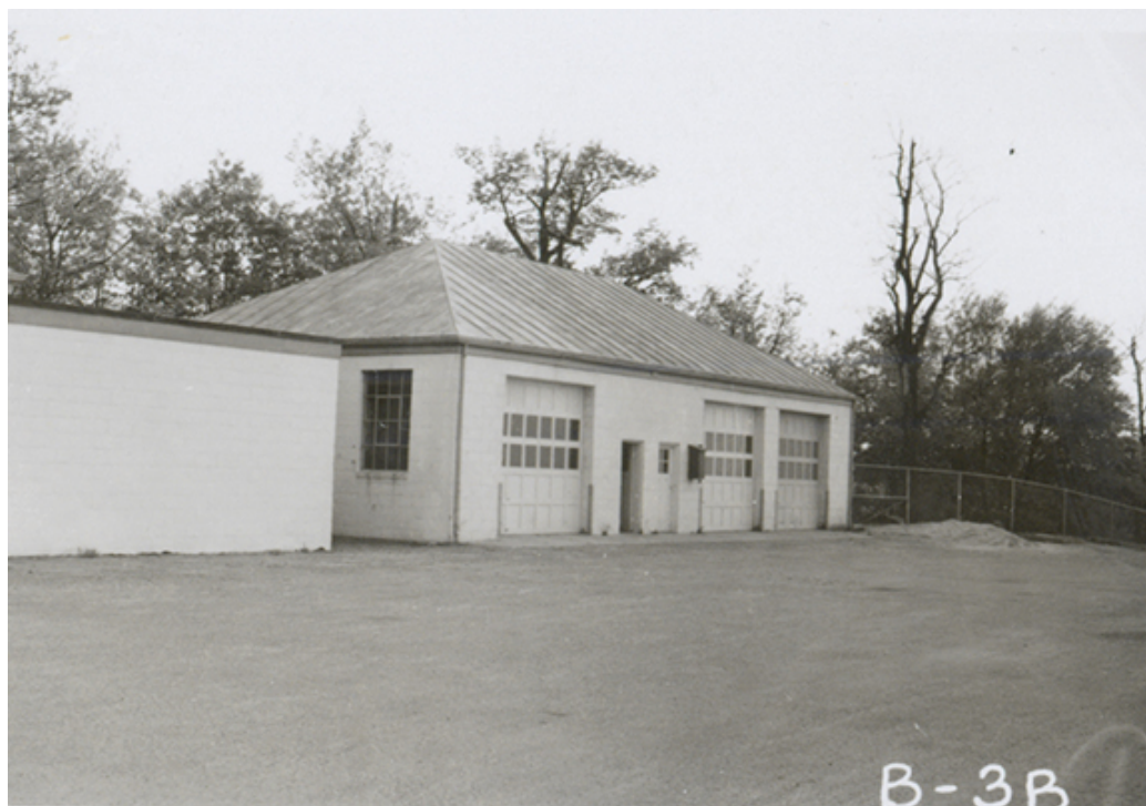
Figure 8. Carpenter and Paint Shop Building #3, c. 1952 (2014 Rocky Knob Recreation Area CLR, p. 132)
