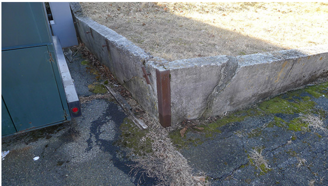
Figure 15. Concrete retaining wall, 2011 (2014 Rocky Knob Recreation Area CLR, p. 138)
