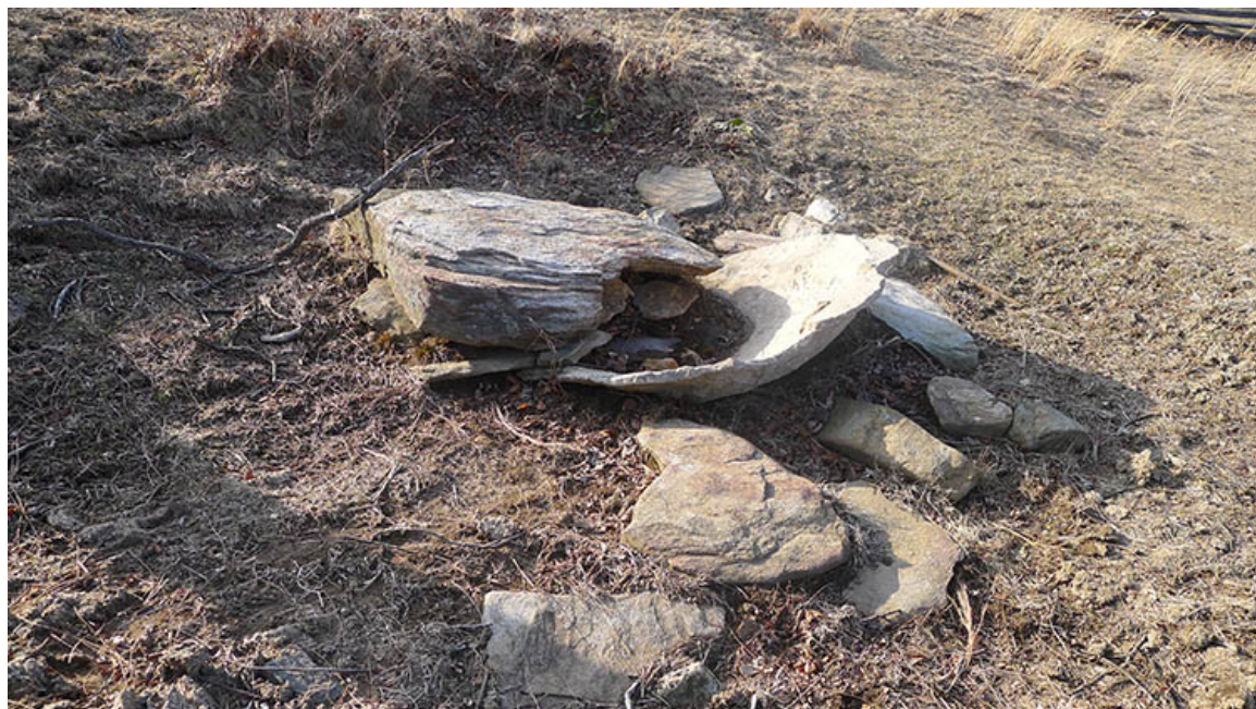
Figure 29. Collapsed spring outlet wall along Parkway Section 1-S near mile 169.6 (2014 Rocky Knob Recreation Area CLR, p. 162)
