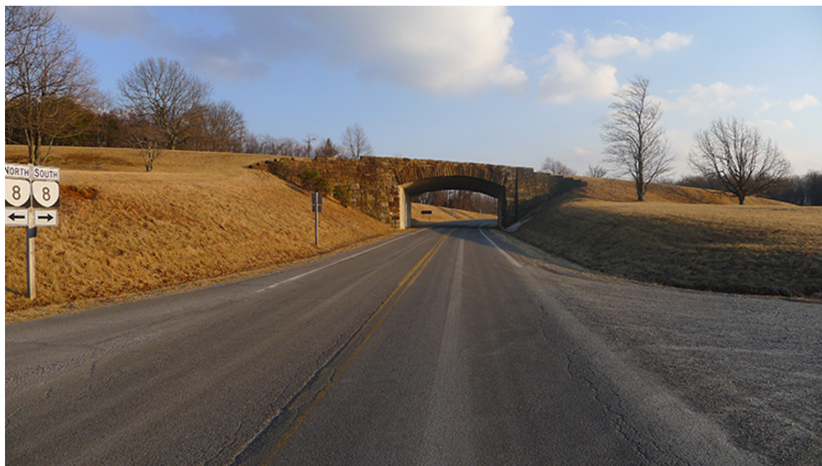
Figure 18. Grade-separated interchange at Tuggle Gap, 2011 (2014 Rocky Knob Recreation Area CLR, p. 159)
