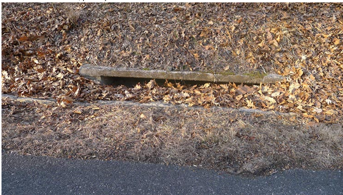
Figure 21. Typical stone headwall along Parkway Section 1-S, 2011 (2014 Rocky Knob Recreation Area CLR, p. 159)
