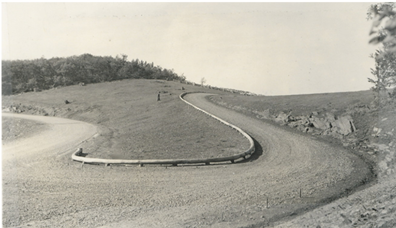
Figure 10. Construction of rubble gutter, c.1938. (2014 Rocky Knob Recreation Area CLR, p. 21)
