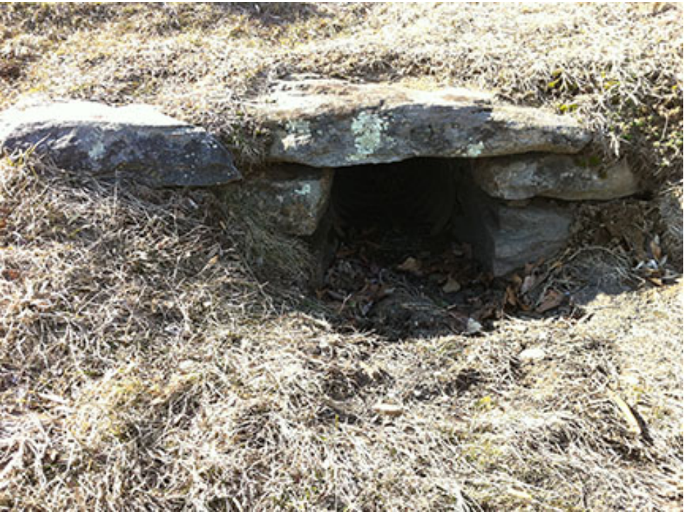
Figure 41. Stone headwall at Twelve O'clock Overlook, 2011 (2014 Rocky Knob Recreation Area CLR, p. 176)
