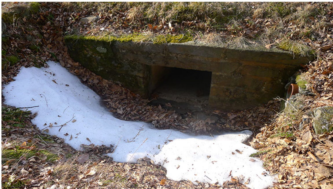
Figure 21. Typical stone headwall along Parkway Section 1-S, 2011 (2014 Rocky Knob Recreation Area CLR, p. 159)
