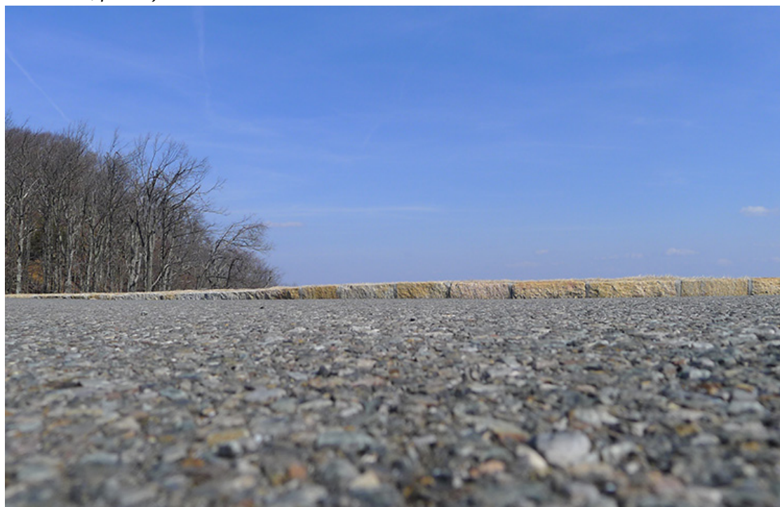
Figure 38. Stone curb transition into grade at Rock Castle Gorge Overlook, 2011 (2014 Rocky Knob Recreation Area CLR, p. 172)
