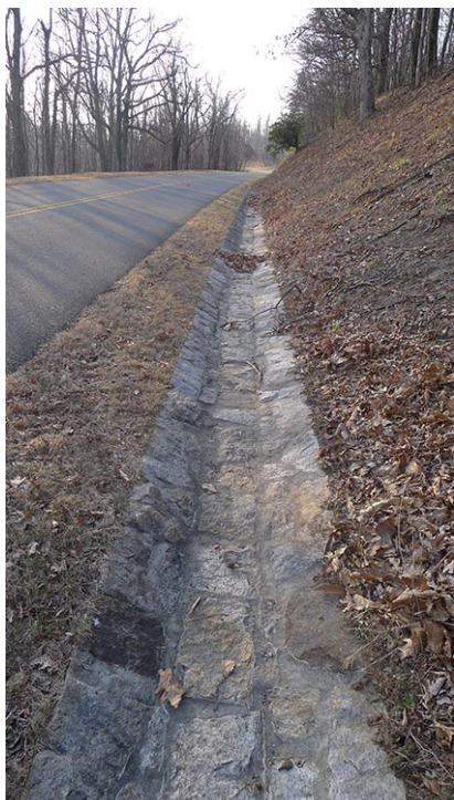
Figure 23. Stone gutter along Parkway Section 1-S, 2011 (2014 Rocky Knob Recreation Area CLR, p. 160)
