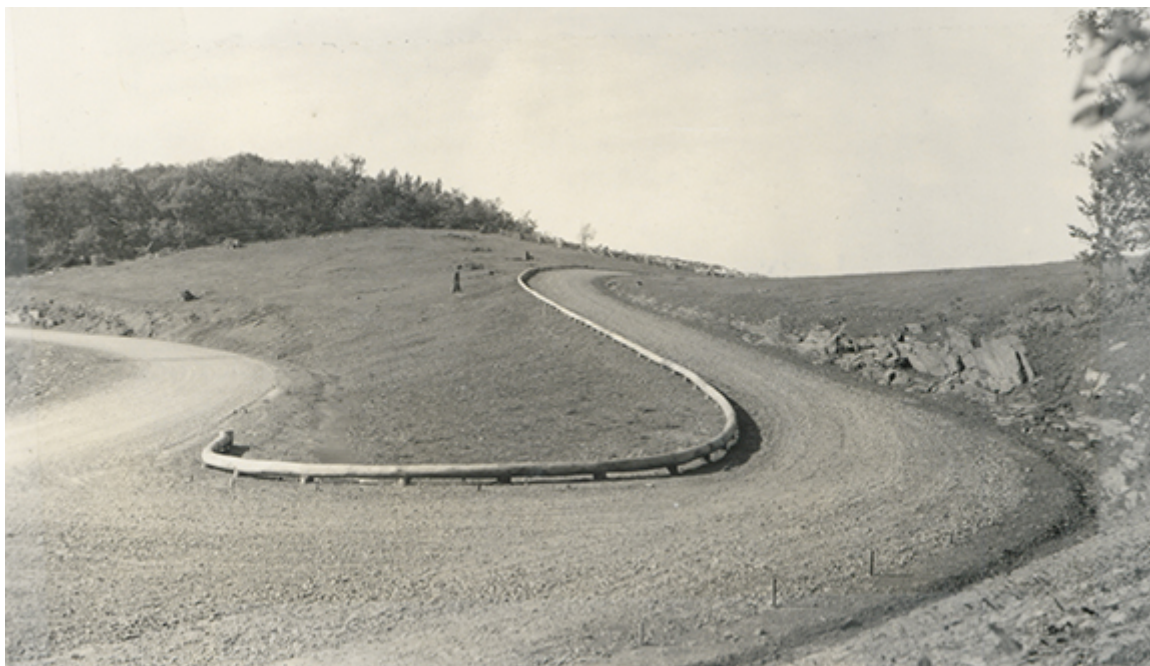
Figure 33. Wooden guardrail at The Saddle Overlook, c. 1938 (2014 Rocky Knob Recreation Area CLR, p. 168)
