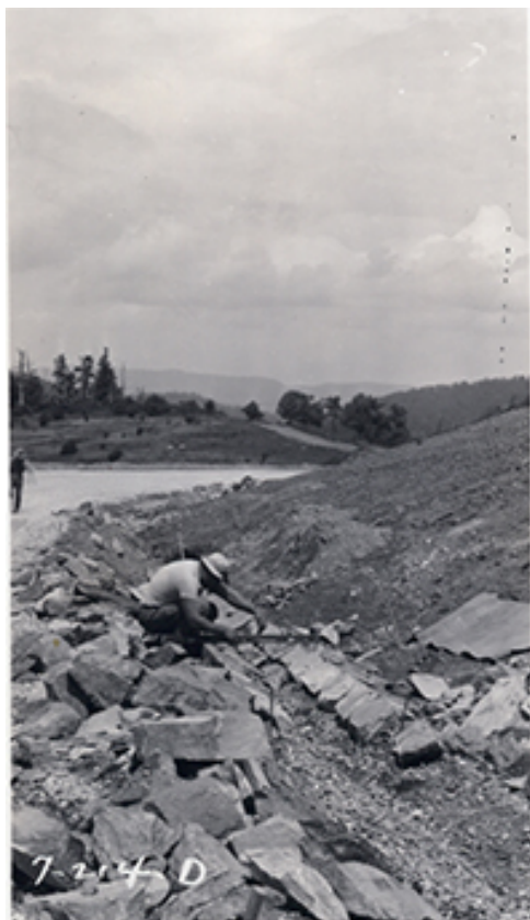
Figure 10. Construction of rubble gutter, c.1938. (2014 Rocky Knob Recreation Area CLR, p. 21)
