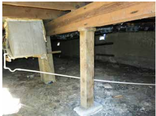
Figure 112. Crawlspace facing northwest. (Source: RATIO Architects, 2020)
