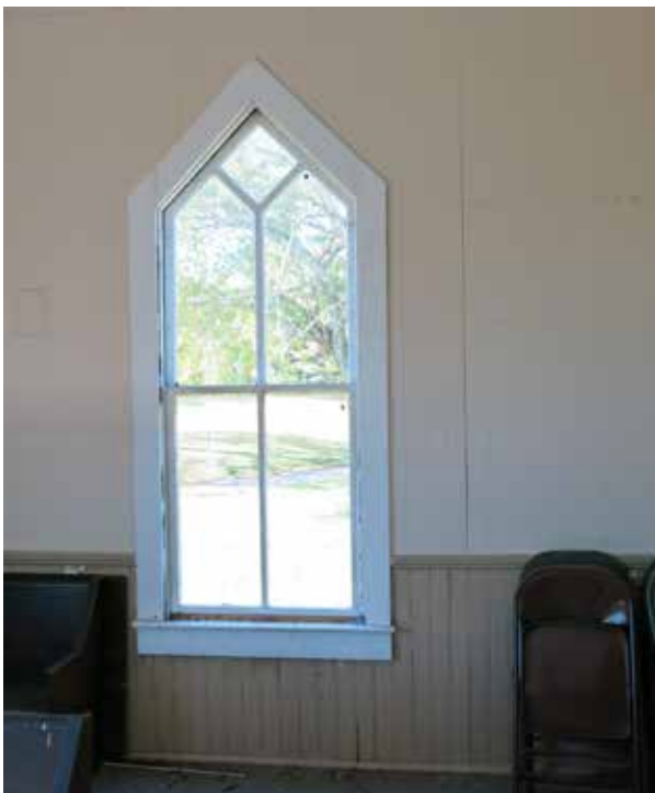
4 Figure 119. Detail of west wall of sanctuary showing 5 typical finishes: bead-board wainscoting, plywood paneling 6 covering flat plaster, and typical window casing. (Source: 7 RATIO Architects, 2020)
