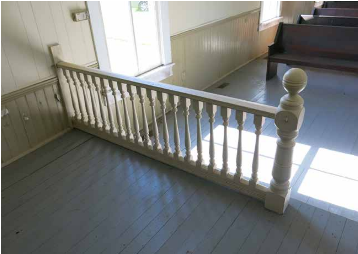
1 Figure 127. Upper (east) face of south section of dais balustrade. Note curtain hardware mounted to newel and wall. (Source: 2 RATIO Architects, 2020)
