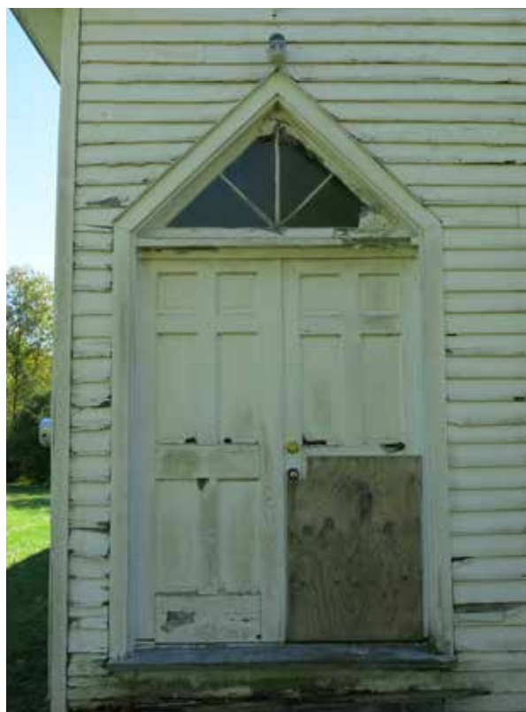
50 Figure 76. Entrance with modern replacement doors 51 installed during 2000-2005 renovation. These doors have a 52 very different appearance from the original horizontal-panel 53 doors. (Source: RATIO Architects, 2020)
