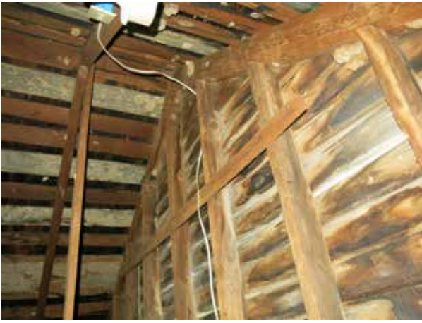
1 Figure 87. View southwest in attic showing back side of 4 2 weatherboard siding at west façade and skip-sheathing at 5 3 roof. (Source: RATIO Architects, 2020) 6 7
