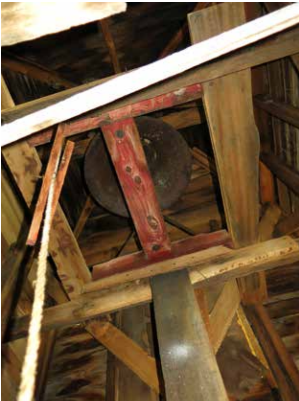
40 Figure 135. View into cupola from attic, facing north. 41 (Source: RATIO Architects, 2020)
