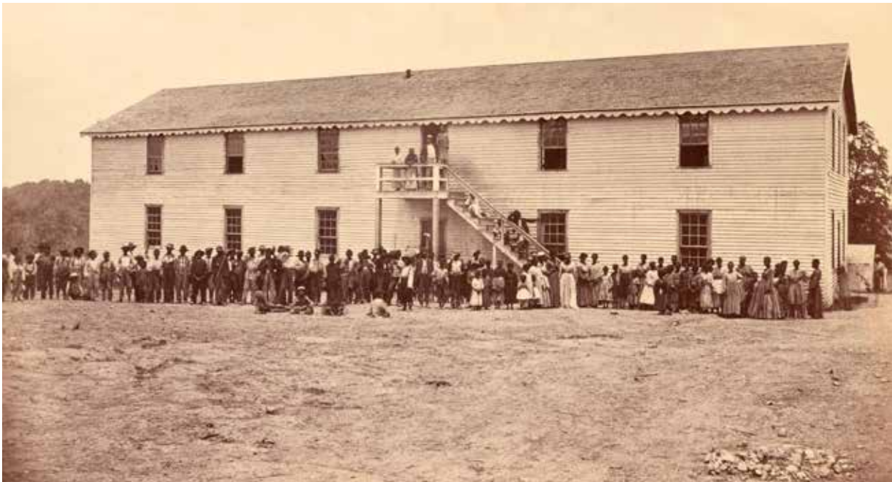
9 Figure 11. Refugees at the School House (Building 78) at the National Home for Colored Refugees, 1865. This photograph 10 shows the southwest and southeast elevations of the building that was built to house the school founded by John Fee in 1864. 11 The man at the top of the stairs might be John Fee or Rev. Abishai Scofield or he may be a refugee. The photographer is in a 12 similar position to Figure 10, where the camera is rotated approximately ninety degrees to the right from this view. (Source: 13 National Archives, Still Picture Branch, Washington, D.C.; G. W. Foster and Co., photographers)
