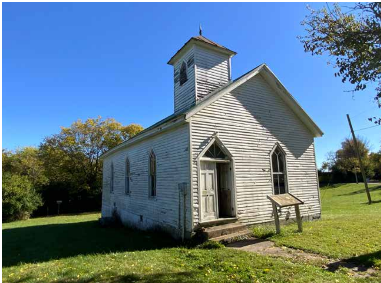
42 Figure 63. North elevation and west façade, facing southeast. Note modern siding covering west face of cupola where a 43 louvered opening was formerly present. (Source: RATIO Architects, 2020)
