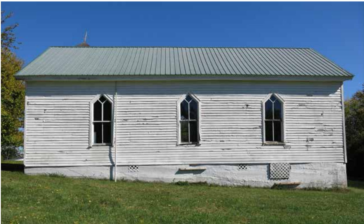
2 Figure 67. South elevation, facing north. (Source: RATIO Architects, 2020)
