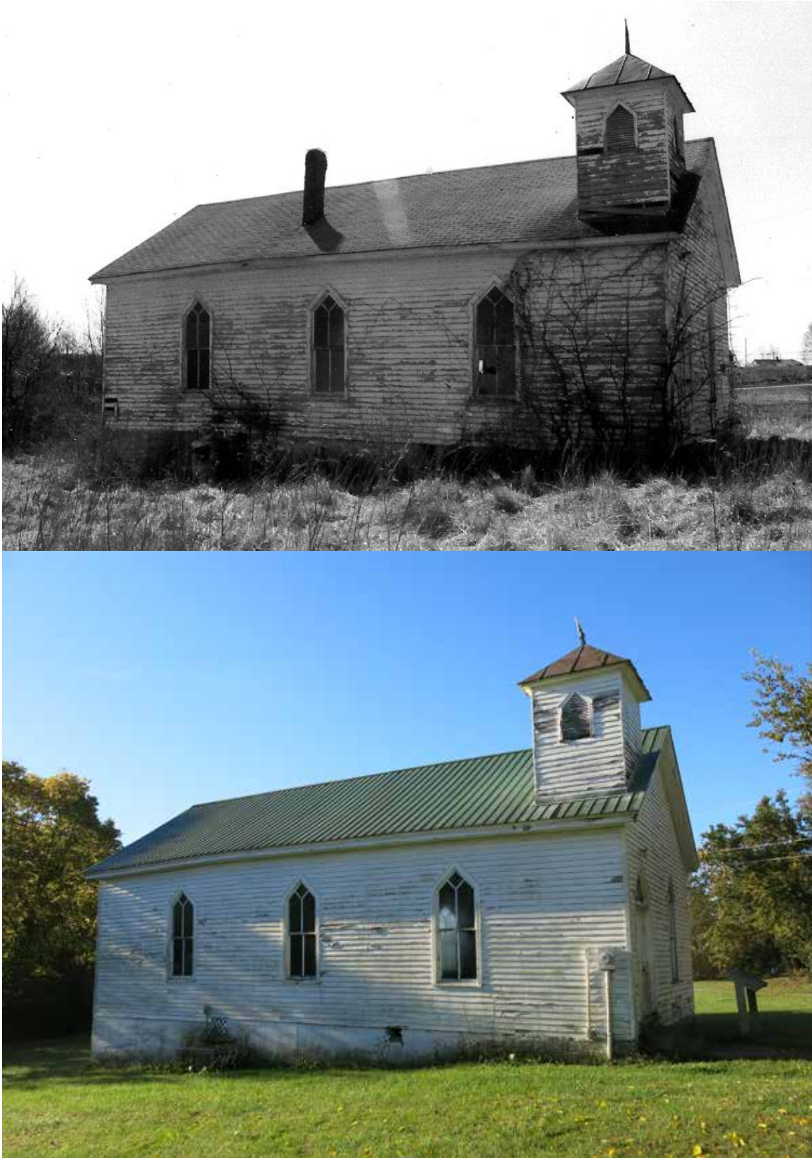
1 Figure 53. North elevation and west façade of Fee Memorial Church, ca. 1994-2000. This shows the deteriorated condition of 2 the church prior to the Jessamine County renovation. (Source: Camp Nelson Civil War District National Register nomination) 3 Similar view of the north elevation and west façade in 2020. (Source: RATIO Architects)
