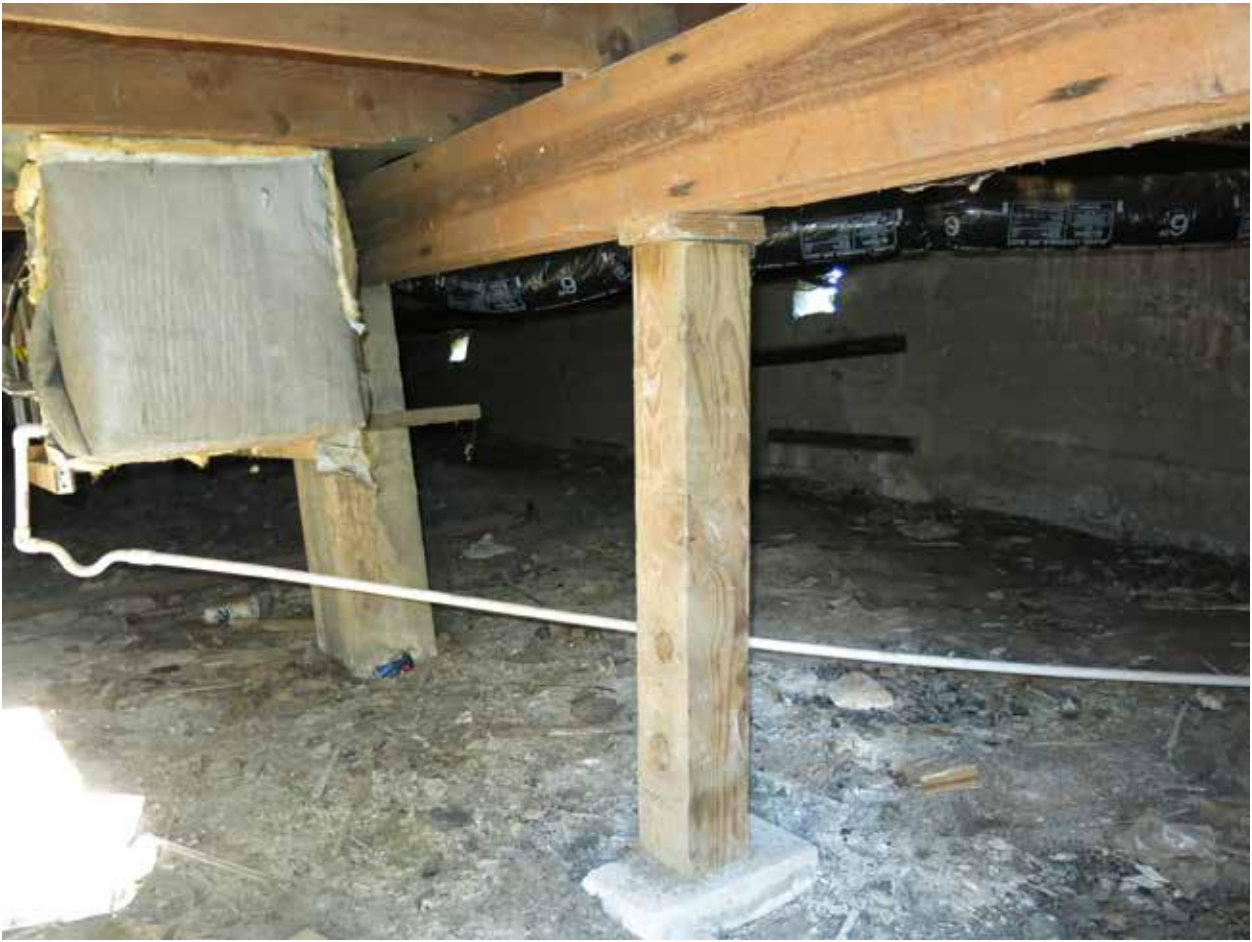
1 Figure 96. Crawlspace facing northwest, showing central beam. (Source: RATIO Architects, 2020)
