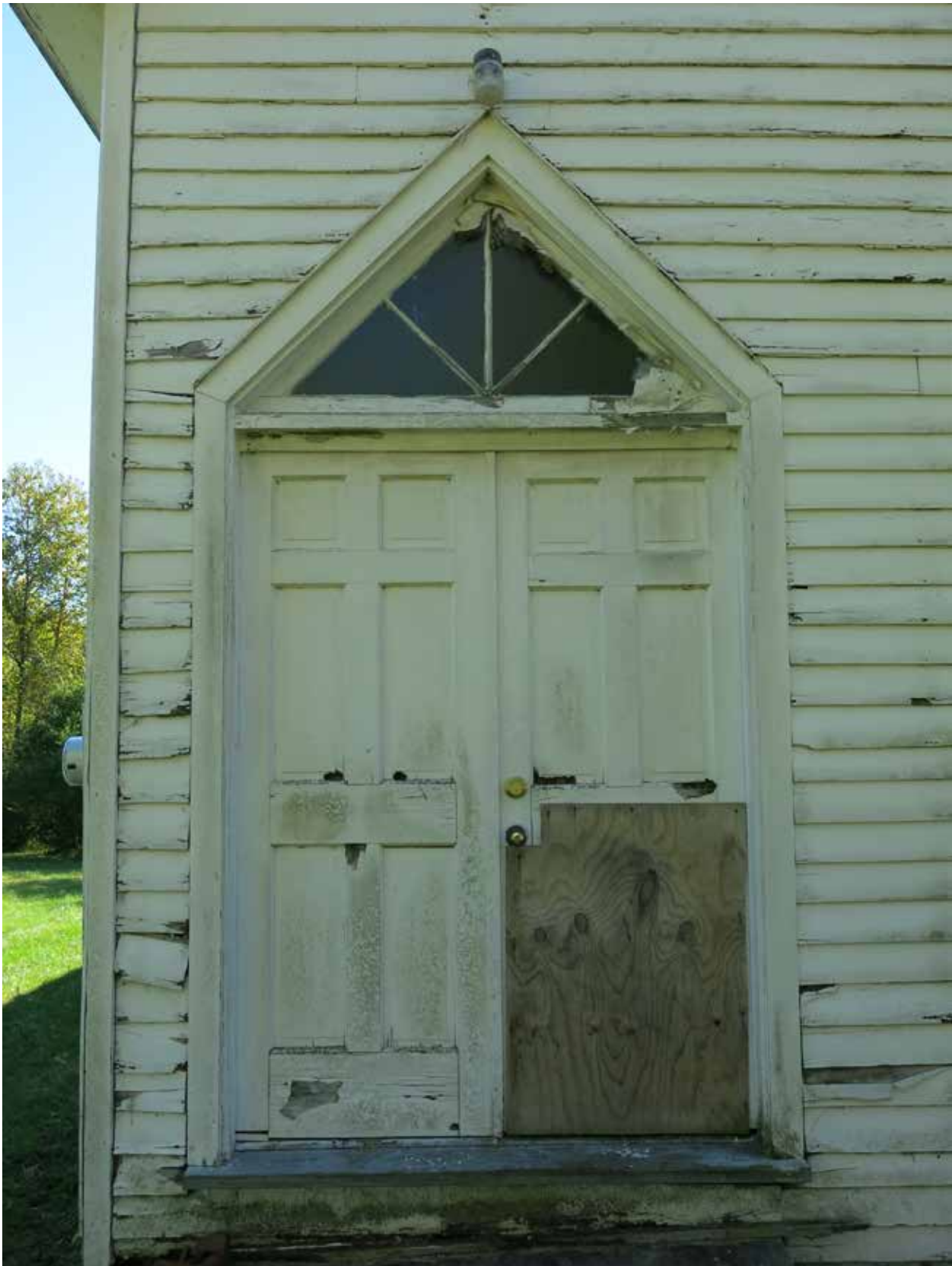
1 Figure 82. Entrance with modern replacement doors installed during 2000-2005 renovation. These doors have a very different 2 appearance from the original horizontal-panel doors. (Source: RATIO Architects, 2020)
