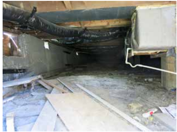
Figure 111. Crawlspace looking west. (Source: RATIO Architects, 2020)
