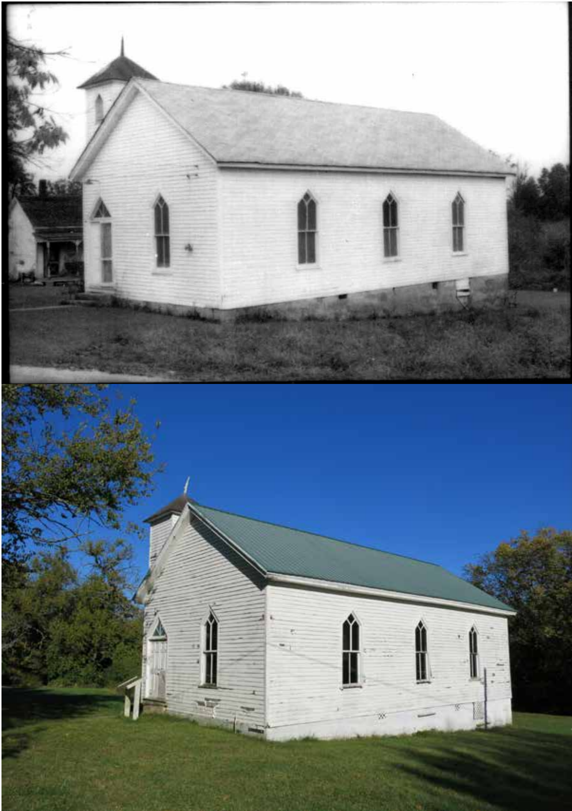
1 Figure 47. (Top) West façade and south elevation of Fee Memorial Church, summer 1977. These are the earliest photographs 2 of the church located to date and they appear to show the building largely as built in 1912. Note the entry doors and louvers 3 on the face of the cupola, all now missing. The south chimney had been removed before this photograph was taken. Note 4 also manse at left. (Source: Kentucky Historic Resources Inventory, JS56. Reprinted with permission from the Kentucky Heritage 5 Council) Bottom photo is a similar view from October 2020 (Source: RATIO Architects)
