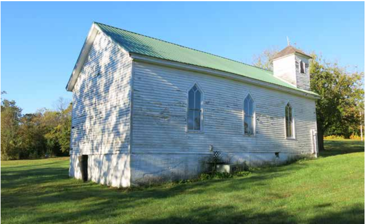
2 Figure 69. East and north elevations, facing southwest. (Source: RATIO Architects, 2020)
