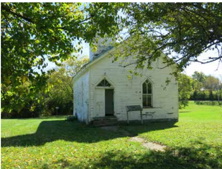
Figure 59. Immediate context of Fee Memorial Church showing partially exposed concrete walkway, uneven steps, and wayside interpretive sign. (Source: RATIO Architects, 2020)
