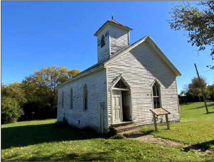
Photo 1 – View of the west side of the church at the front.
