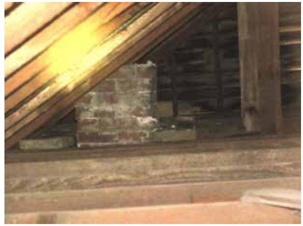
Figure 102. View east in attic showing base of north chimney and back of siding at east elevation. (Source: RATIO Architects, 2020)
