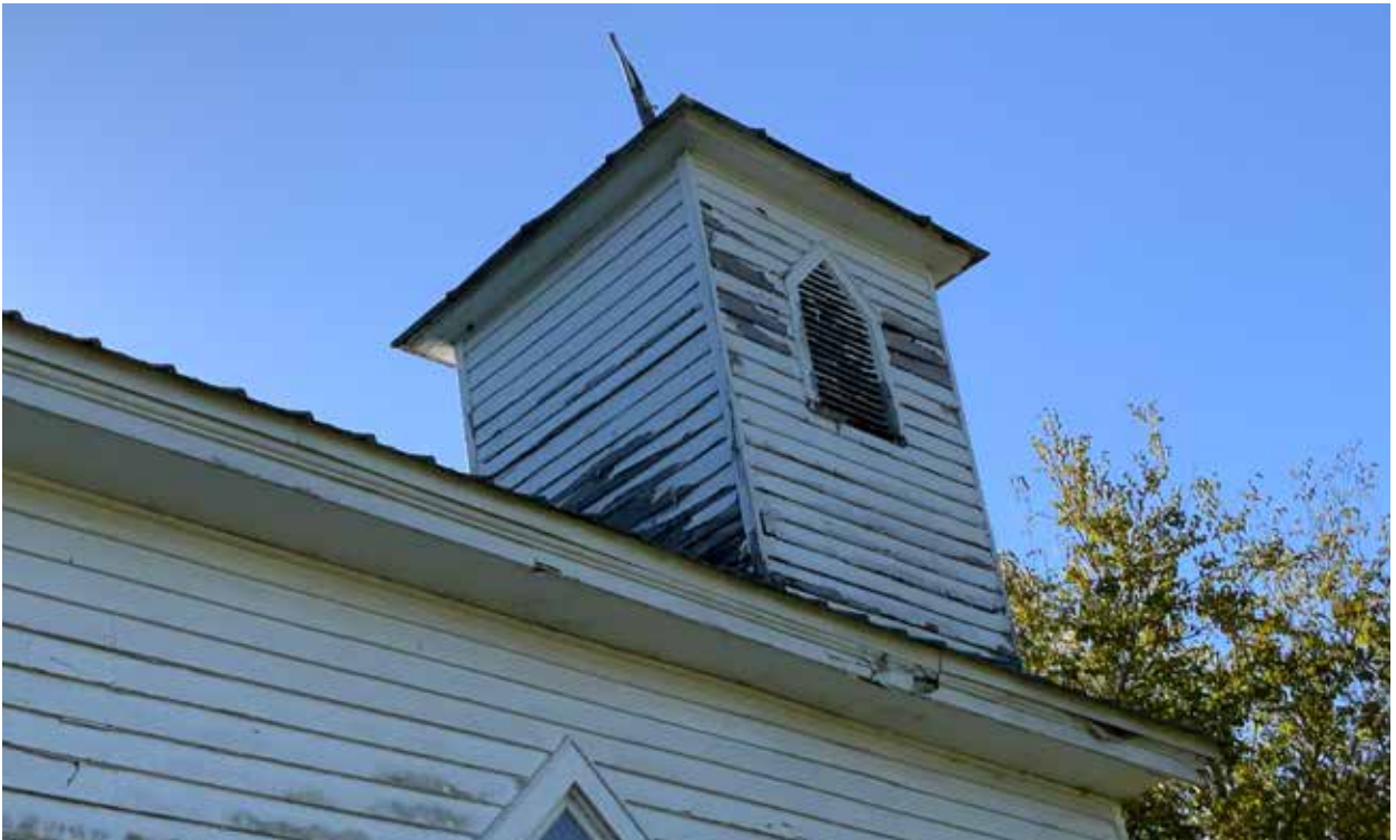
2 Figure 65. Detail of east and north elevations of cupola, facing southwest. (Source: RATIO Architects, 2020)
