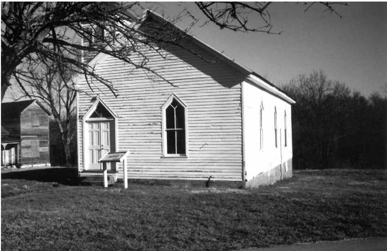
4 Figure 55. West façade and south elevation of Fee Memorial Church, ca. 2000-2005. This appears to show the building near 5 the end of the Jessamine County renovation. Note modern replacement doors on church, west louvers of cupola, and manse in 6 distance at left. (Source: W. Stephen McBride)
