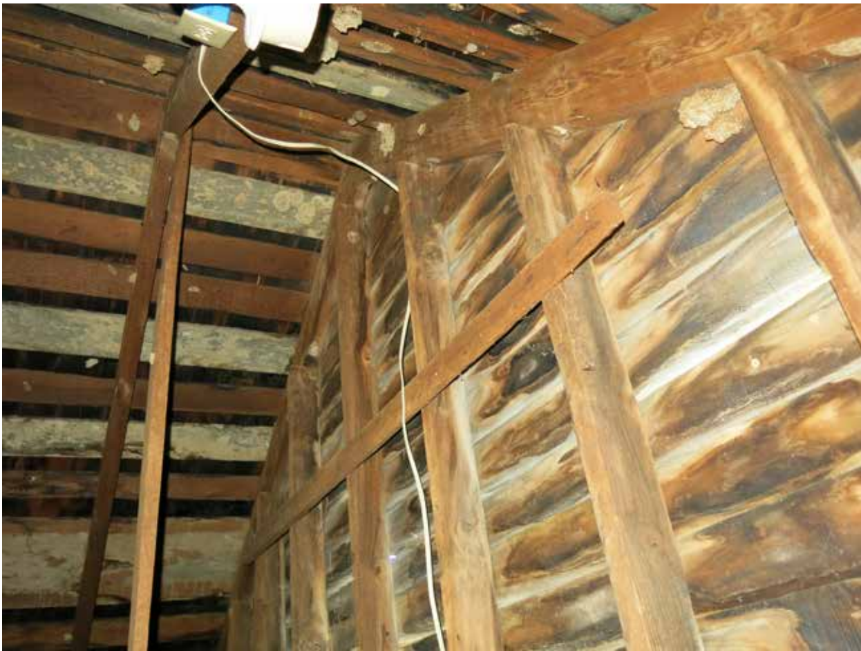
1 Figure 100. View southwest in attic showing roof framing. (Source: RATIO Architects, 2020)
