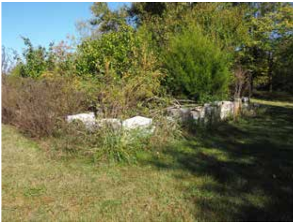
Figure 34. View of manse foundation from the southeast showing overgrowth. The stone foundation survives but is currently obscured by overgrowth. (Source: RATIO Architects, 2020)
