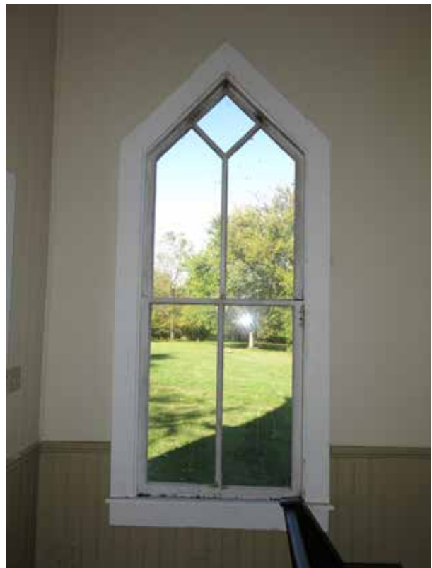
Figure 74. Typical interior face and trim of windows; west window of north elevation, facing north. (Source: RATIO Architects, 2020)
