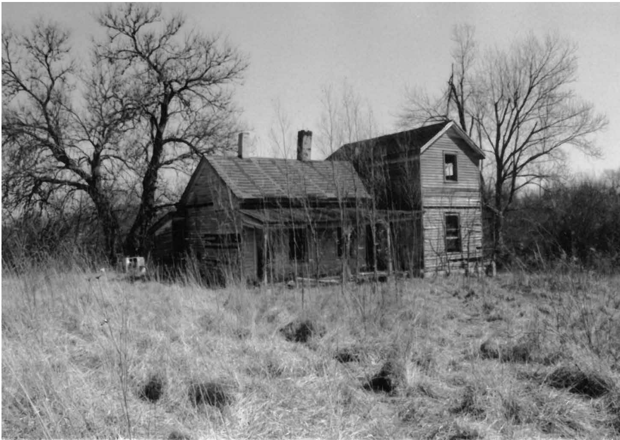
Figure 32. View of manse/parsonage, facing northeast, ca. 1994-2000. The photographer is standing near the entrance to the Fee Memorial Church. This house was built between about 1890-1910 and housed the ministers of the Fee Memorial Church. It was demolished around 2007. (Source: W. Stephen McBride)
