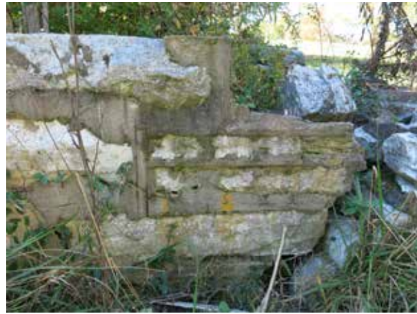
Figure 35. Detail of manse foundation at north part of east elevation. Note raised mortar joints at right; rough joints at left were concealed by the porch floor. (Source: RATIO Architects, 2020)
