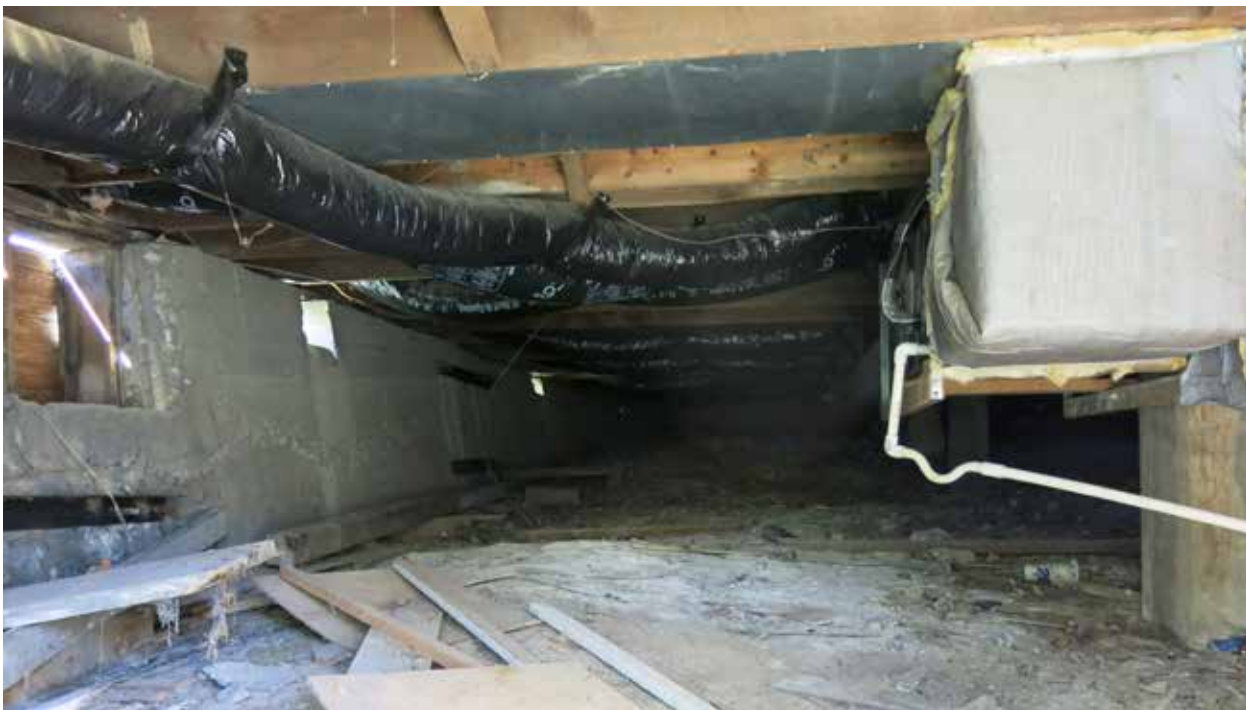
Figure 95. Crawlspace looking west, showing joists. (Source: RATIO Architects, 2020)
