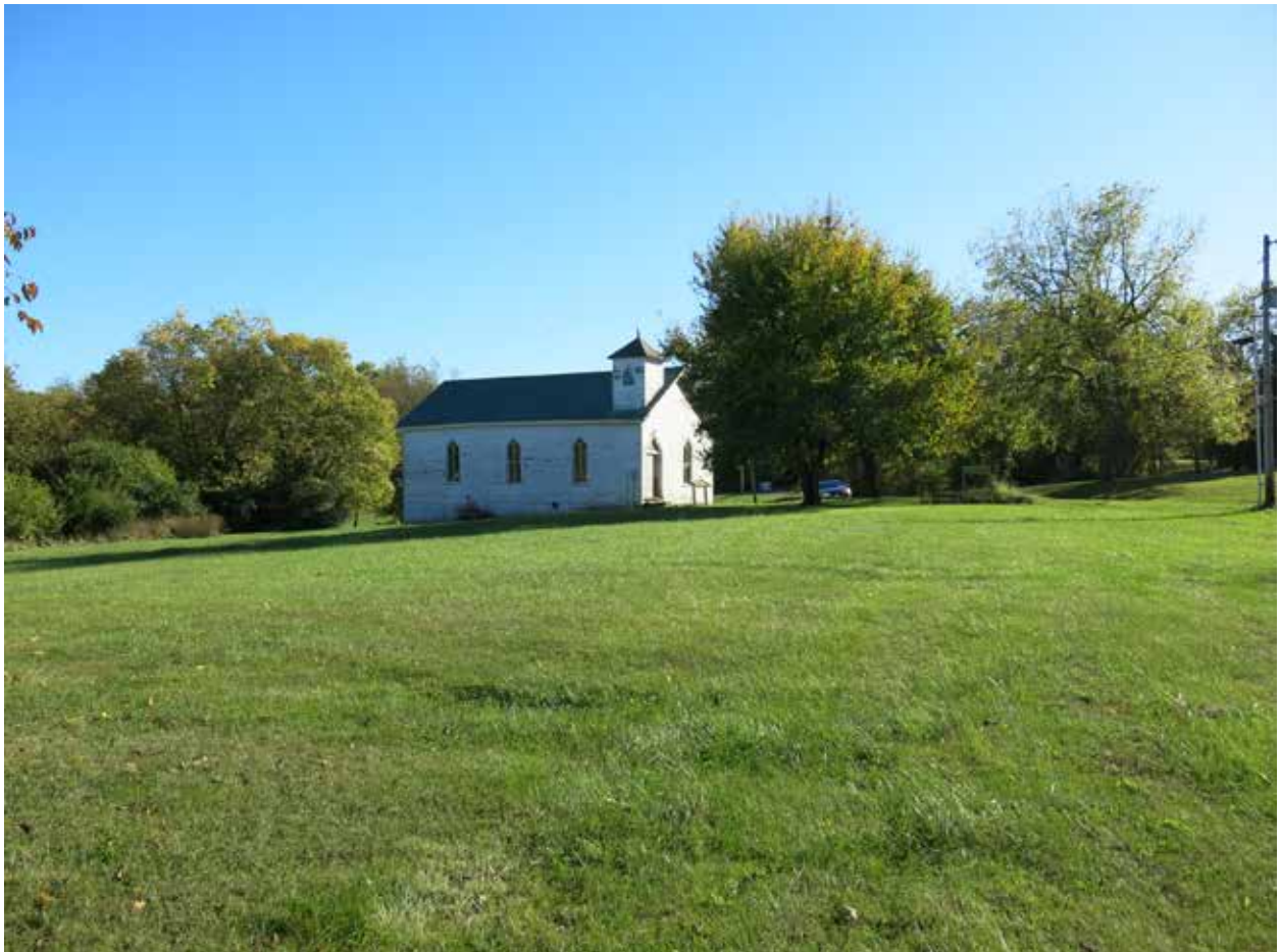
Figure 56. Fee Memorial Church from apparent site of dormitory, facing southeast; overgrown manse foundation is at left. (Source: RATIO Architects, 2020)
