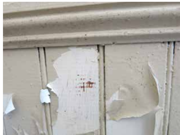
2 Figure 120. Detail of wainscot at south wall showing 3 underlying finish layers. (Source: RATIO Architects, 2020)
