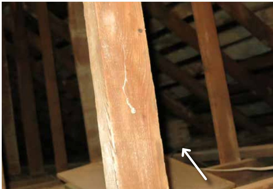
Figure 93. View southeast within attic. The studs in the foreground define the south wall of the vestibule; The base of the south chimney is visible at center right. (Source: RATIO Architects, 2020)
