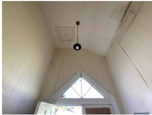
Figure 114. Upper part of vestibule, facing west. Note attic hatch, bell-rope, and pendant fixture. (Source: RATIO Architects, 2020)
