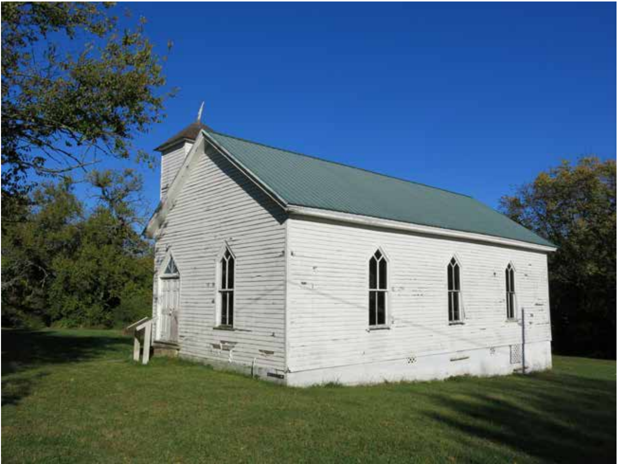
1 Figure 64. West façade and south elevation, facing northeast. (Source: RATIO Architects, 2020)
