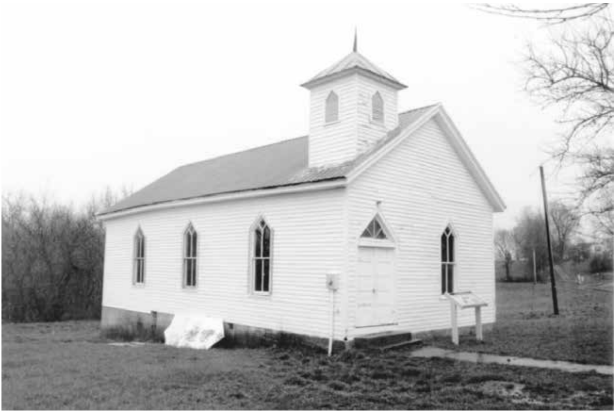
1 Figure 54. North elevation and west façade of Fee Memorial Church, ca.2000. This appears to document the exterior during 2 the Jessamine County renovation. Note louver on west face of cupola and horizontal-panel front doors. (Source: Camp Nelson 3 Civil War District National Register nomination) See Figure 46 for a similar view in 2020.
