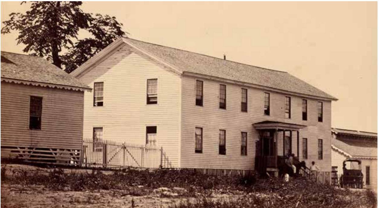
6 Figure 9. View of the Head Dormitory (Building 75) of the National Home for Colored Refugees, facing north, 1865. The 7 buildings at right and left are two of the wards (Buildings 74) and may be the “wings” mentioned at the time the Head 8 Dormitory was purchased for Ariel Academy in 1868. These buildings formed the original facilities of Ariel Academy. (Source: 9 National Archives, Still Picture Branch, Washington, D.C.; G. W. Foster and Co., photographers)
