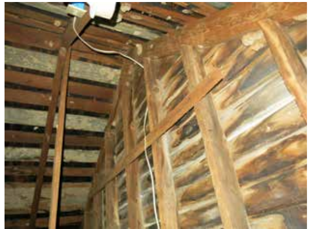
31 Figure 131. View southwest in attic showing back side of 32 weatherboard siding at west façade and skip-sheathing at 33 roof. (Source: RATIO Architects, 2020)
