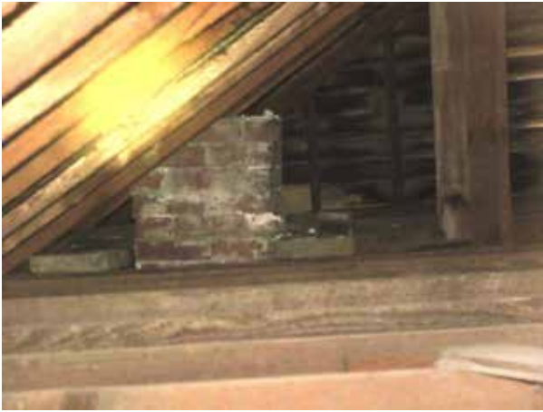
1 Figure 133. View east in attic showing base of north 2 chimney and back of siding at east elevation. (Source: RATIO 3 Architects, 2020)
