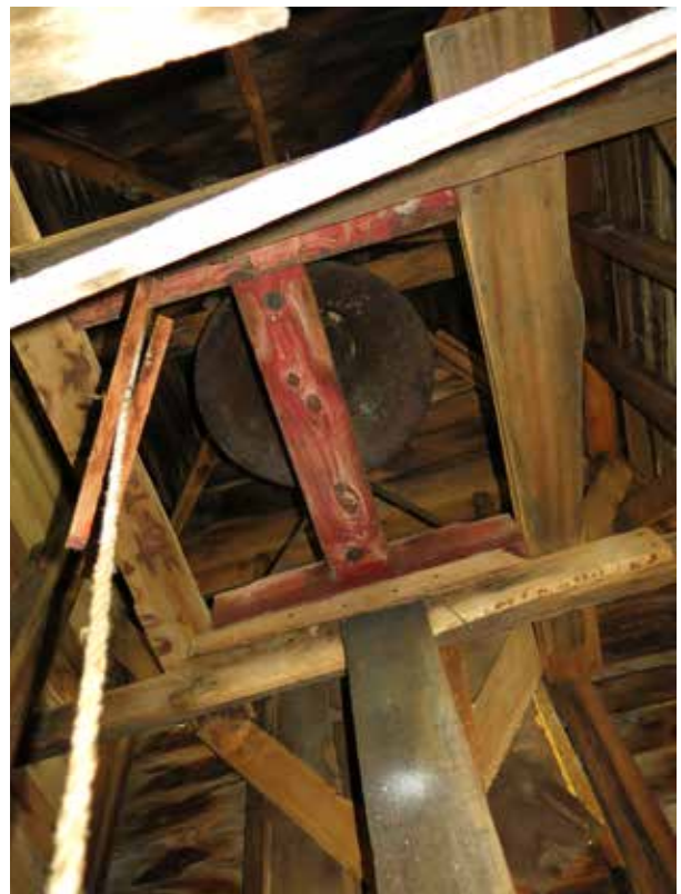
Figure 103. View into cupola from attic, facing north. (Source: RATIO Architects, 2020)
