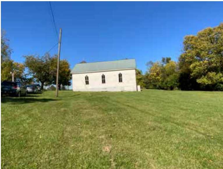
Figure 57. Fee Memorial Church and context from the south, facing north. (Source: RATIO Architects, 2020)
