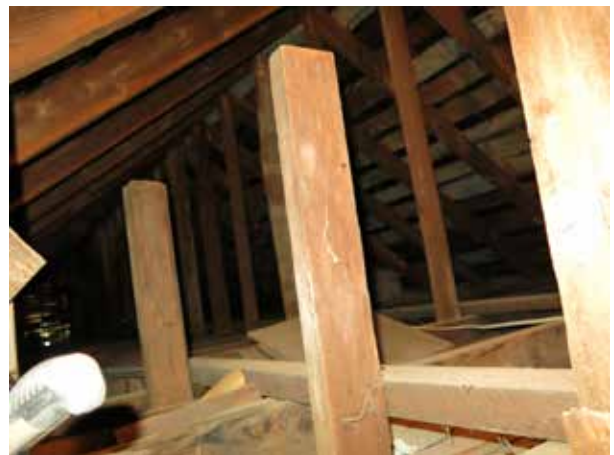
34 Figure 132. View southeast within attic. The studs in the 35 foreground define the south wall of the vestibule. The base 36 of the south chimney is visible at center right. (Source: RATIO 37 Architects, 2020)
