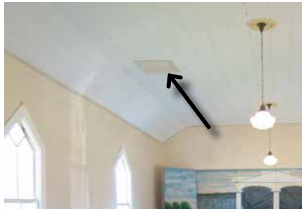
Figure 92. Sanctuary, facing east. Note patch at underside of north chimney at upper left. (Source: RATIO Architects, 2020)
