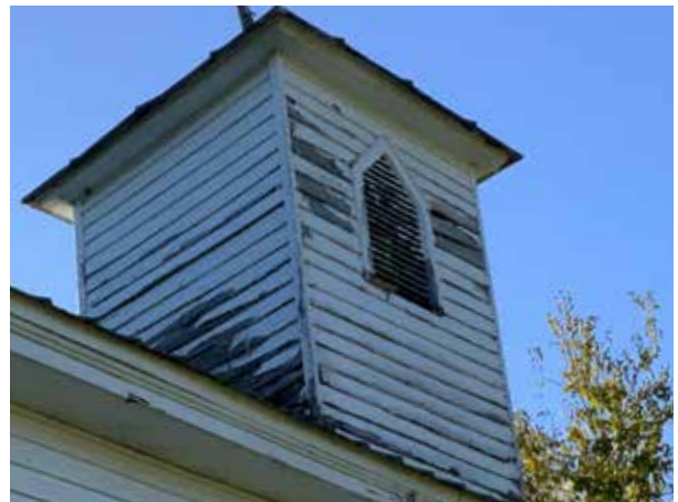
11 Figure 80. Detail of east and north elevations of cupola, 12 facing southwest. (Source: RATIO Architects, 2020)
