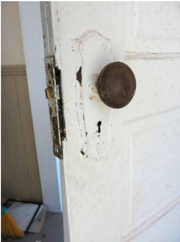
1 Figure 85. Detail of hardware at vestibule door. (Source: 2 RATIO Architects, 2020)
