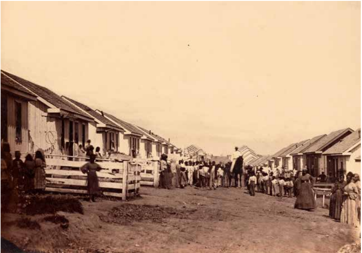
Figure 12. View northwest along the south street of double cottages (Buildings 85) at the National Home for Colored Refugees, 1865. These cottages were built to provide refugees with sanitary housing and were designed better support the maintenance of family units. This street became Row Street when the village of Ariel was laid out in 1868. The camera appears to be placed near the present curve of Church Street (formerly the intersection of Front and Row Streets), in a similar position and orientation to Figure 37. (Source: National Archives, Still Picture Branch, Washington, D.C.; G. W. Foster and Co., photographers)
