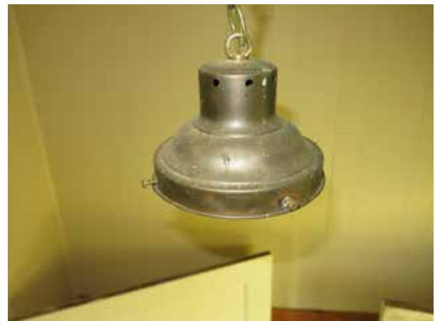
Figure 108. Detail of shade holder of vestibule pendant showing later chain of dissimilar finish. (Source: RATIO Architects, 2020)
