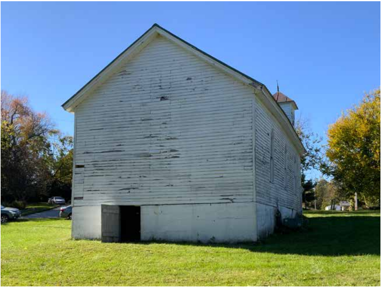
1 Figure 68. East and north elevations, facing southwest. (Source: RATIO Architects, 2020)
