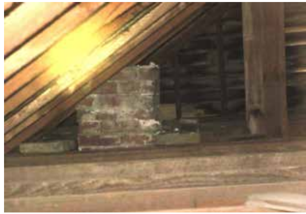
Figure 91. View east in attic showing base of north chimney and back of siding at east elevation. (Source: RATIO Architects, 2020)
