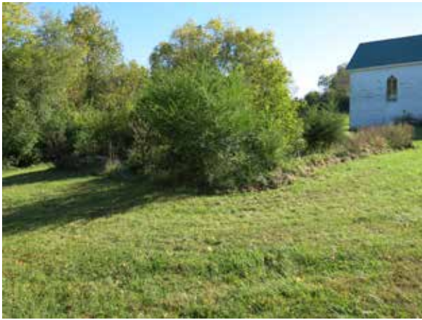
Figure 36. View of manse foundation from the northwest showing overgrowth, with Fee Memorial Church at right. (Source: RATIO Architects, 2020)
