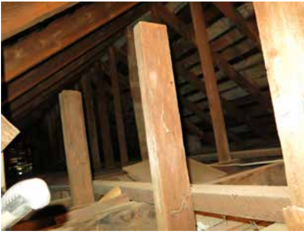
Figure 101. View southeast within attic. The studs in the foreground define the south wall of the vestibule. The base of the south chimney is visible at center right. (Source: RATIO Architects, 2020)
