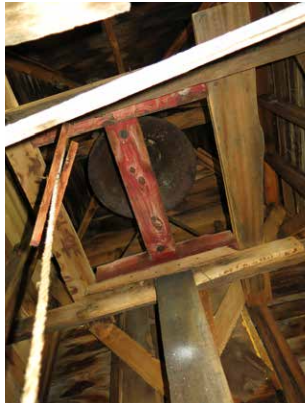
12 Figure 90. View into cupola from attic, facing north. (Source: 4 13 RATIO Architects, 2020) 5
