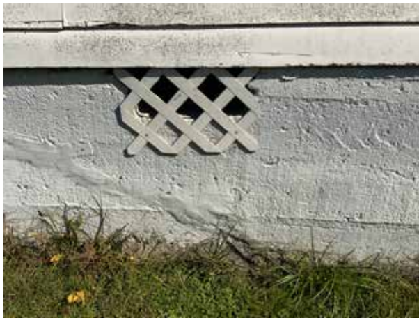
Figure 70. Detail of board-formed concrete foundation at south elevation showing typical exterior surface and modern lattice applied over crawlspace vents. (Source: RATIO Architects, 2020)
