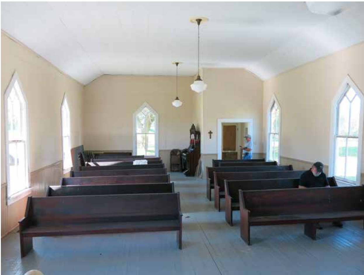
1 Figure 118. Sanctuary, facing west. Note stovepipe opening for south chimney at upper right. (Source: RATIO Architects, 2020)
