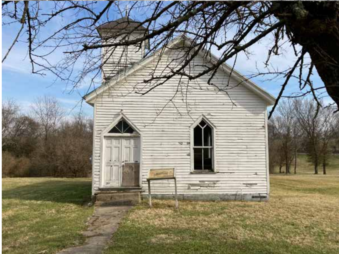
1 Figure 48. (Top) West façade of Fee Memorial Church, ca. 1994-2000. This shows the deteriorated condition of the church prior 2 to the Jessamine County renovation. Note louver on west face of cupola and horizontal-panel front doors. (Source: W. Stephen 3 McBride) March 2021 photo of a similar view (Source: WLA Studio)
