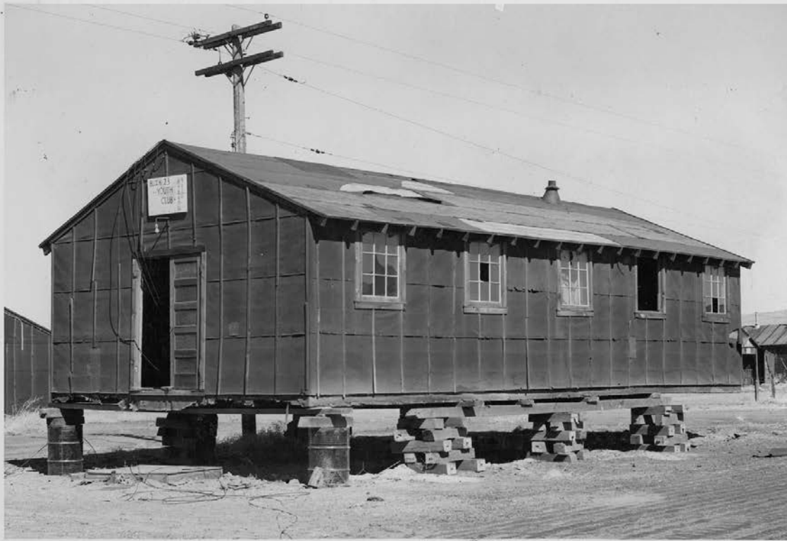
KP-1377-R2 - Klamath Project. Buildings at Newell. One method of removing barracks from the old Jap Camp at Newell is to set the building up on blocks, cut it into sections and carry it away on a truck. This building has just been set up on blocks preparatory to hauling it away in sections. J. E. Fluharty, Photo. March 15, 1947.
