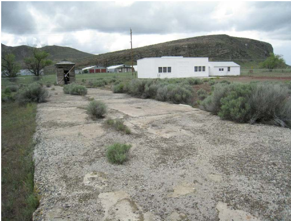
Archeological Sites #4: Foundation slab of building 75, TULE 2004 A-130, looking west (PWR Cultural Landscapes Program, 2015).
