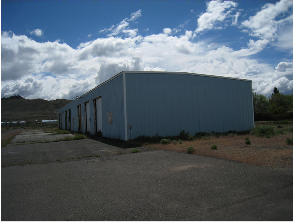
Buildings and Structures #3: Building 104, view to southwest (PWR Cultural Landscapes Program, 2015).
