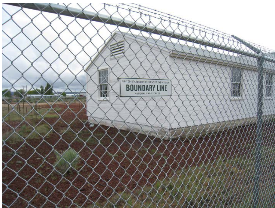
Small Scale Features #10: Non-Contributing fence between Post Engineer's Yard and Highway 139, looking from highway to the east (PWR Cultural Landscapes Program, 2015).
