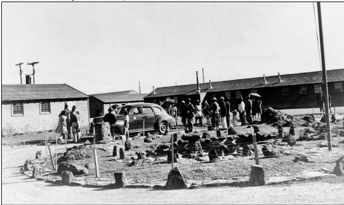
History #17: A rock garden near the flagpole at the Tule Lake Segregation Center, 1943 (Library of Congress, Prints & Photographs Division, FSA/OWI Collection, [LC-USZ62-132041]).
