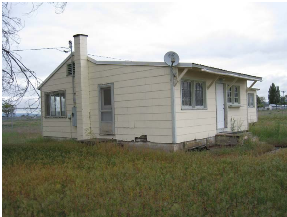
Buildings and Structures #8: Ditch Rider House, view to north (PWR Cultural Landscapes Program, 2015).
