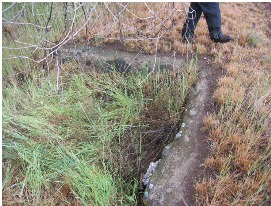
Small Scale Features #6: Culvert headwall at Highway 139 (PWR Cultural Landscapes Program, 2015).
