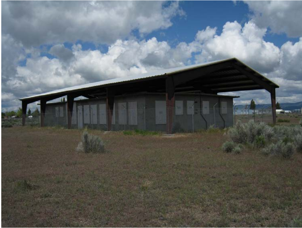
Buildings and Structures #1: Jail, view to north (PWR Cultural Landscapes Program, 2015).
