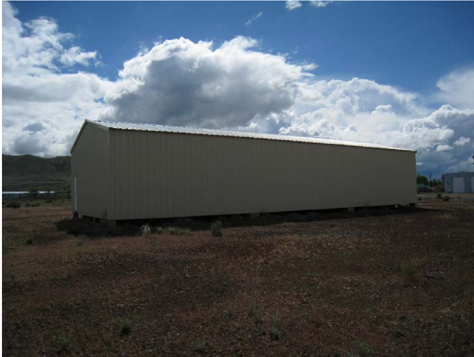
Buildings and Structures #4: Building 208, view to southwest (PWR Cultural Landscapes Program, 2015).
