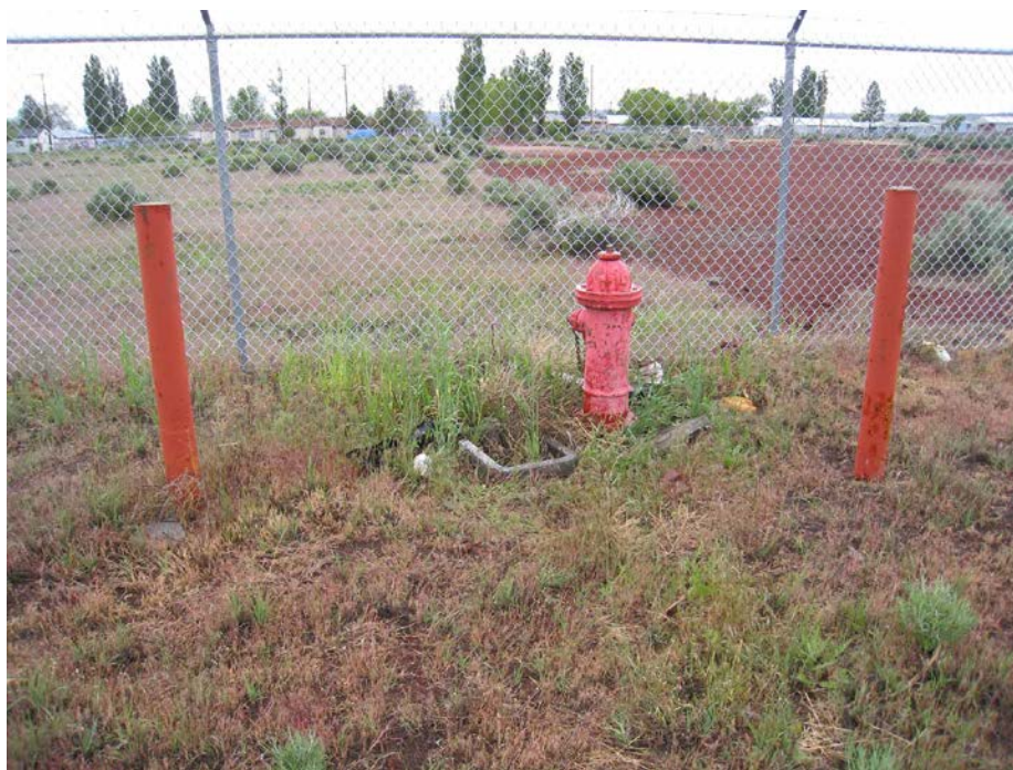
Small Scale Features #5: One of two fire hydrants on site (PWR Cultural Landscapes Program, 2015).
