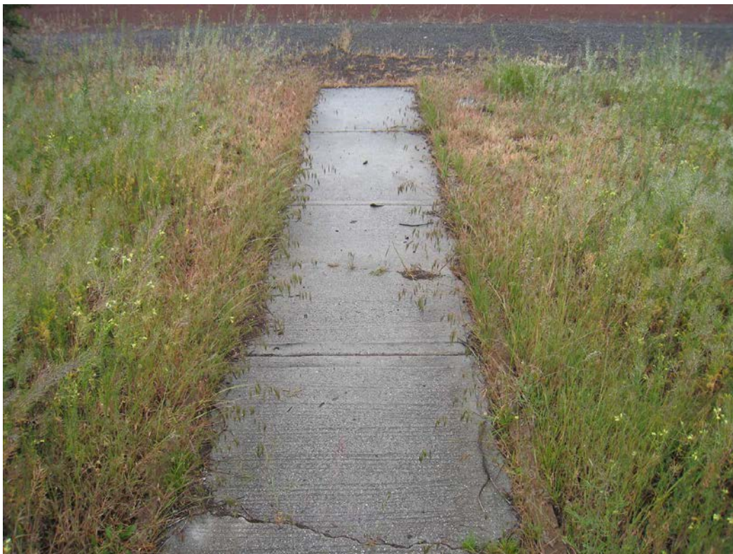
Circulation #4: Sidewalk of Residence, Ditch Rider House, TULE 2004 A-127 looking southeast from house (PWR Cultural Landscapes Program, 2015).
