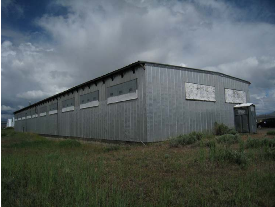
Buildings and Structures #2: Building 103, view to north (PWR Cultural Landscapes Program, 2015).
