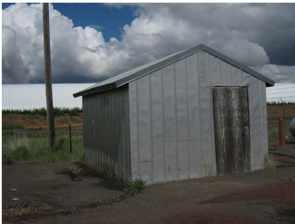
Buildings and Structures #5: Building 105-1, view to southeast (PWR Cultural Landscapes Program, 2015).
