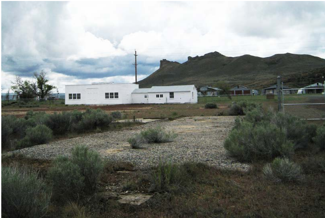
Circulation #3: Sidewalk of Administration, Building 72 at bottom of photo, looking south (PWR Cultural Landscapes Program, 2015).
