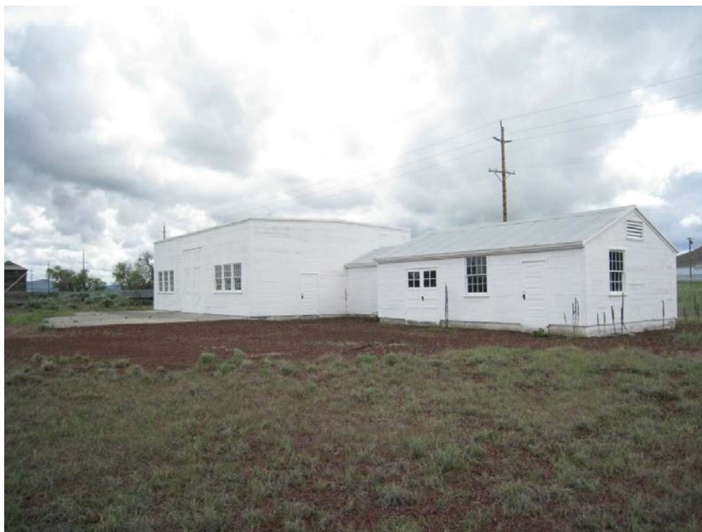
Buildings and Structures #6: Building 76, view to south (PWR Cultural Landscapes Program, 2015).
