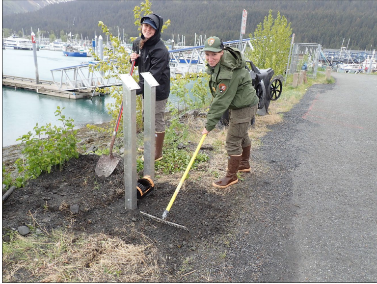
SCA intern and KEFJ biological science technician installing a boot brush at the north ramp at the Seward Harbor.
