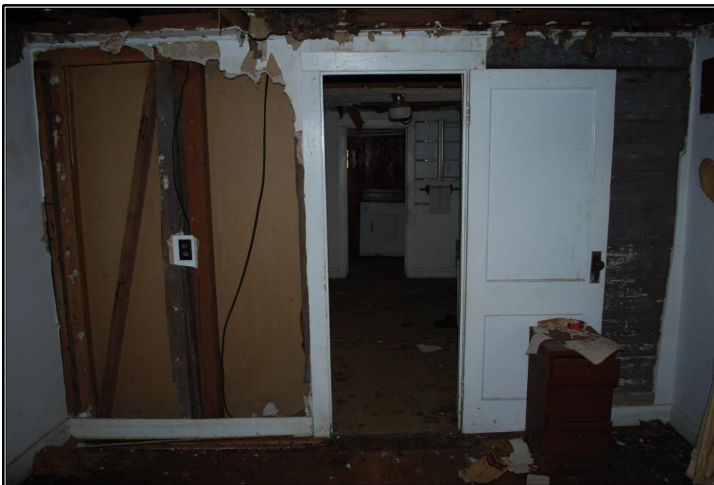
Figure 16. House interior: East original rear room looking north to portion of original plank wall covering (Room 103 on floor plan). Photograph taken October 29, 2019, by Trent Spurlock.
