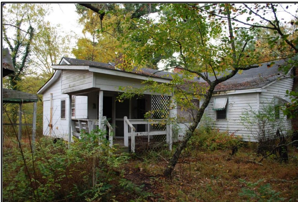
Figure 11. Rear (north) and west elevations of the dwelling showing the shed-roof rear porch, looking southeast. Photograph taken October 29, 2019, by Trent Spurlock.
