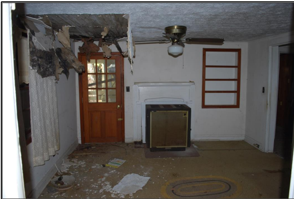
Figure 19. House interior: West room of gable-roof kitchen addition looking north to rear porch entry (Room 106 on floor plan). Photograph taken October 29, 2019, by Trent Spurlock.
