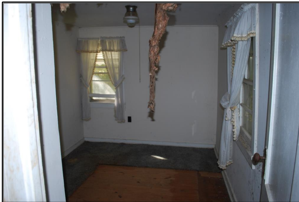
Figure 18. House interior: West original rear room looking west (Room 105 on floor plan). Photograph taken October 29, 2019, by Trent Spurlock.
