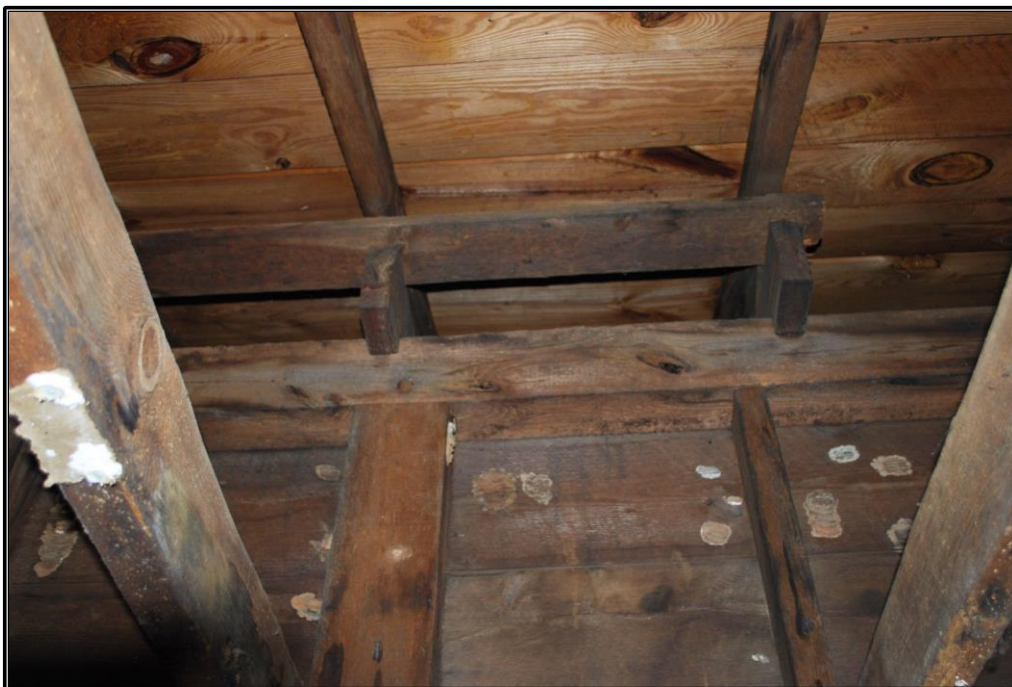
Figure 27. House interior: Mortise-and-tenon joint on top plate and continuous ledge looking from Room 103 towards Room 102. Photograph taken October 29, 2019, by Trent Spurlock.
