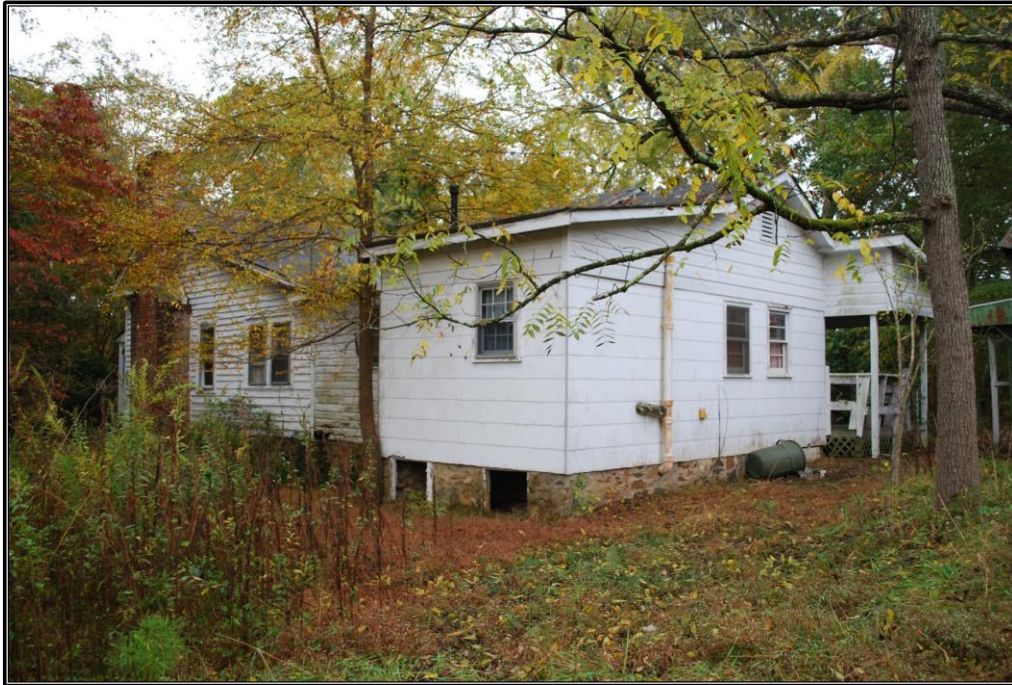
Figure 10. East and rear (north) elevations of the house showing the rear addition containing the bathroom and utility room, looking southwest. Photograph taken October 29, 2019, by Trent Spurlock.
