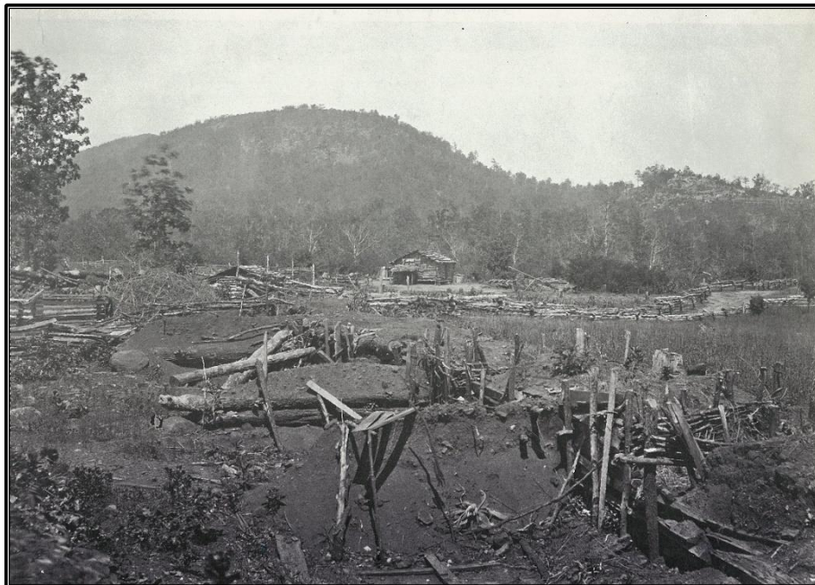
Figure 48. View of Kennesaw Mountain from the federal lines south of the Burnt Hickory and Marietta Roads near the Hardage house, looking northeast toward Kennesaw Mountain and Pigeon Hill. 115
