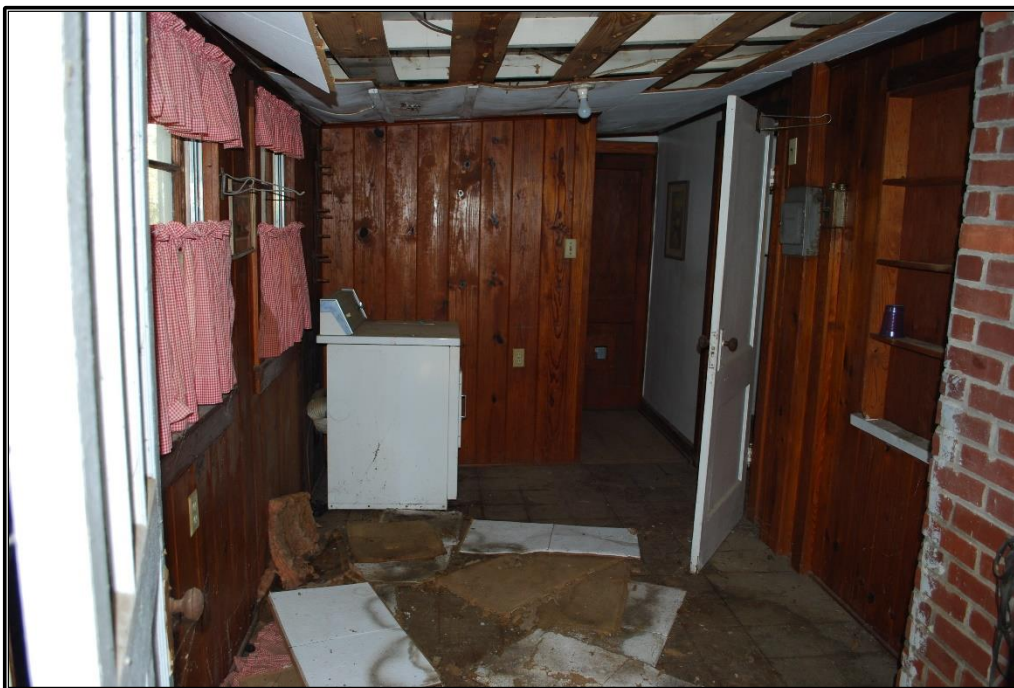
Figure 22. House interior: Utility room (Room 108 on floor plan) looking east to the bathroom. Photograph taken October 29, 2019, by Trent Spurlock.
