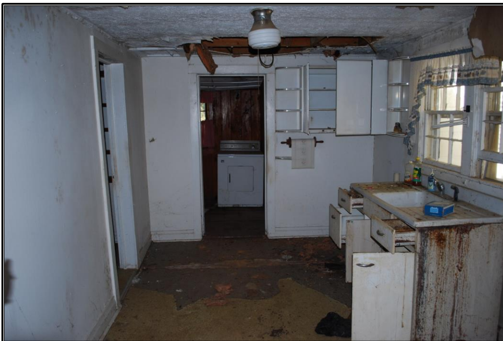
Figure 20. House interior: Kitchen (Room 107 on floor plan) looking north to utility room (Room 108). Photograph taken October 29, 2019, by Trent Spurlock.
