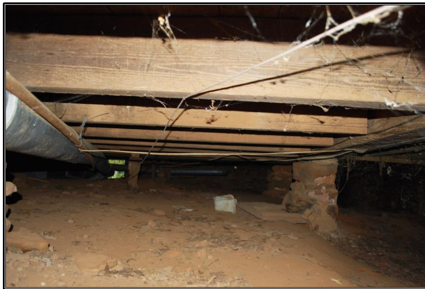
Figure 24. House crawlspace: Floor joists exhibiting sash sawn markings, stone support piers, and the front sill beam. Photograph taken October 29, 2019, by Trent Spurlock.
