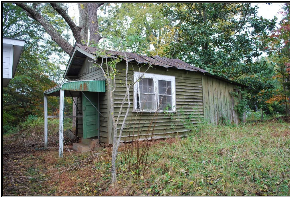
Figure 29. Smokehouse (Resource B): Façade (south) and east elevations. Photograph taken October 29, 2019, by Trent Spurlock.
