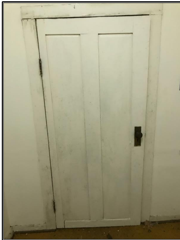
Figure 25. House interior: Two-panel, mortise-and-tenon door between Rooms 100 and 104. Photograph taken October 1, 2020, by Anthony Winegar.
