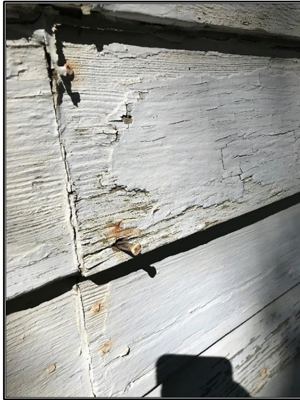
Figure 23. House exterior: Detail of weatherboard siding and cut nail on east side of house. Photograph taken October 1, 2020, by Anthony Winegar.
