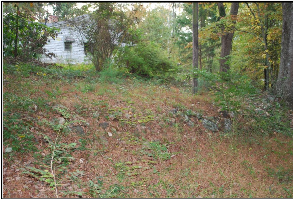
Figure 34. Stone Retaining Walls (Resource G), looking east-southeast along the driveway to the house. Photograph taken October 29, 2019, by Trent Spurlock.
