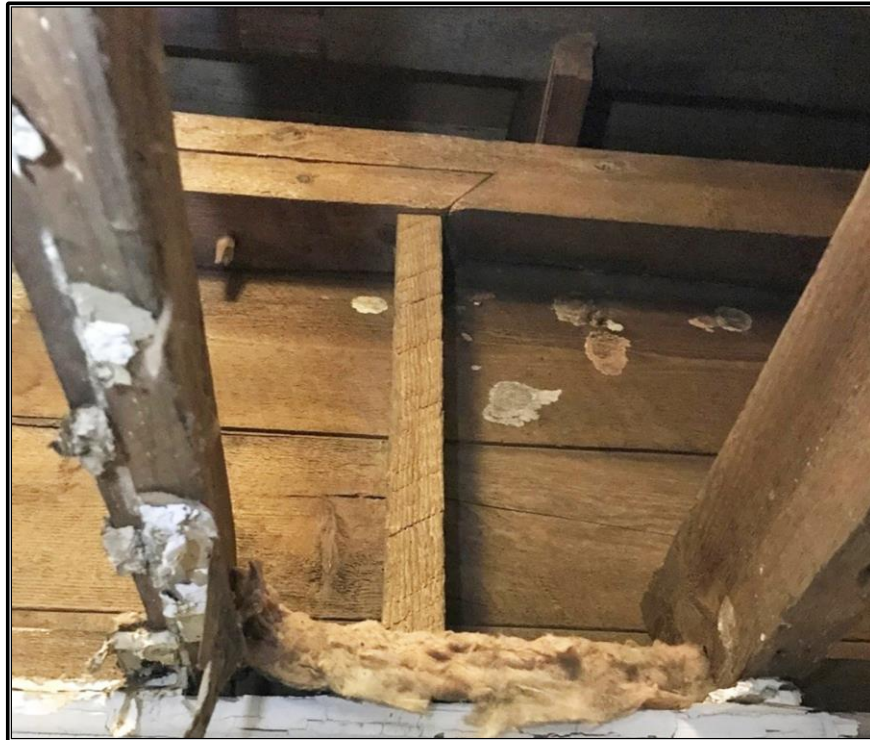
Figure 26. House interior: View of simple z-scarf joint with peg along the top plate. Photograph taken October 1, 2020, by Anthony Winegar.
