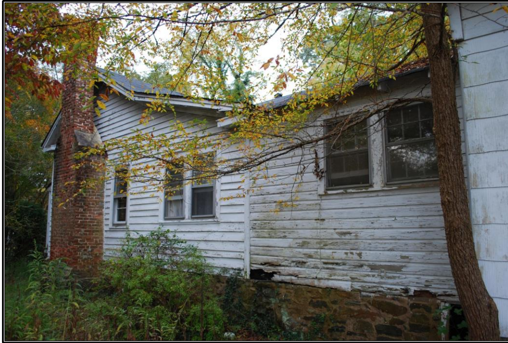
Figure 9. East elevation of the residence, looking southwest at original portion and gable-roof addition at rear of original block of house. Photograph taken October 29, 2019, by Trent Spurlock.
