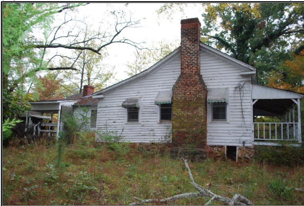
Figure 8. West elevation of the residence, looking east. Photograph taken October 29, 2019, by Trent Spurlock.
