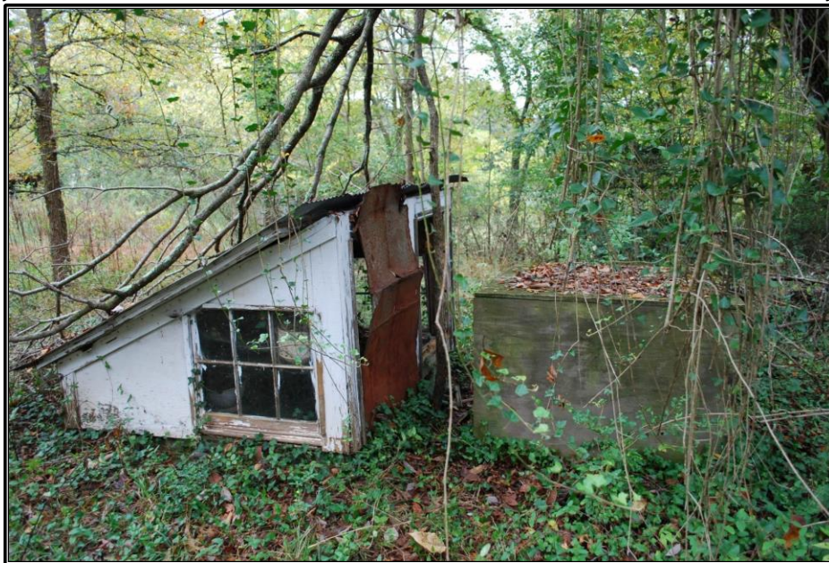
Figure 33. Original well and well (Resources F and E): West and south elevations. Photograph taken October 29, 2019, by Trent Spurlock.
