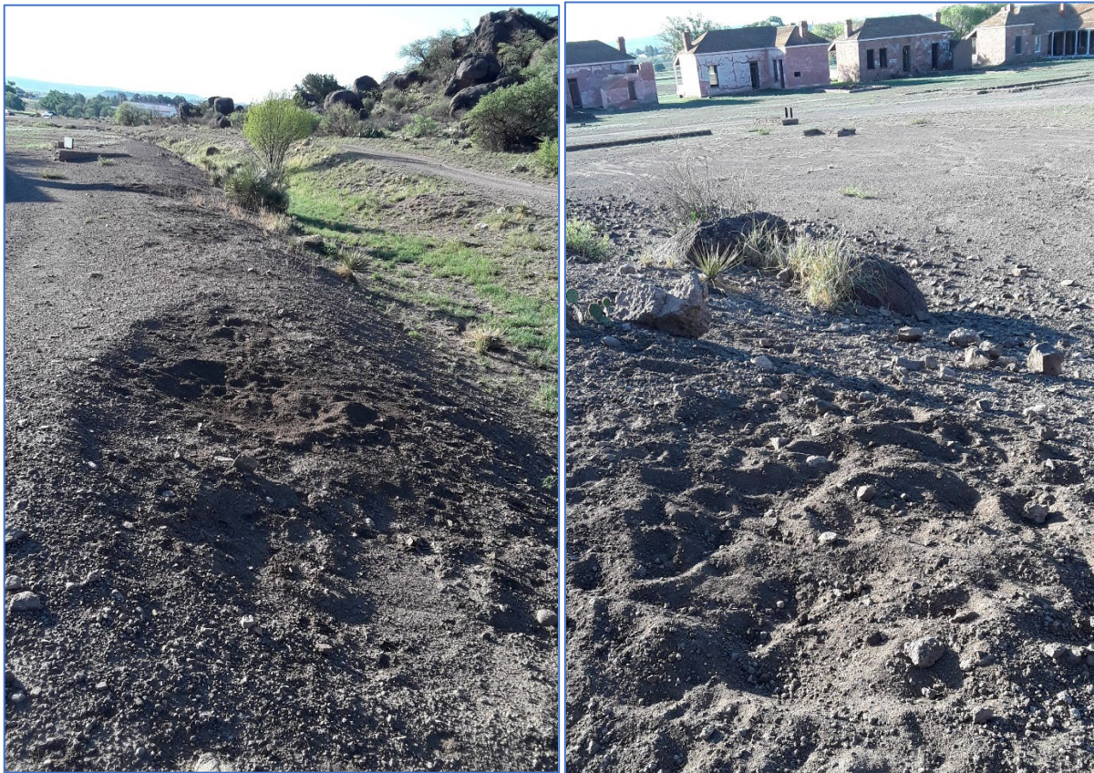
Figure 4: Aoudad pits in historic water diversion earthworks
