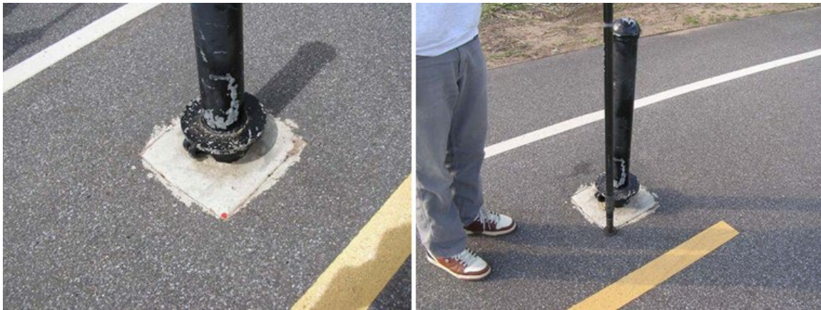
Figure S3.3. Monument located at corner of cement slab on the bike path at Fort Wadsworth, Gateway National Recreation Area; adequate space to site a GPS/GNSS rover receiver pole (Staten Island, New York, April 2009).
