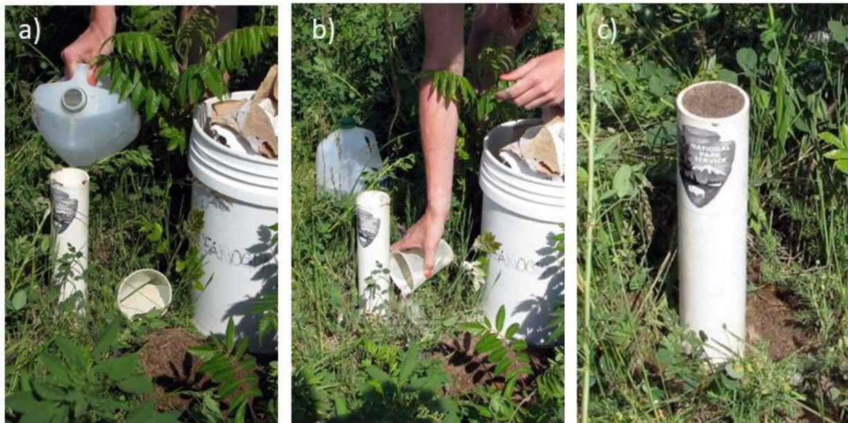
Figure S3.6. Installation of the PVC pipe monument, a) and b) inserting the cement, water, and sand into and around the pipe, and c) National Park Service logo on PVC pipe.
