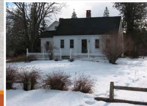
609 Cranberry Road (Espinoza/Bancroft House) (Photo by Grulich 2014)
