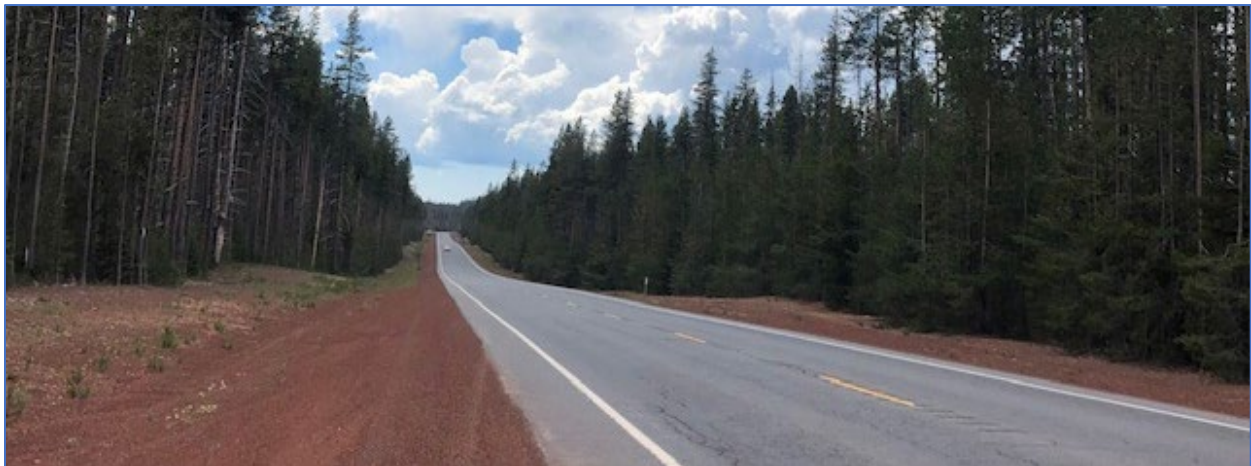
Figure 19. Highway 138 after being recently graded showing very few plants growing on the roadside. Photo by Alexandra von Bergman.
