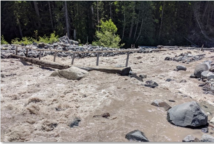
Figure 1. A foot log on the Wonderland Trail crossing the Nisqually River in Mount Rainier National Park, is damaged by high water during the heat event. NPS Photo.
