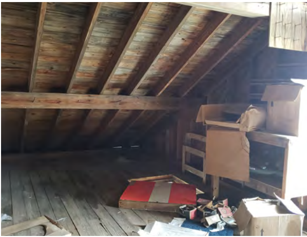
Figure 2.140. Attic - View looking southeast.
