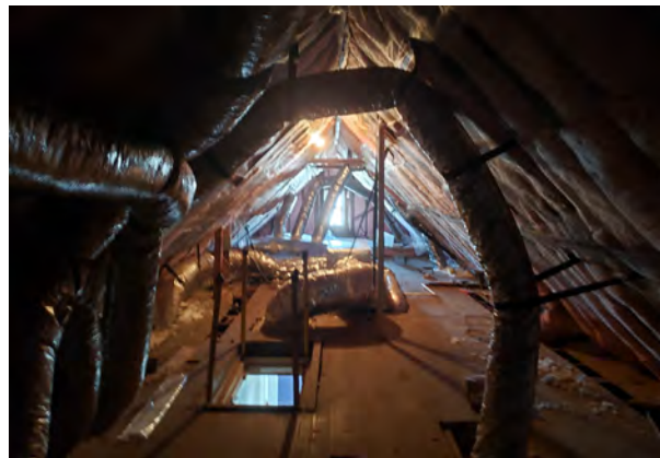
Figure 2.110. Overview of attic looking east toward original gable end.
