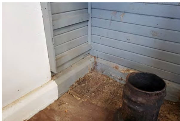
Figure 2.133. Original concrete curb and wall cladding in Room 103.
