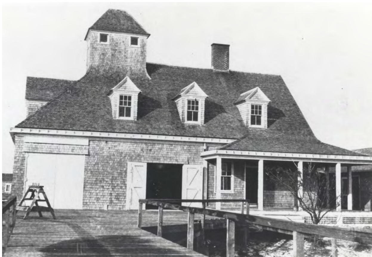
Figure 2.8. Early photo of the south elevation thought to reflect original 1908 condition. (NPS ID: 3338 SRI new USLSS restricted-jpg634023527350000000, provided March 2020 by previous contracting officer's representative (COR))
