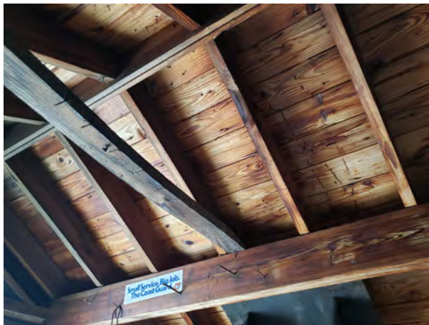
Figure 2.152. Ridge pole at north and south ends of the attic.
