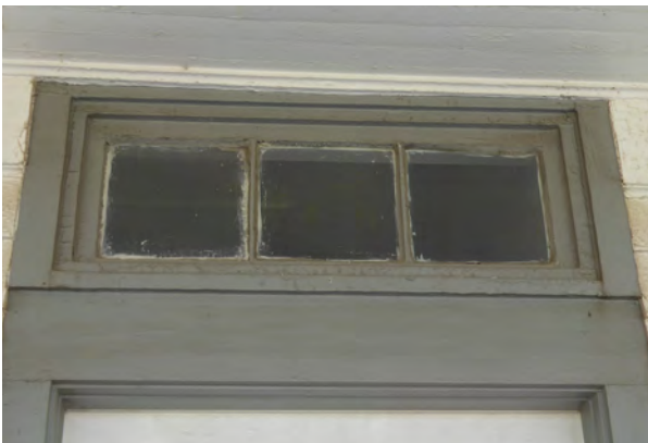
Figure 2.19. Original transom sash at north doorway.
