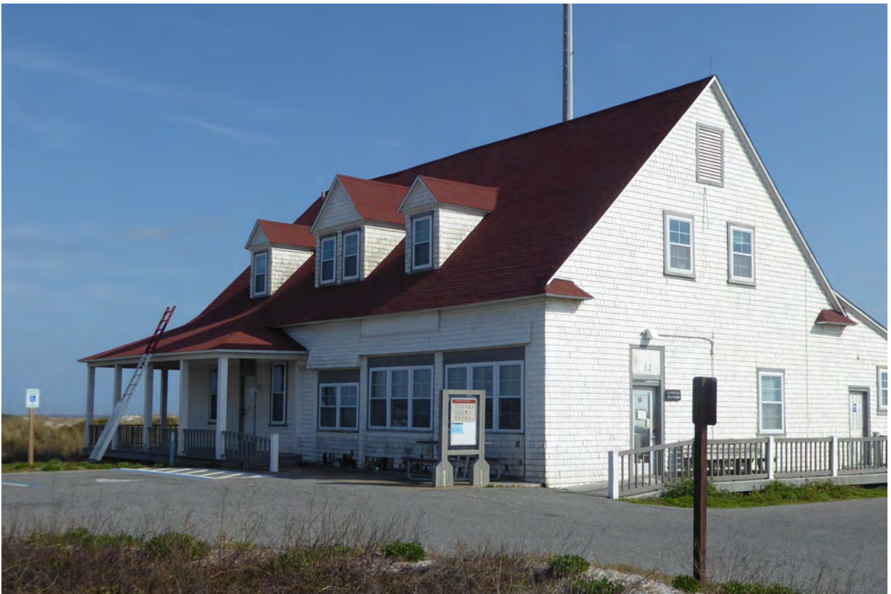
Figure 2.7. Oblique view of the station from the northwest. Note modern deck at right.
