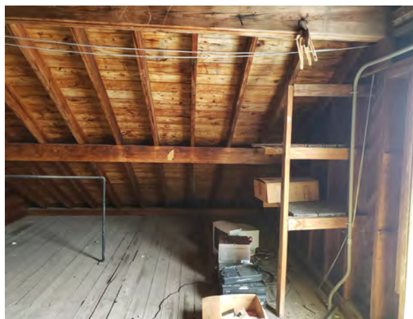
Figure 2.153. Roof framing at ends of attic. Note pair of beams supporting the rafters.
