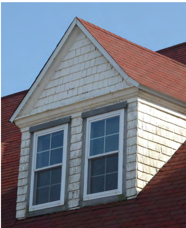
Figure 2.29. Typical large dormer added in 1937.
