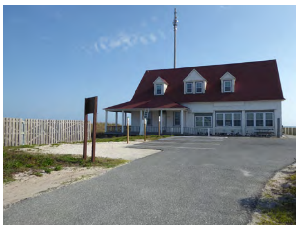
Figure 2.3. Parking area north of the station.
