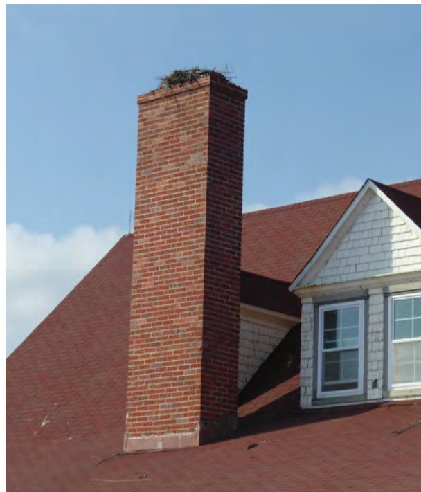
Figure 2.31. Brick chimney on south elevation.
