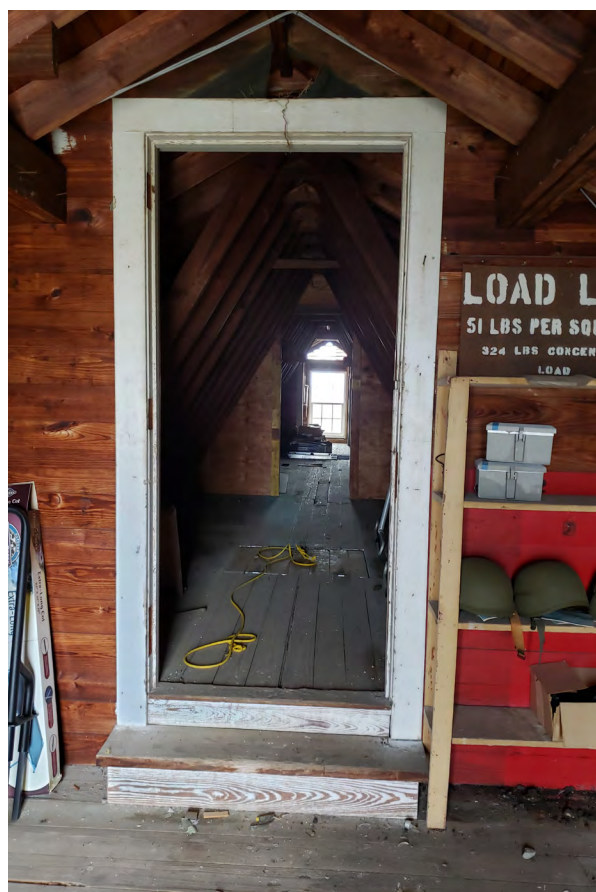
Figure 2.147. Typical doorway and casing in attic.
