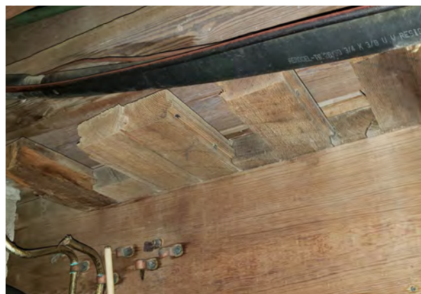
Figure 2.73. Ends of early floorboards beneath Room 101C as seen in the crawlspace.
