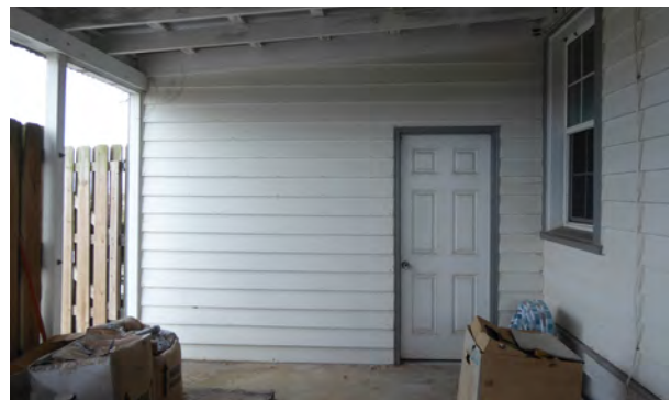
Figure 2.122. Garage - Fenced area at north elevation looking east.
