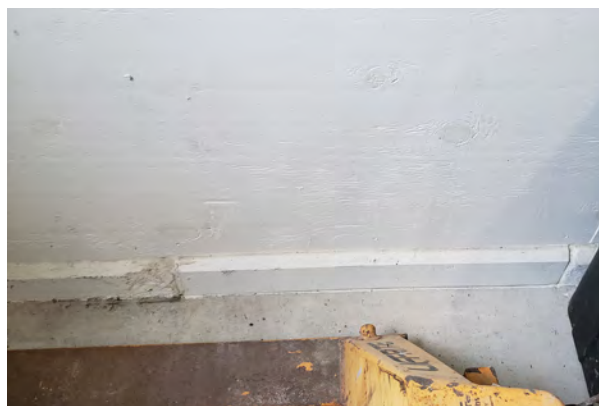
Figure 2.134. Example of wood patch in concrete curb at original interior doorway location in Room 102.
