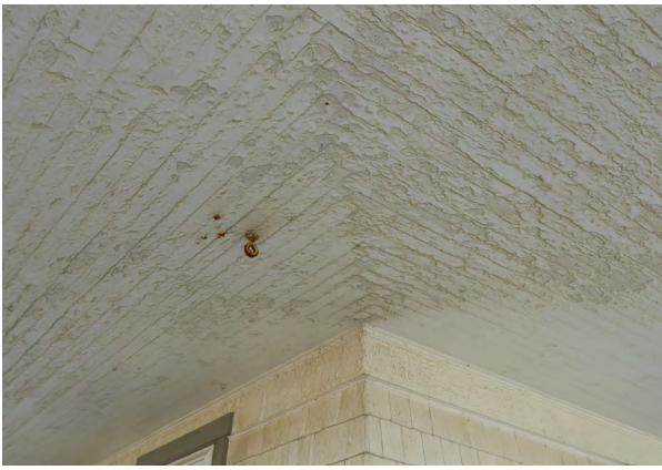
Figure 2.26. Original beaded-board porch ceiling.
