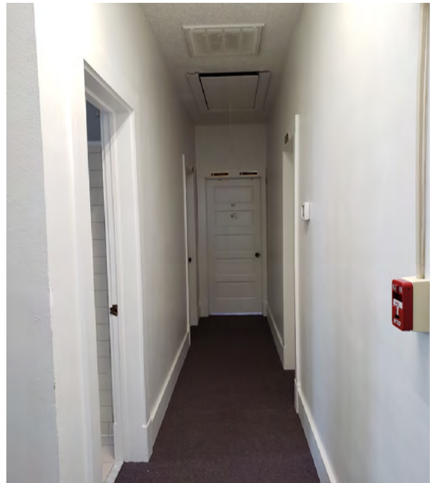
Figure 2.90. Room 203 - View looking west.
