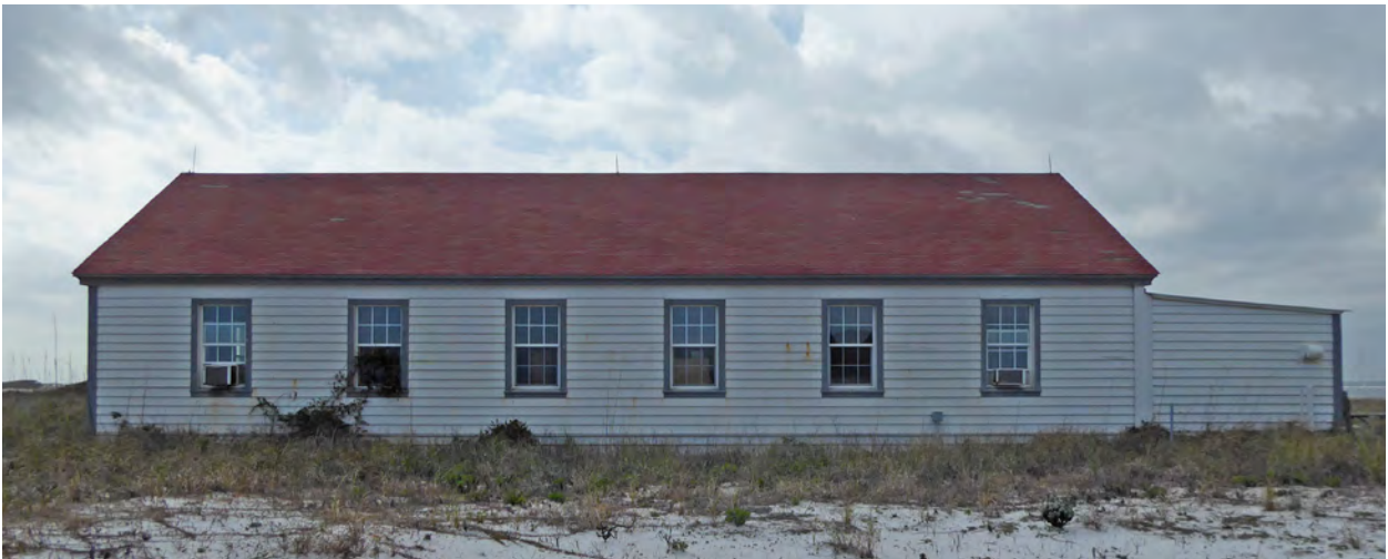
Figure 2.119. Garage - East elevation.
