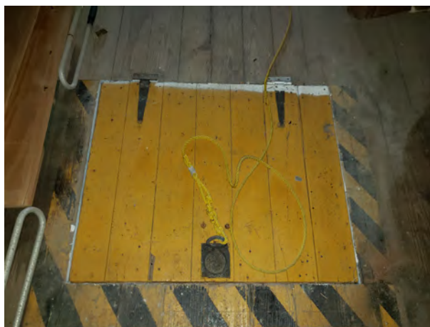
Figure 2.146. Early hatch door in floor of center portion of the attic.
