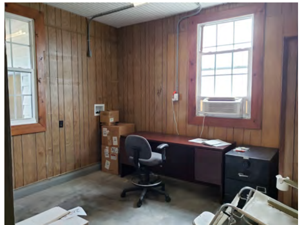
Figure 2.128. Room 101B - View looking northeast.
