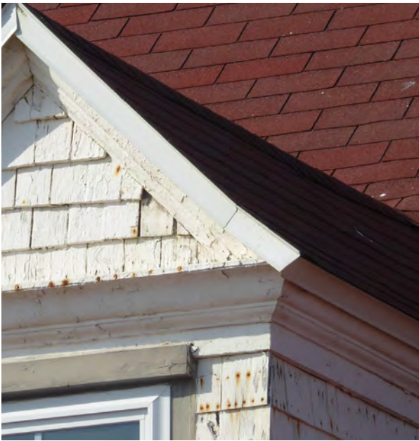
Figure 2.18. Detail of original cornice molding at dormer.
