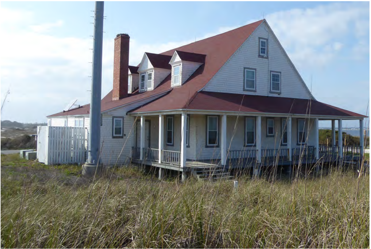
Figure 2.6. Oblique view of the station from the southeast. Note original wrapping open porch and the 1937 shed roofed-addition at left.
