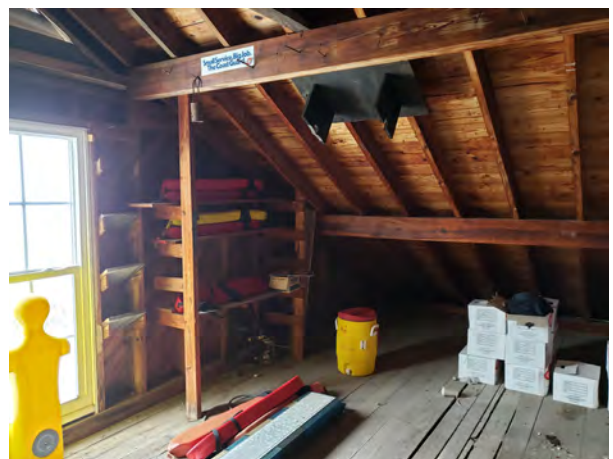
Figure 2.145. Attic - View looking northeast.
