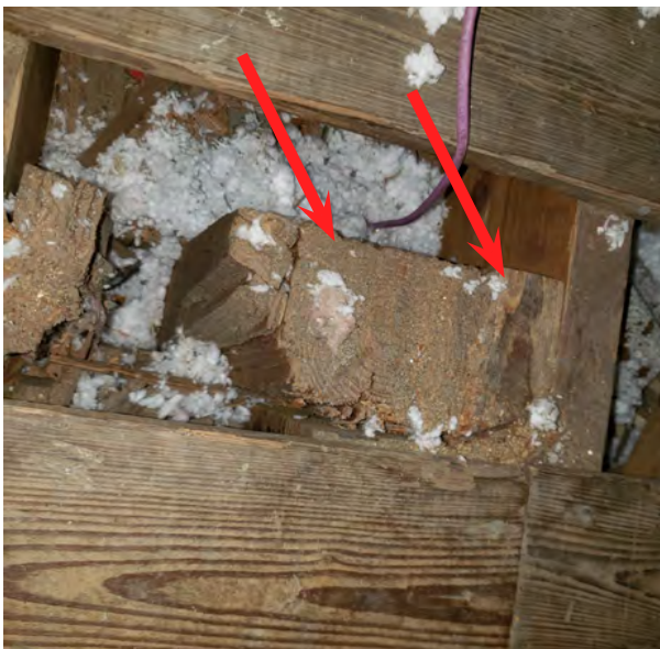
Figure 2.109. Original corner post of lookout as viewed in attic.
