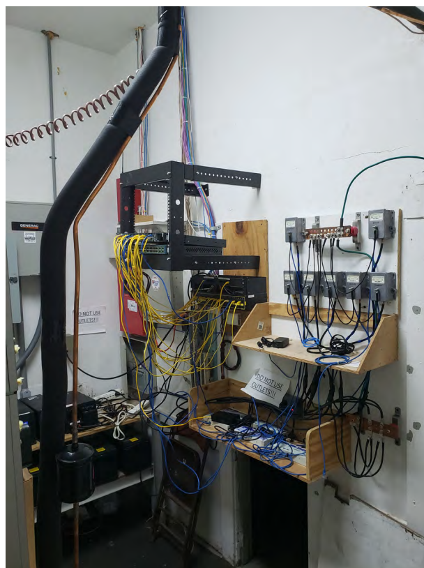
Figure 2.66. Room 109 - View looking southeast.
