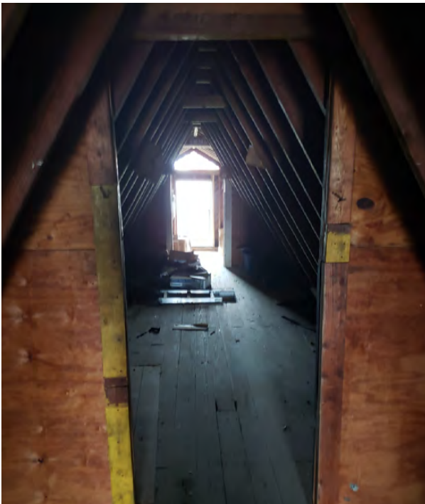
Figure 2.142. Attic - Center portion looking south.
