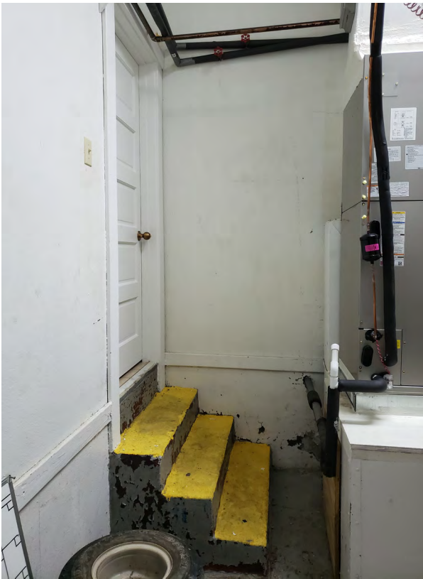
Figure 2.67. Room 109 - View looking northwest.
