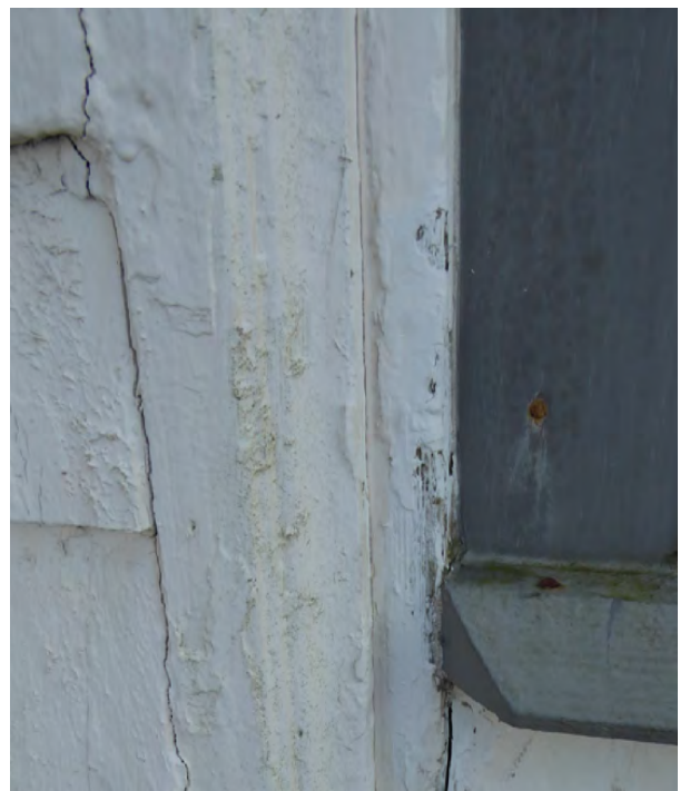
Figure 2.21. Detail of typical original exterior casing at boat doorways.
