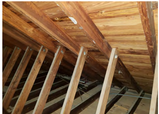
Figure 2.150. Diagonals at the midspan of the rafters of the center portion. Note exposed floor joists and topside of plywood ceiling of Room 102.
