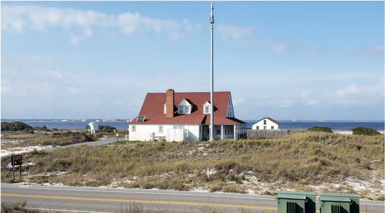
Figure 2.1. The 1908 Santa Rosa Life-Saving Station as viewed from the southeast, across Fort Pickens Road. The 1939 Coast Guard Garage is visible to the right of the station building. Unless otherwise noted, all photos in this section were taken by JKOA in 2020.
