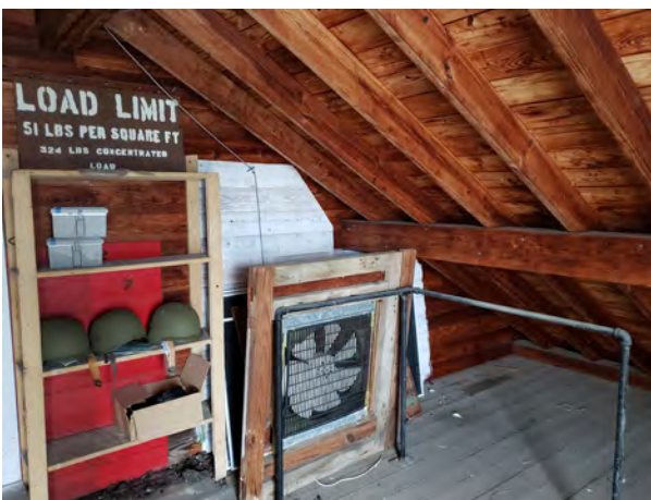
Figure 2.144. Attic - View looking southwest.
