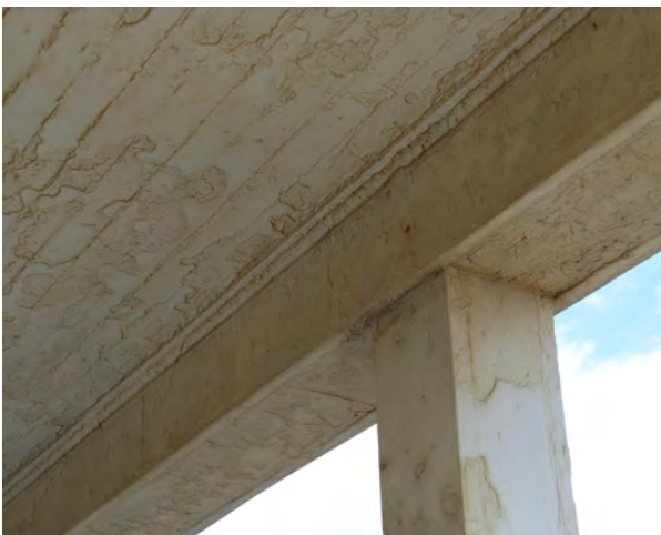
Figure 2.27. Original porch beam, trim, and post wrapping.
