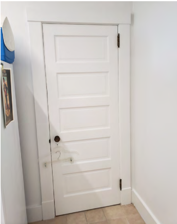
Figure 2.75. Example of typical 1937 five-horizontal-panel interior door in Room 105.
