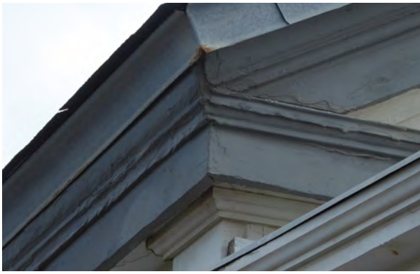
Figure 2.123. Early cornice molding and fascia as seen at northwest corner.
