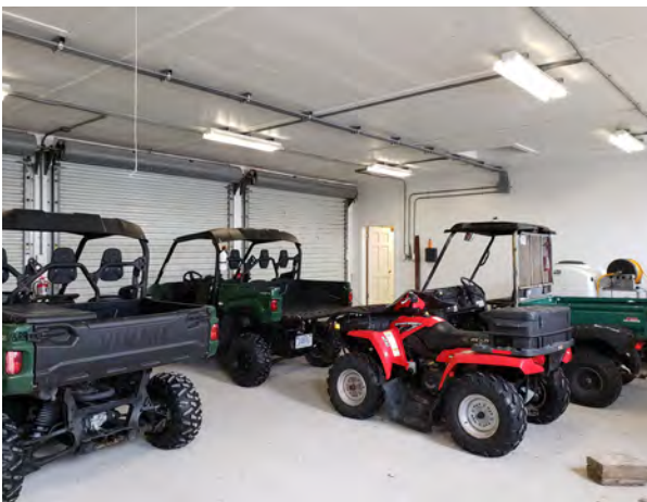
Figure 2.129. Room 102 - View looking southwest.
