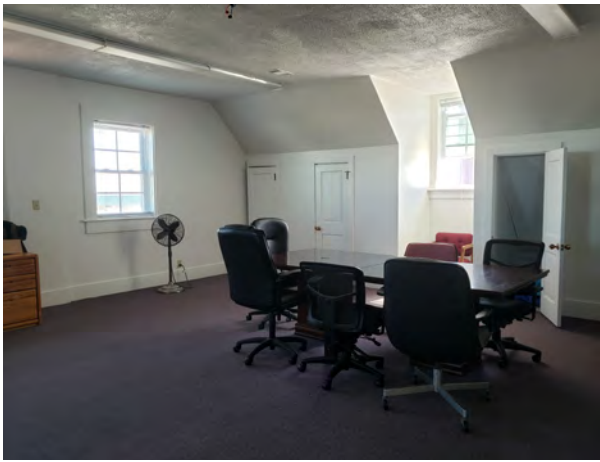
Figure 2.93. Room 205 - View looking southeast.
