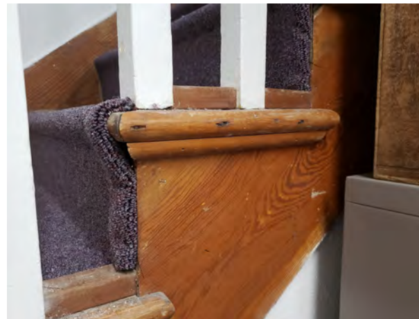
Figure 2.81. Detail of stair treads and nosings.
