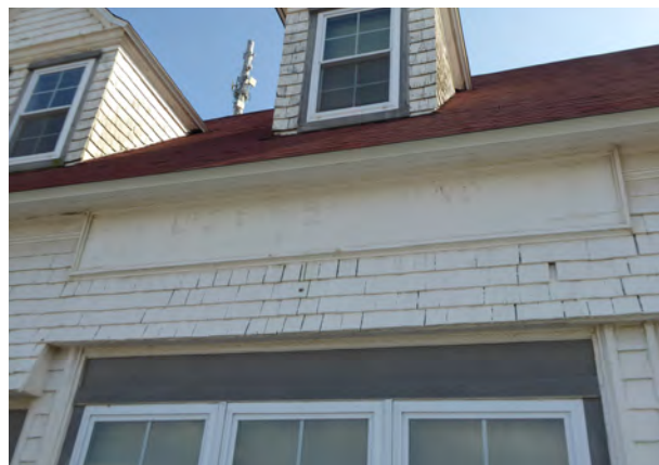
Figure 2.32. Early or original sign board on north elevation.
