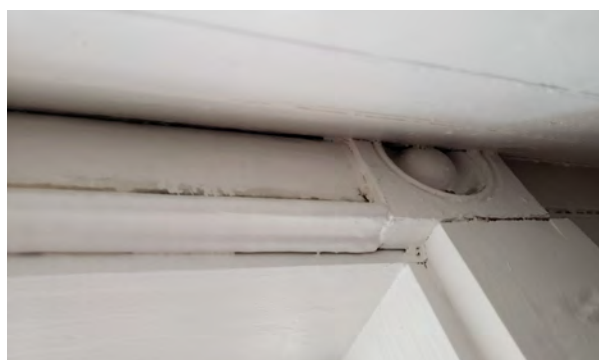
Figure 2.104. Partial original trim in southeast closet of Room 105.
