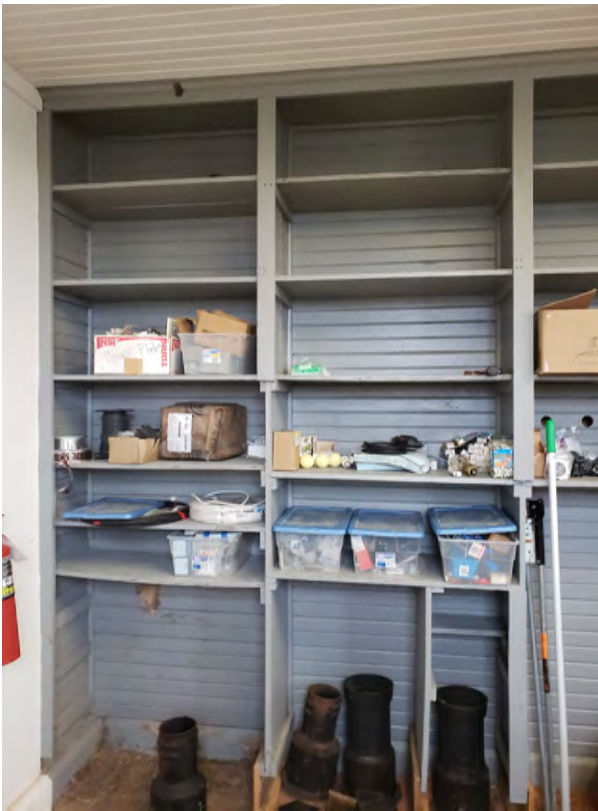
Figure 2.135. Original horizontal V-groove boards at rear of casework in Room 103.
