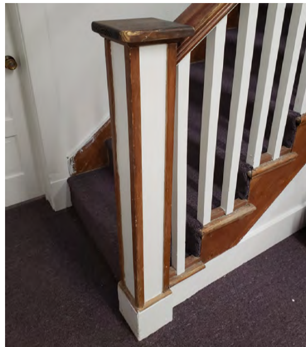
Figure 2.80. Newel post at base of stair. Newel at top of stair is similar.
