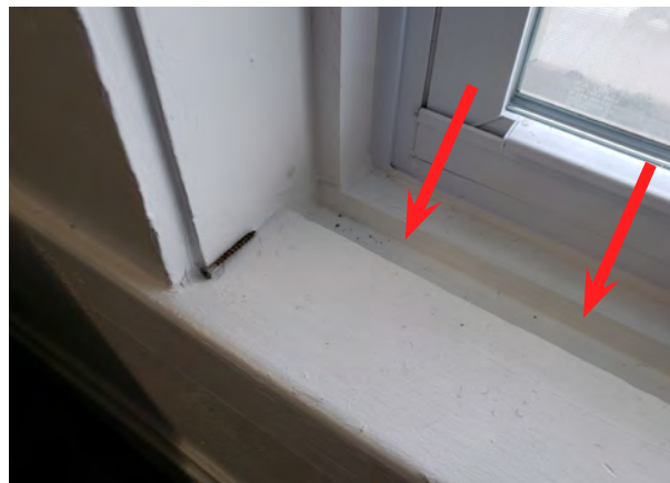
Figure 2.25. Interior view of typical window opening at sill. Note channel where wood sash would have been located. Stops have been added at the new vinyl window.
