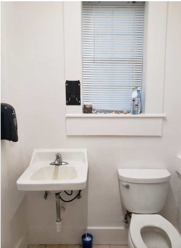
Figure 2.59. Room 106 - View looking east.
