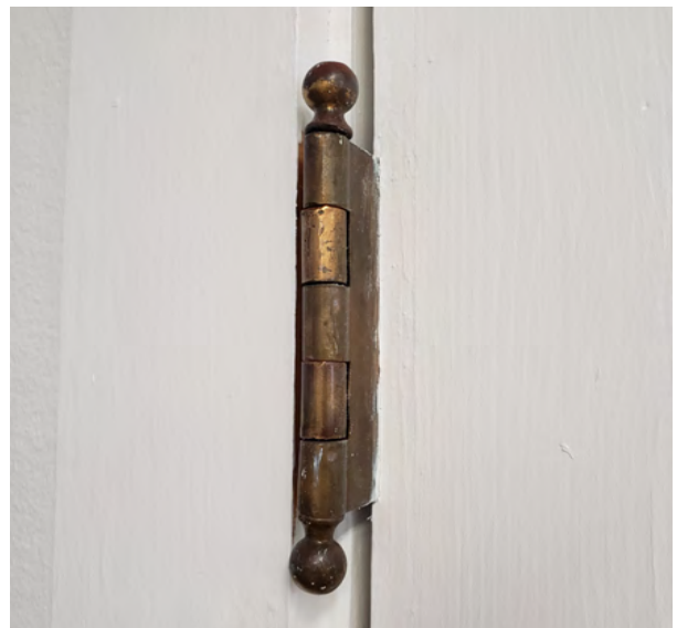
Figure 2.76. Example of typical 1937 ball-pin hinge.
