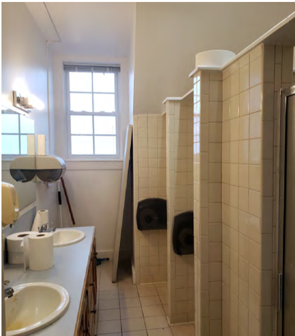
Figure 2.97. Room 206 - View looking south.
