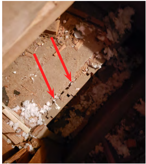
Figure 2.100. Early vertical wall cladding boards on south wall of Room 204 as viewed from attic.
