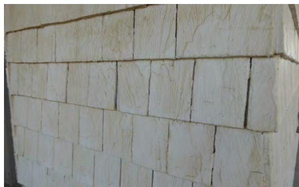
Figure 2.17. Example of early wood shingle siding beneath porch roof.
