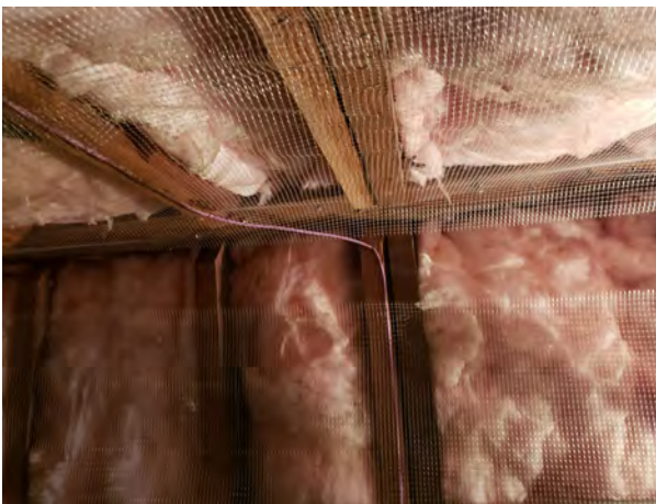
Figure 2.113. Transition point between 1908 and 1937 ridge pole and rafters.
