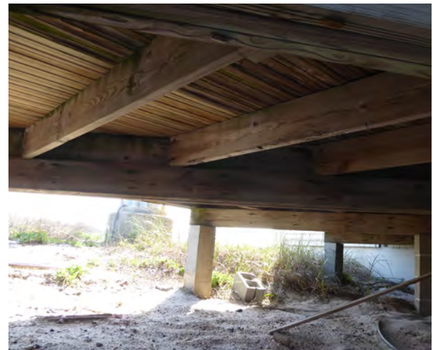
Figure 2.107. Typical porch floor framing.
