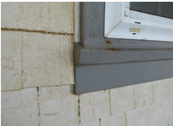
Figure 2.23. Detail of early or original exterior window sill below porch roof.
