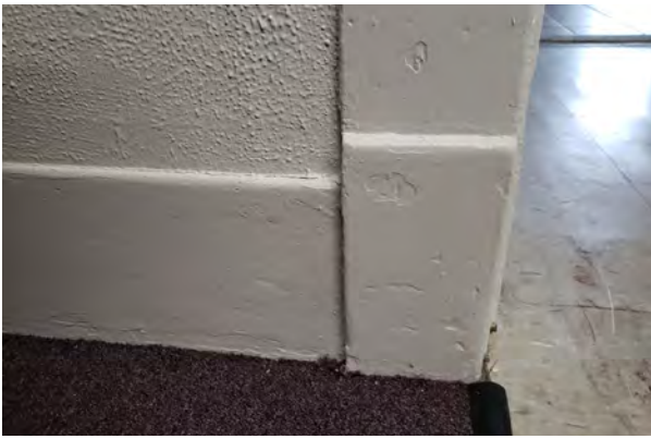
Figure 2.74. Example of typical 1937 plinth block and baseboard.
