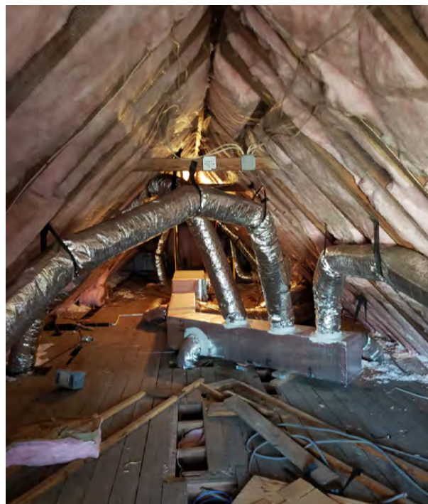
Figure 2.111. Overview of attic looking west toward 1937 gable end.
