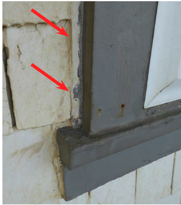
Figure 2.24. Detail of sill and overlay window casing. Note early casing flush with wood shingles at left.
