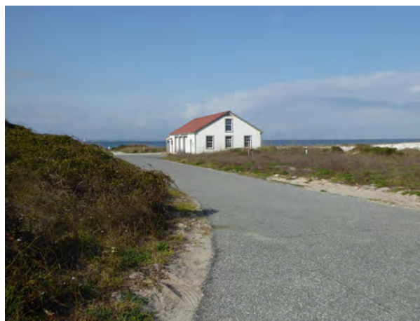
Figure 2.4. View north from the rear of the station toward the 1939 garage.
