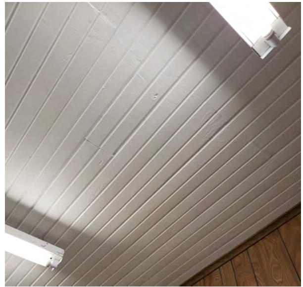
Figure 2.137. Original v-groove ceiling in Room 101A. The same ceiling is in Room 101B.
