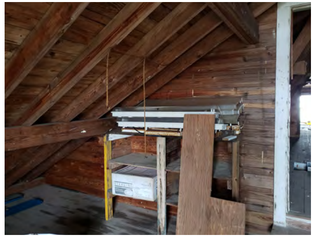
Figure 2.141. Attic - South portion looking northwest.
