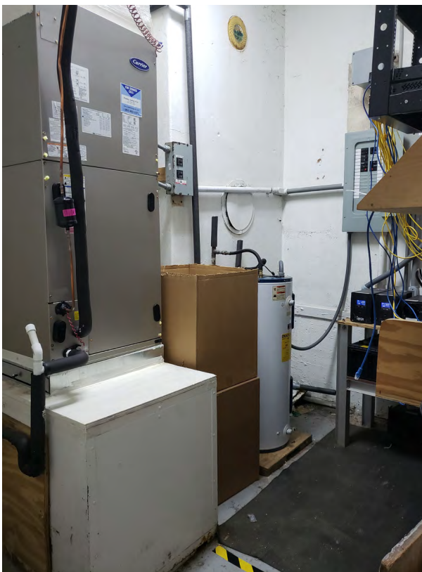
Figure 2.65. Room 109 - View looking northeast.
