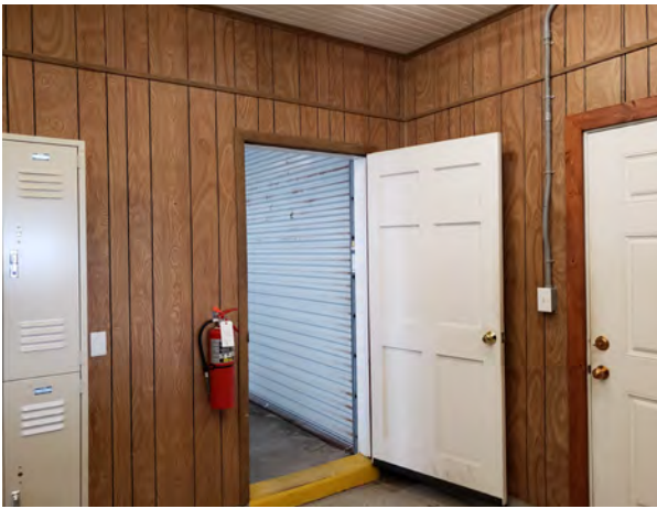
Figure 2.125. Room 101A - View looking southwest.
