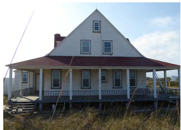
Figure 2.11. Present-day east elevation.
