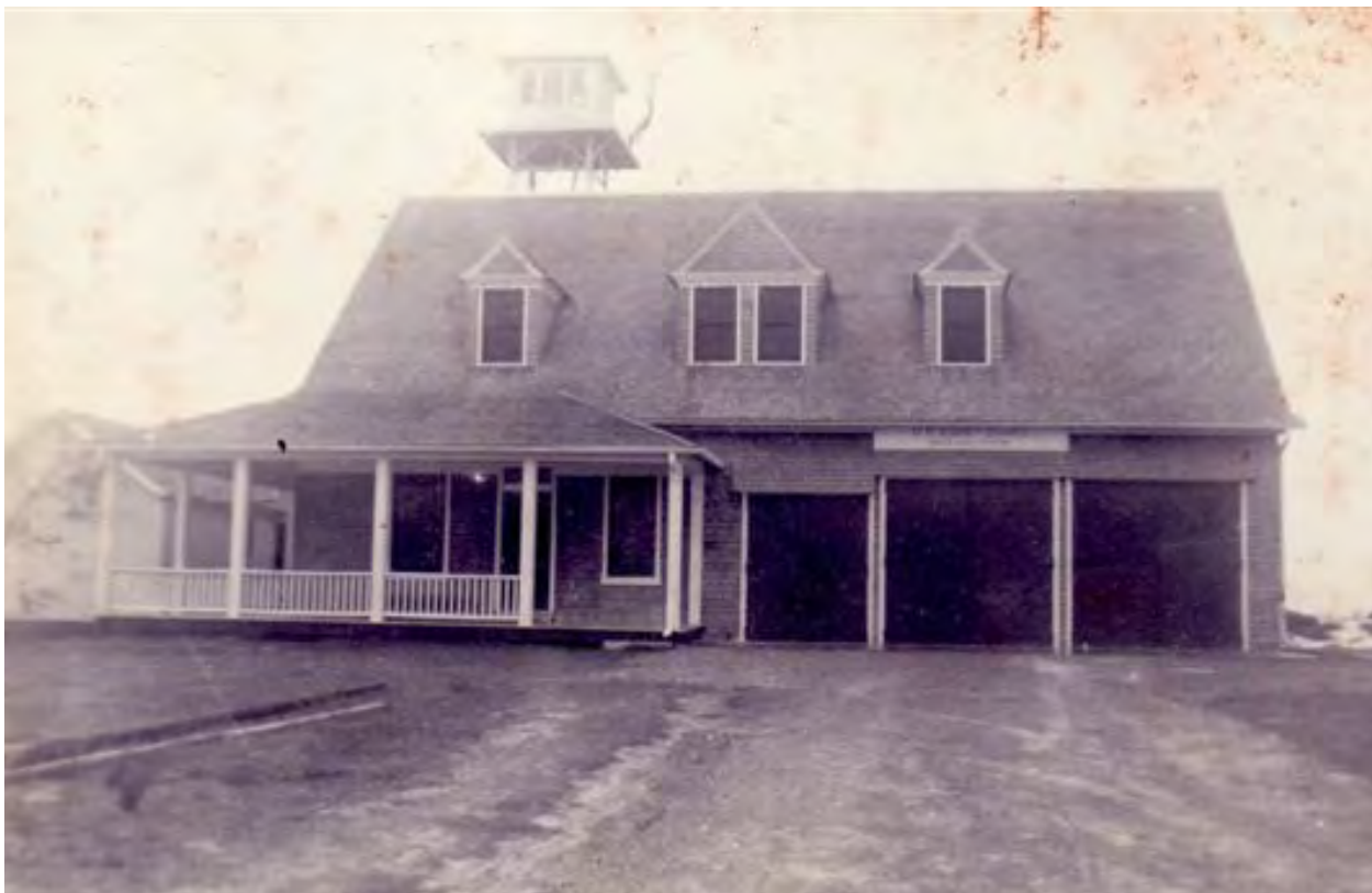
Figure 2.13. Historical photo showing the north elevation after 1937 modifications . Note new freestanding lookout tower behind the building.(NPS ID not given, provided March 2020 by previous contracting officer's representative (COR)).
