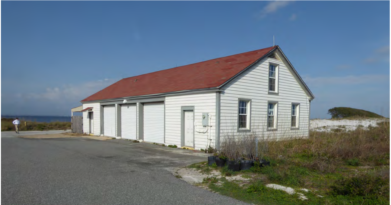
Figure 2.116. The 1939 Coast Guard Garage as viewed from the northwest. Unless otherwise noted, all photos in this section were taken by JKOA in 2020.
