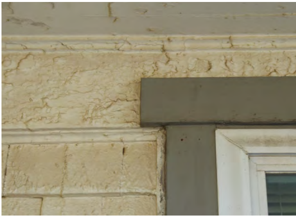
Figure 2.22. Original frieze board and trim below porch roof. Note added window lintel and casing.
