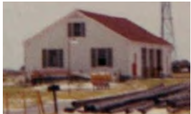
Figure 2.121. Garage - North elevation prior to addition. Low photo quality due to structure not being the focus of the original photo. (NPS ID not given, provided March 2020 by previous contracting officer's representative (COR)).
