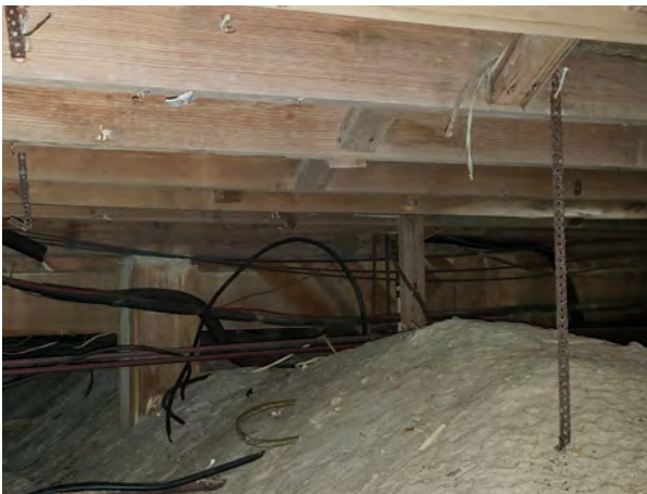
Figure 2.106. View looking east in crawlspace. Note drop in framing height in background corresponding with transition to boat room level.
