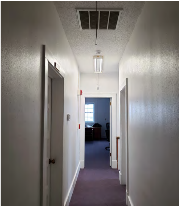
Figure 2.89. Room 203 - View looking east.
