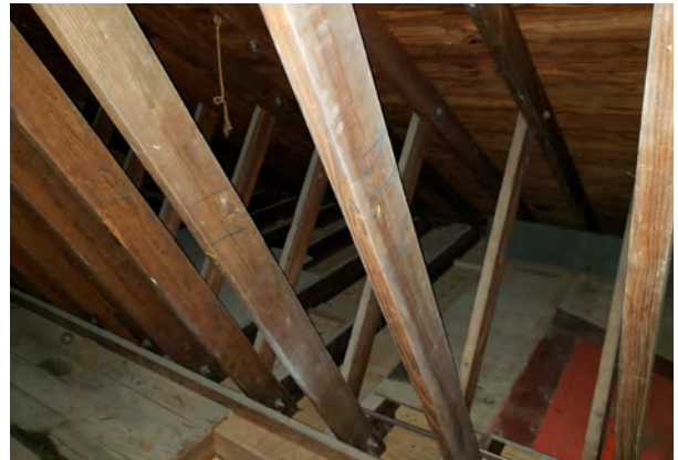
Figure 2.149. Diagonal members at center section. Members in foreground form A-frame of truss.
