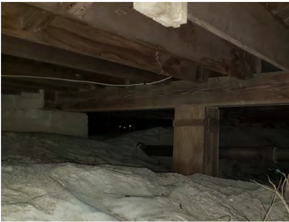
Figure 2.105. View of crawlspace beneath east portion of the building. Original chimney base visible at left. Major east-west beam lies in-line with chimney and rests on concrete piers. Note that wood forms remain on many piers in the crawlspace.
