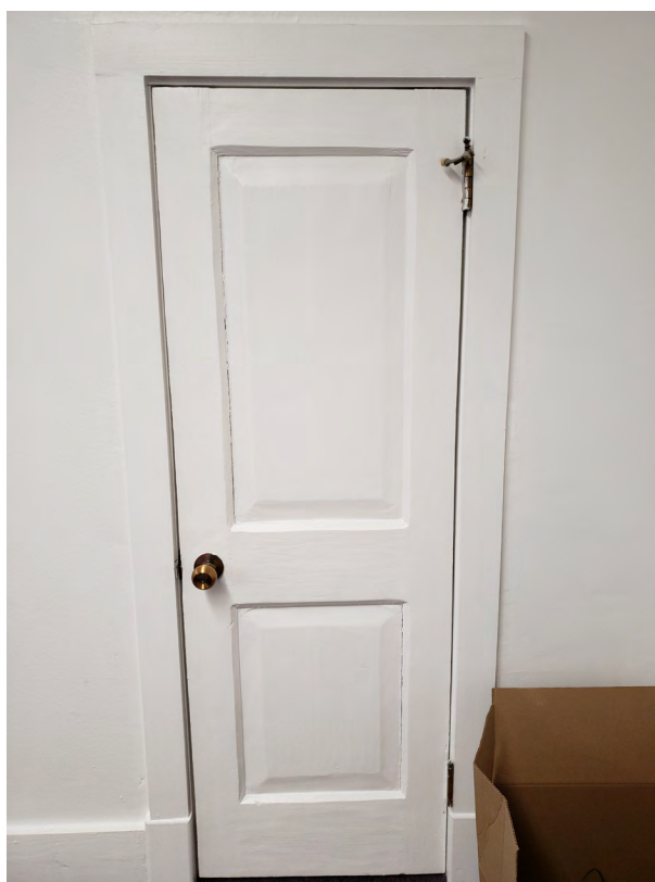
Figure 2.102. Original two-panel doors in Room 205.
