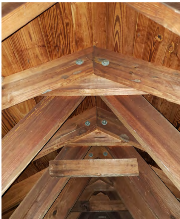
Figure 2.151. View of ridge and collar ties at center portion.
