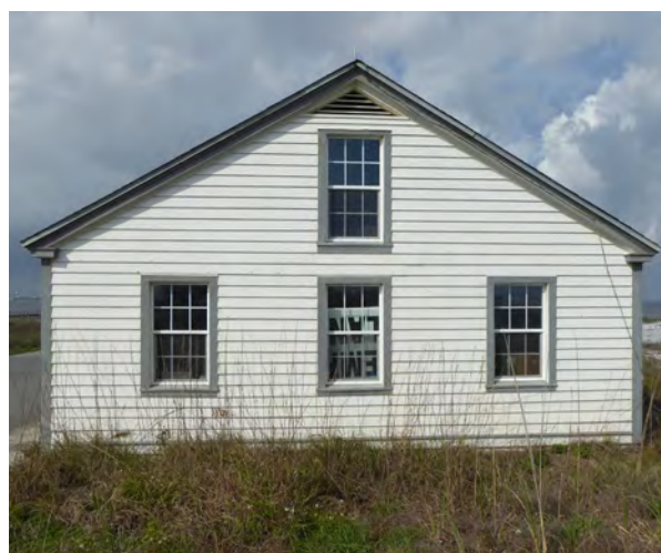
Figure 2.118. Garage - South elevation.
