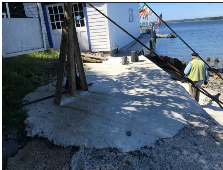
Figure 2 - Bear Island Boat House showing Structure, Fixed Dock, and Floating Dock
